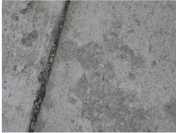
Figure 10. Salt scaled concrete sidewalk
