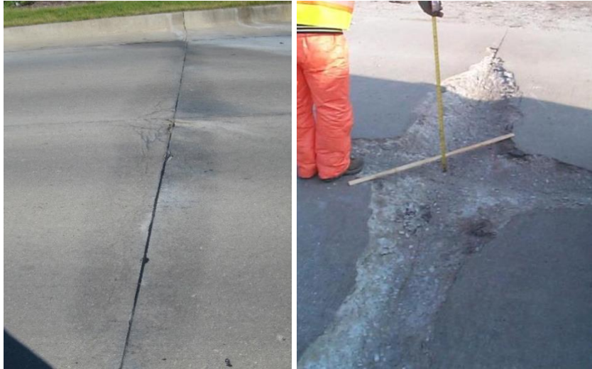
Figure 69. Deteriorated joint in concrete pavement
