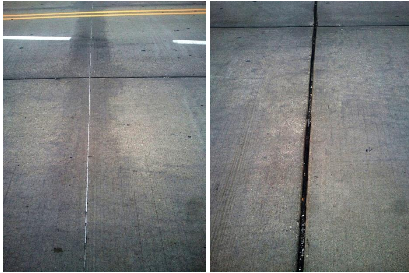
Figure 77. Comparison performance of sawn joint and formed joint
