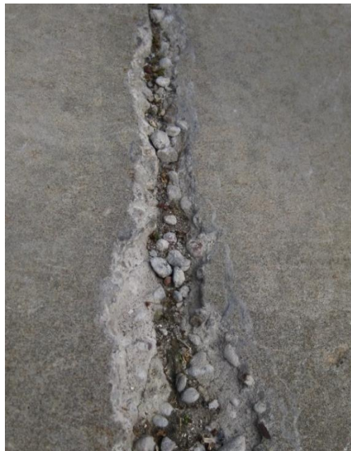
Figure 41. Field observation of joint deterioration
