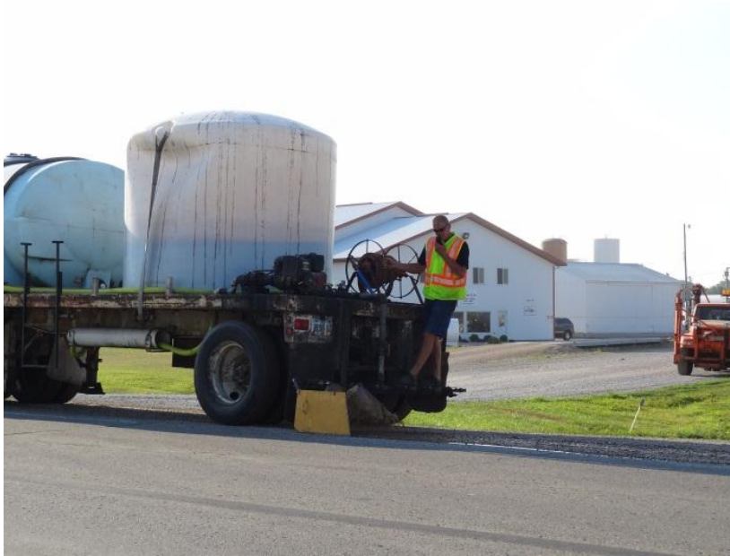
Figure 8. Soapstock application process
