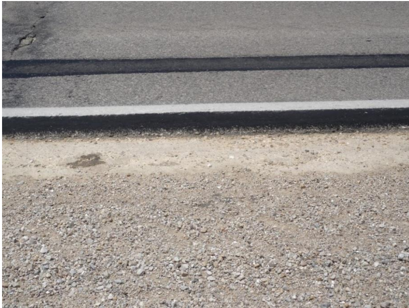
Figure 28. Shoulder of US 18 on eastbound near east of West Union
