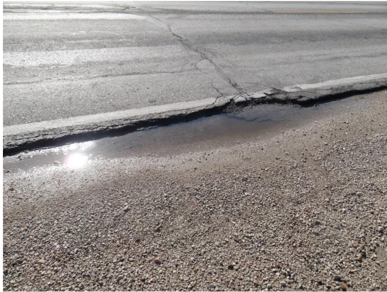
Figure 22. Edge rut developed around south of Algona
