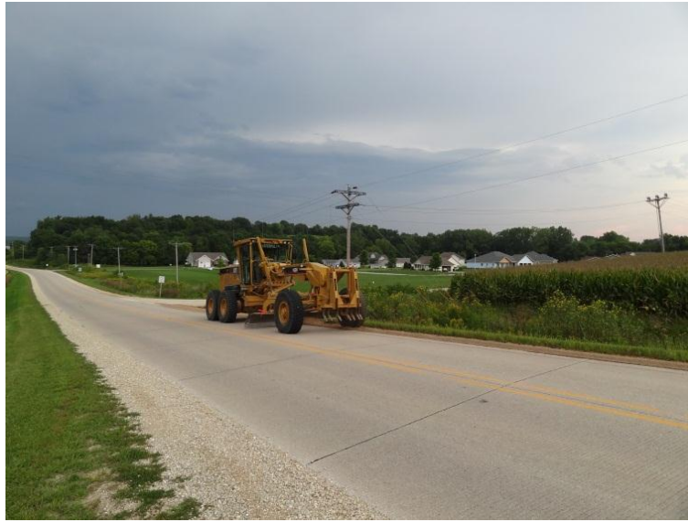
Figure 18. Grader bladed over the shoulder applied with sand
