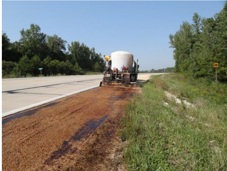
Figure 15. 12-ft wide soapstock applied on the shoulder of IA 13 near east of Elkader
