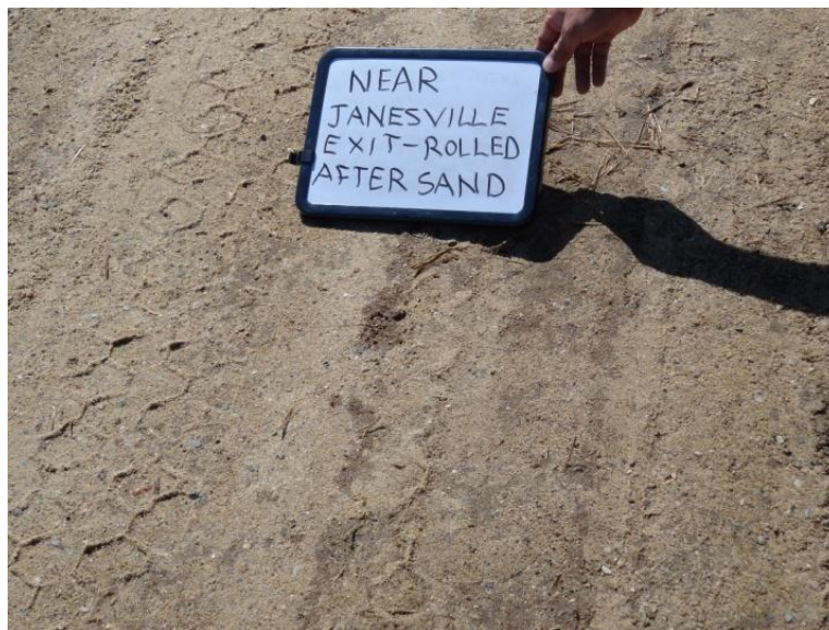
Figure 14. Surface rolled after sand application for the shoulder of US 63 near Denver
