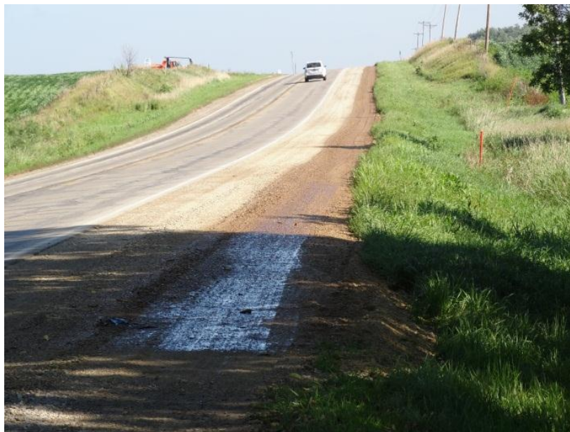
Figure 8. Soapstock application process
