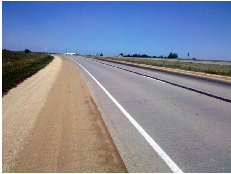
Figure 13. Soapstock and sand applied on the shoulder of US 63 near Denver
