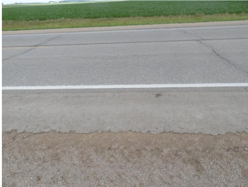
Figure 21. Eastbound shoulder of US 18 near Garner
