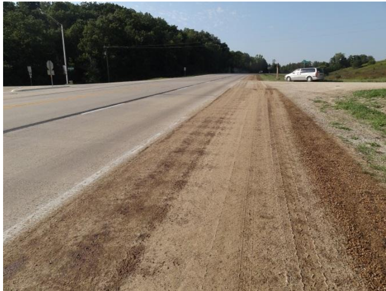
Figure 15. 12-ft wide soapstock applied on the shoulder of IA 13 near east of Elkader
