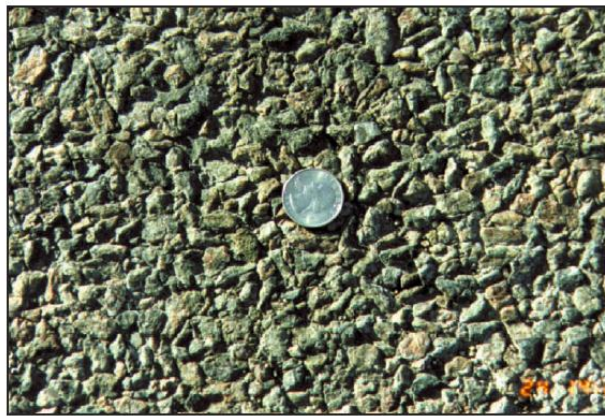
Figure 12: One-sized Chip Seal Application (Wood et. al. 2006)
