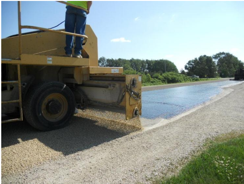
Figure 5: Chip Seal Application (photo taken by author)
