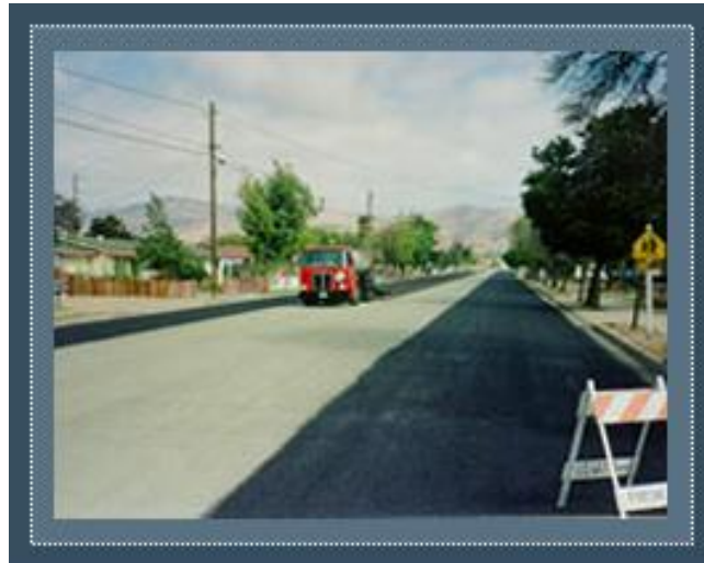
Figure 37: Road Fog Seal (NHI PPTCG 2007)
