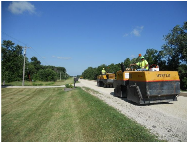
Figure 27: Three Rollers in Chip Seal Operation (photo taken by author)
