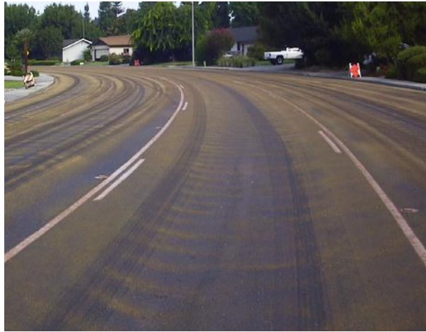
Figure 39: Fog Seal with Sand (Brownridge and Fox 2011)
