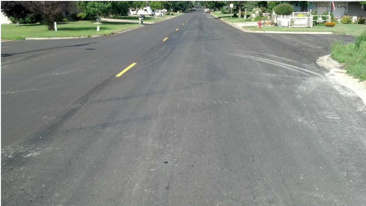
Figure 41: Picture of CSAH 10 near the urban designation-Picture taken 8/15/13 by Francis Dayamba
