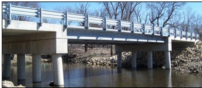
Figure 2-7: Jakway Park Bridge in Iowa using PI-Girders (FHWA 2011)
