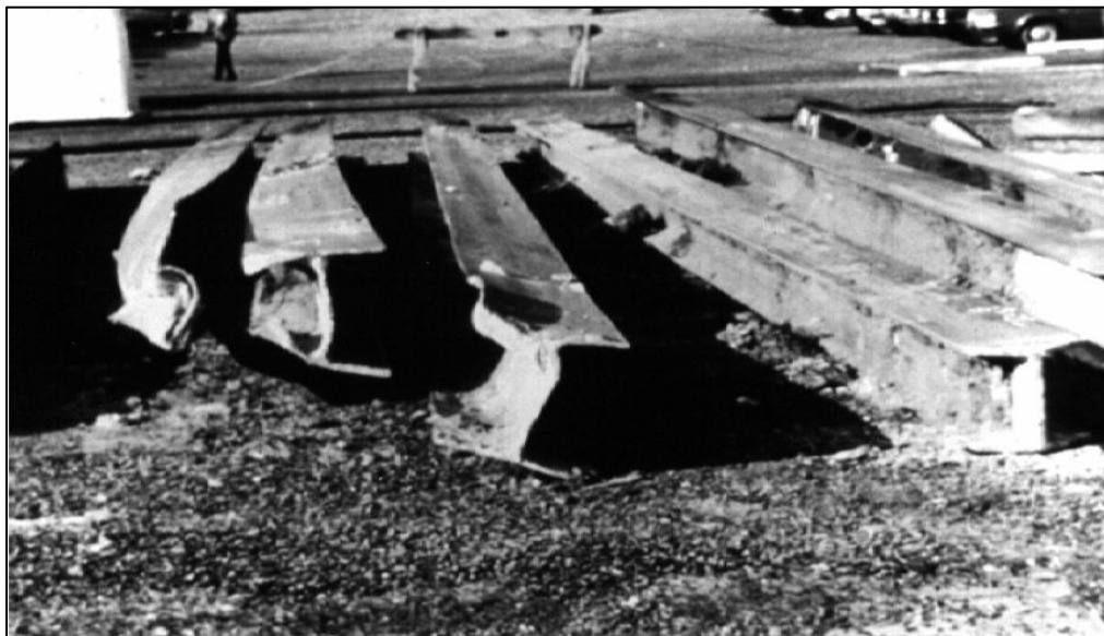
Figure 1-4: Damaged H-Pile Toe (Hannigan et al. 2006)
