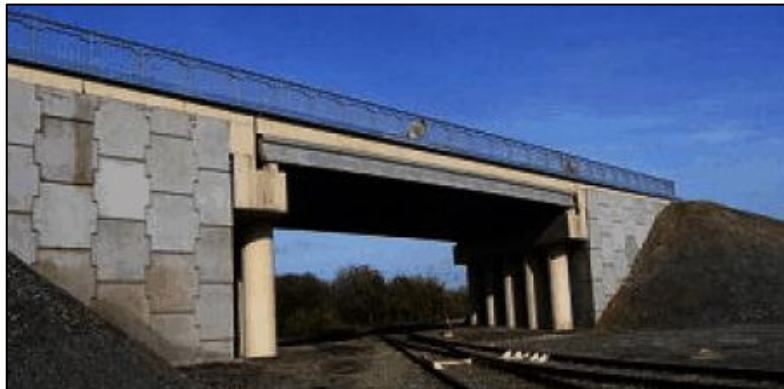
Figure 2-5: Saint Pierre La Cour Bridge in France after Completion (Behloul 2006)
