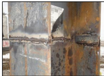
Figure 5-24: Steel HP 12 x 53 Butt-Weld Splice
