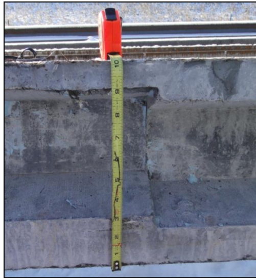
Figure 5-17: Change in the Flange Thickness of P3
