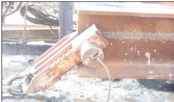
Figure 6-17: Steel HP 10 x 57 Production Pile Pickup Point
