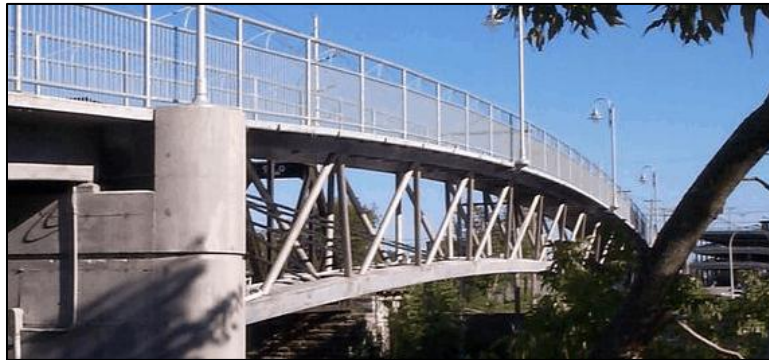
Figure 2-3: Sherbrooke Pedestrian Bridge, Quebec, Canada (Ductal 2012)
