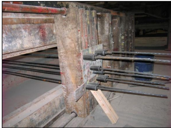
Figure 4-8: Prestressing Strands Layout at the Anchorage end
