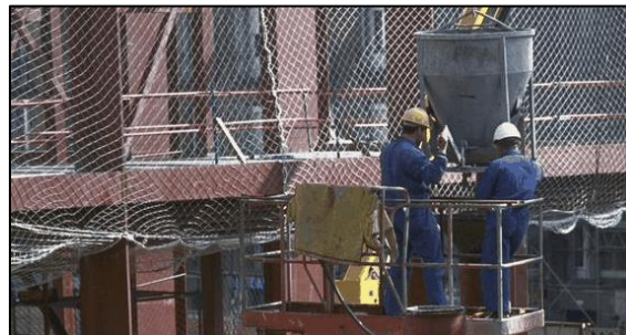
Figure 2-8: Onsite Pour for UHPC Columns during Queen Sofia Museum Expansion (Ductal 2012)
