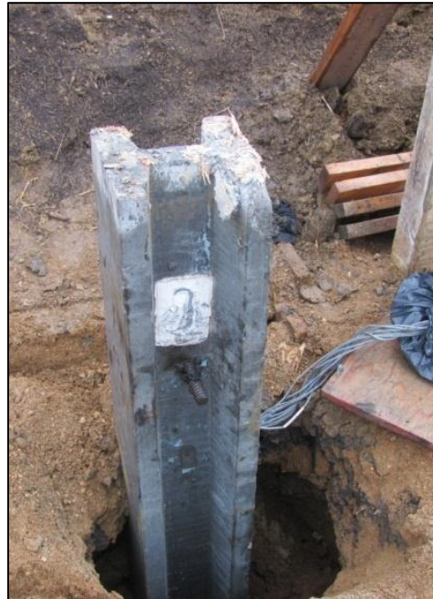
Figure 6-20: UW1-2 after Installed in the Prebore Hole
