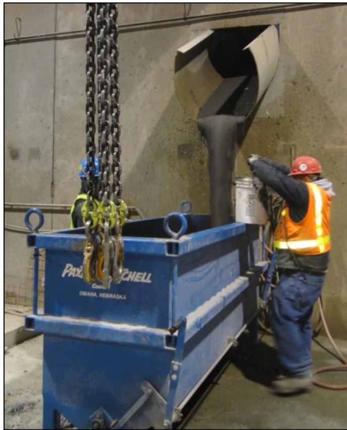
Figure 5-13: Transfer of UHPC from Mixer to Bin
