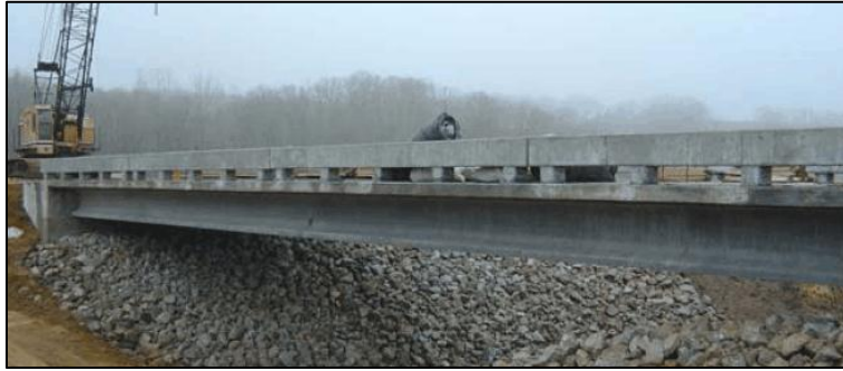
Figure 2-4: The UHPC Girder Bridge in Wapello County, Iowa (Wipf 2009)
