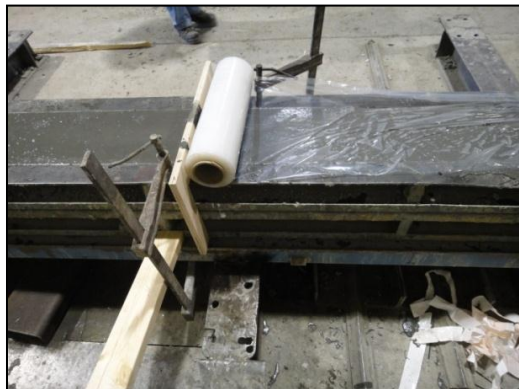
Figure 6-12: Plastic Wrap Cover for UW1-2 at the End of Casting
