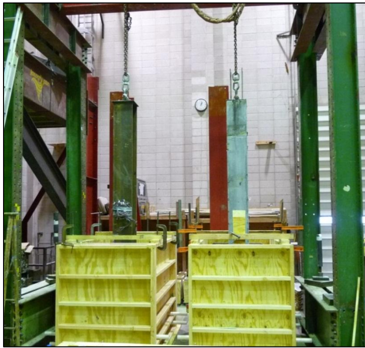
Figure 4-11: Setup used for Casting of the Abutment Cap
