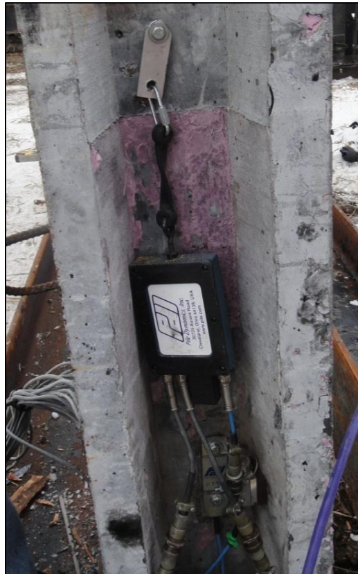
Figure 5-28: Attached PDA Equipment during the Installation of P3
