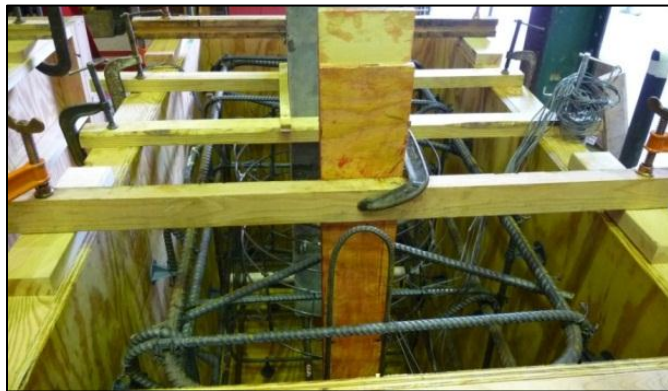
Figure 4-10: Abutment Cap Steel Reinforcement Inside of Forms
