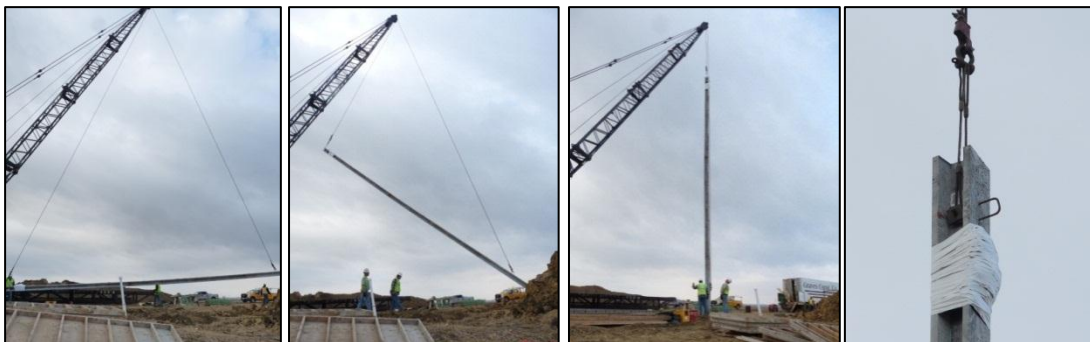
Figure 6-18: Stages in Lifting UW1-2
