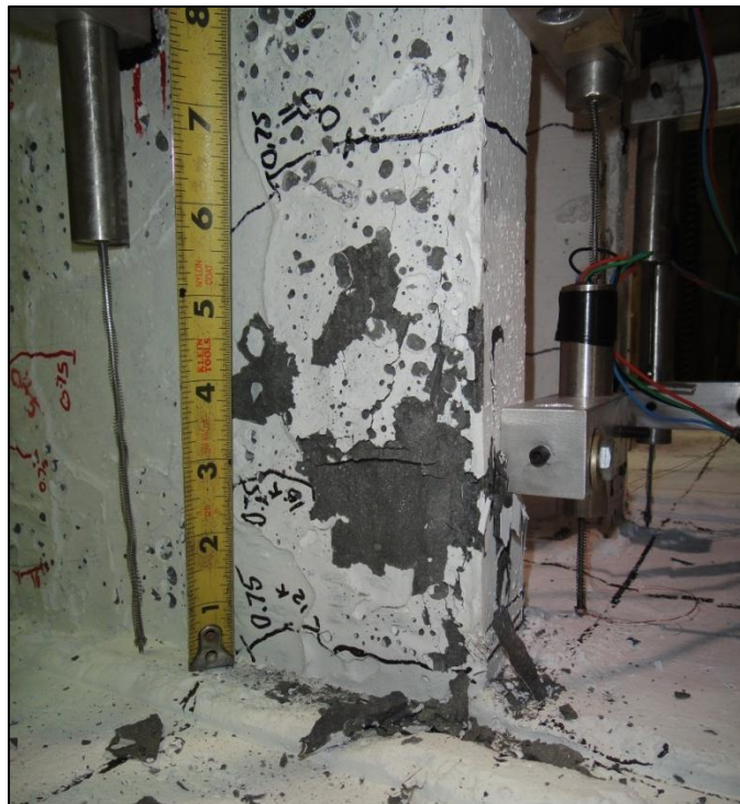
Figure 4-23: Spalled Region of the UHPC Pile Due to Crushing during the UPAC-2 Test after Completing of the 1.0-in. Load Displacement Cycles
