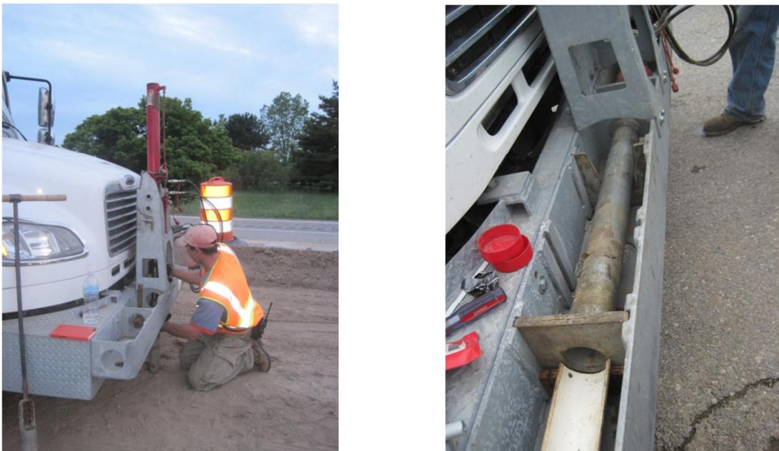
**Figure 7. Shelby tube sampling; subgrade sample retrieval (left),
