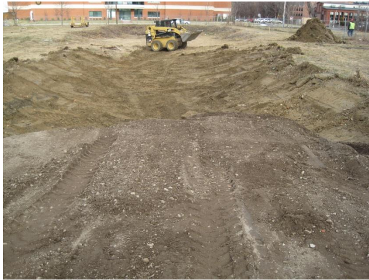
Figure 61. Hard Pack placement
