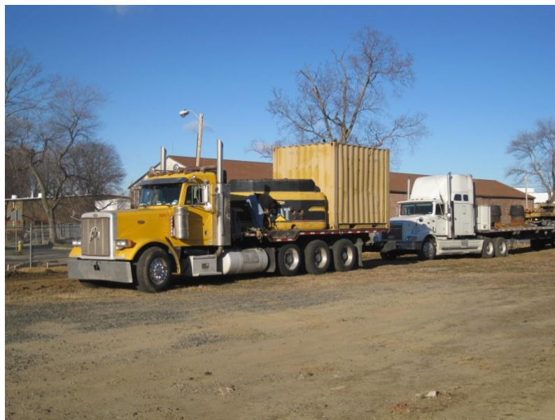
Figure 55. Mobilization of excavator back end and RIC supplies
