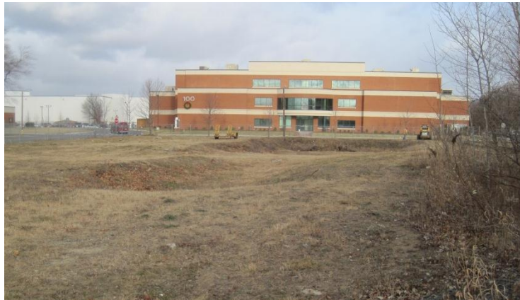
Figure 60. Depression on site prior to backfilling
