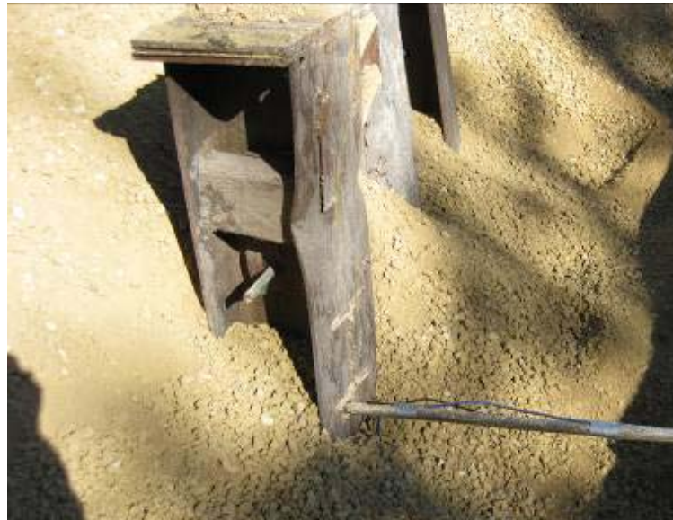
Figure 5-21. Tie rod to H-pile connection.
