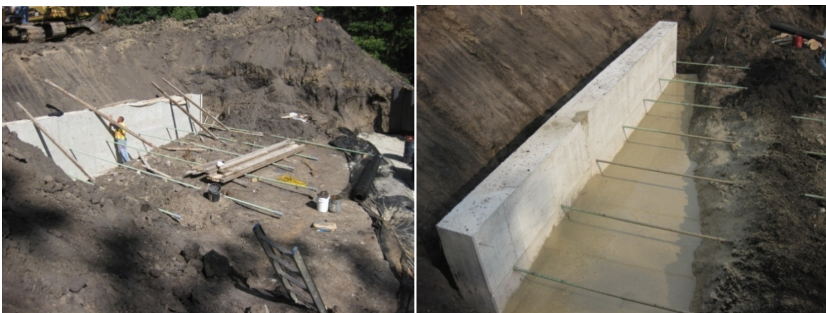
Figure 5-74. Reinforcement placement for concrete deadman.
