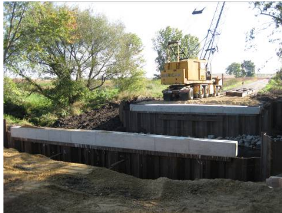
Figure 5-22. Placement of abutment caps on sheet pile walls.
