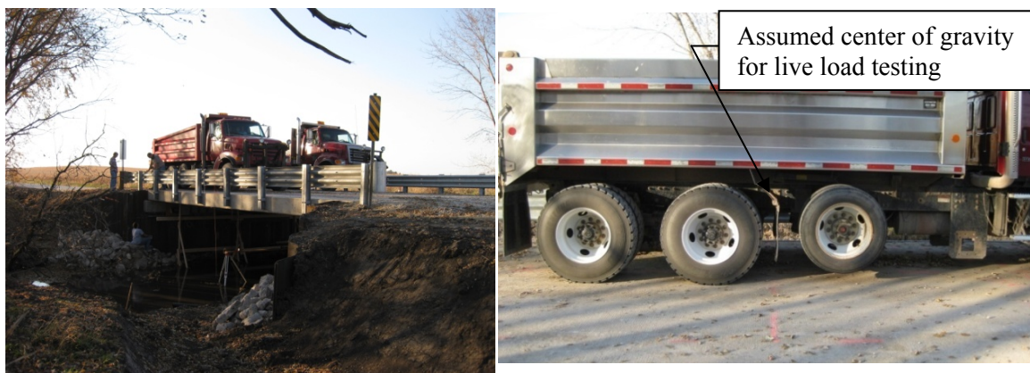
a.) Overview of load testing
