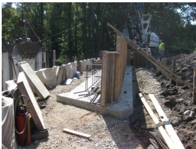
Figure 5-83. Reinforced concrete spread footing on west abutment.
