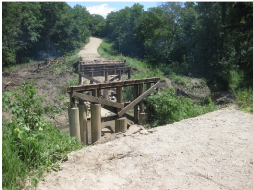
b.) Superstructure removed
