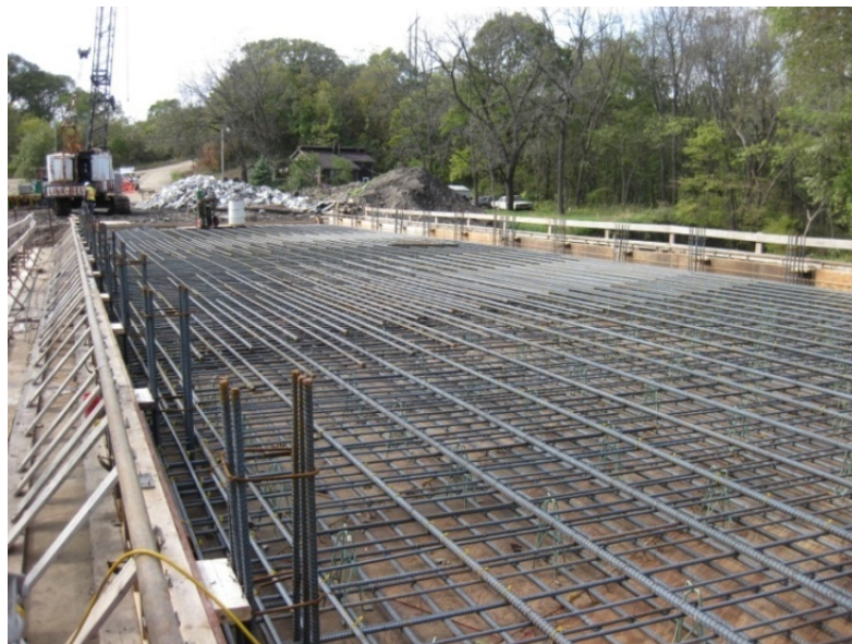
Figure 5-88. Reinforcement in place for continuous concrete slab bridge.
