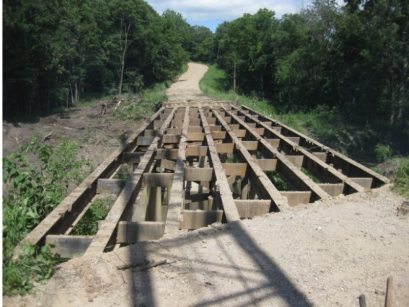
a.) Timber decking removed (exposing steel girders)
