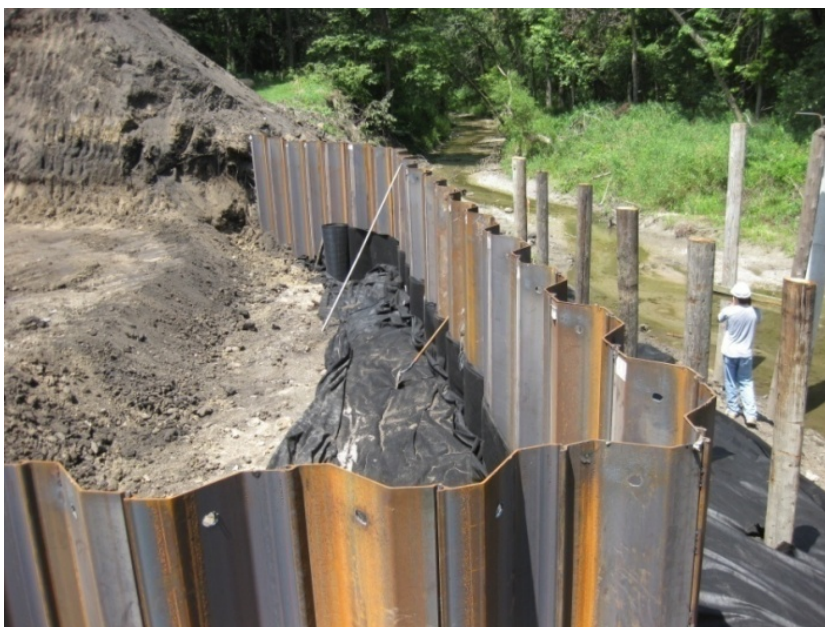
Figure 5-67. West abutment after all sheet piling in place.
