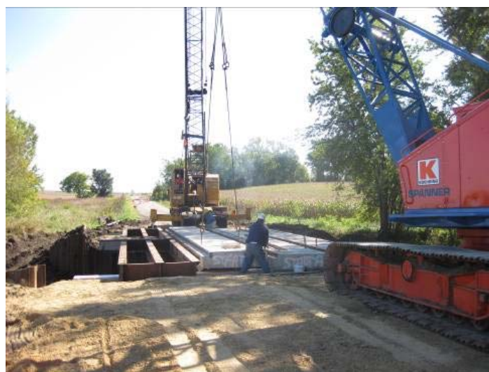
Figure 5-30. Dual crane operation for placement of bridge superstructure.
