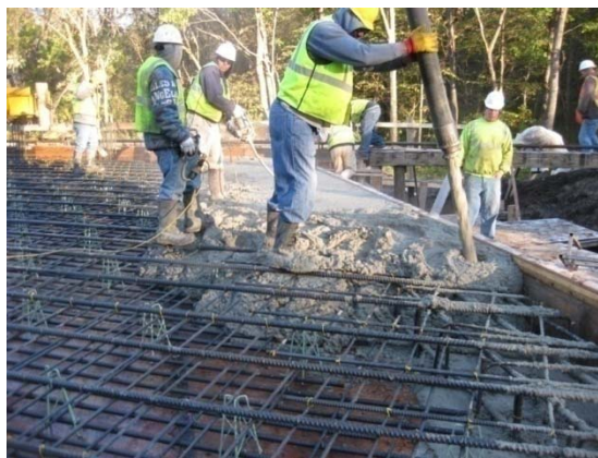
Figure 5-90. Concrete placement near east abutment with pump truck.
