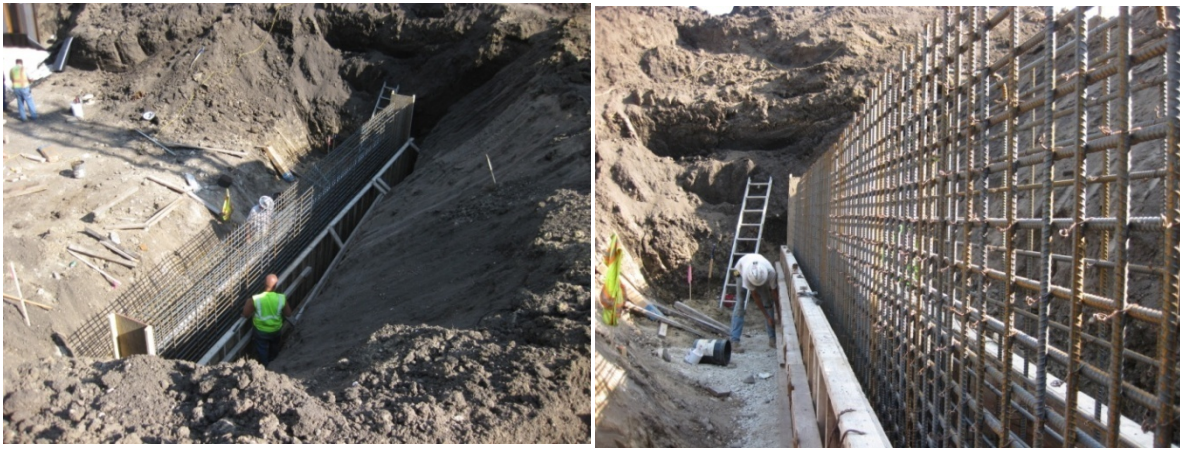
a.) Overview of deadman trench
