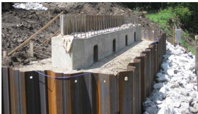
Figure 5-104. State of completion of the west abutment when zero readings were taken to determine loads and deflections for Load 1.
