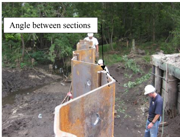
a.) Angle between sections
