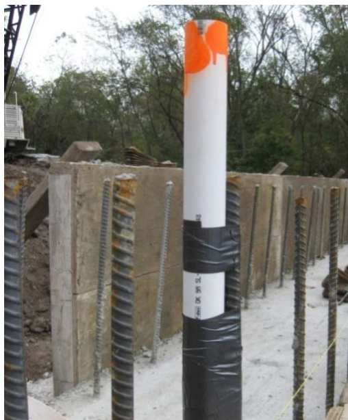
a.) Before placement of the bridge deck
