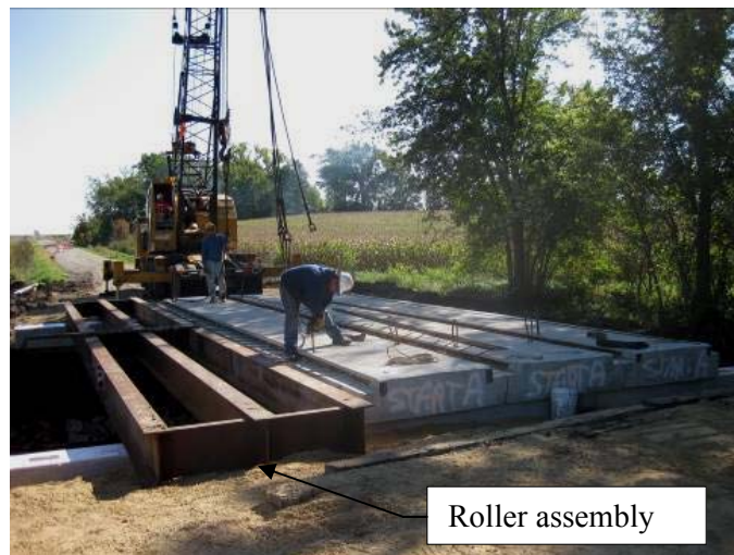
Figure 5-29. Roller assembly used to assist in placement of deck elements.
