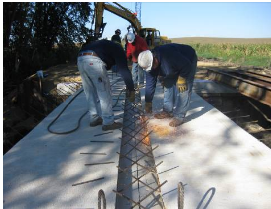
Figure 5-31. Finishing of bridge deck joints.
