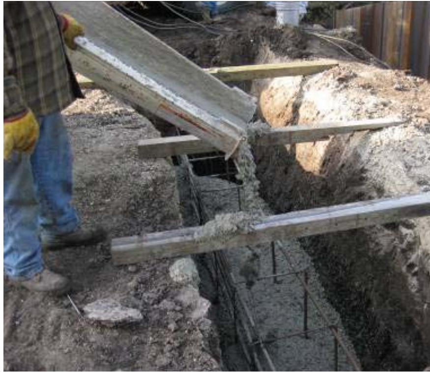
Figure 5-19. Reinforced concrete deadman placement behind east abutment.
