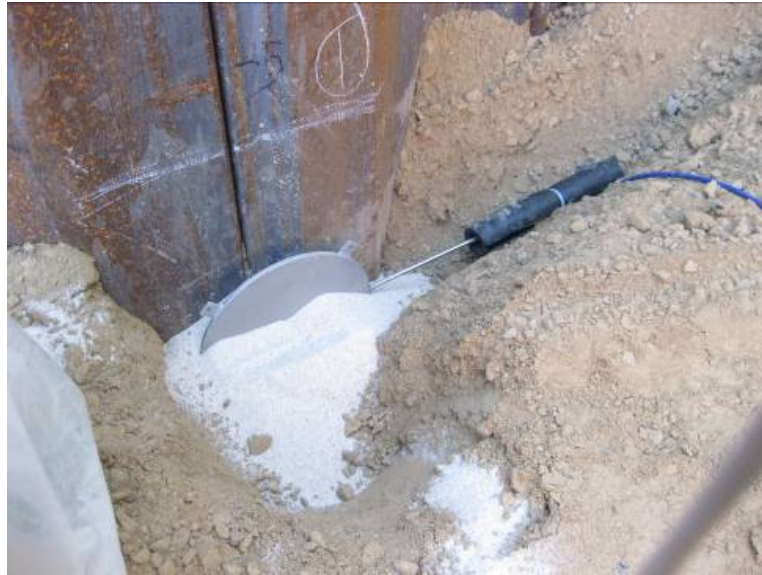
Figure 5-24. Earth pressure cell installation.
