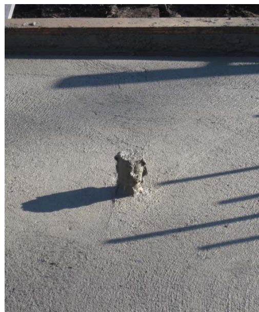
b.) After placement of the bridge deck
