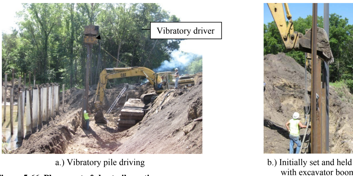
Figure 5-66. Placement of sheet pile sections.
