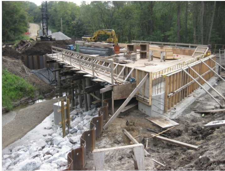
Figure 5-87. Construction of falsework for placement of bridge deck.
