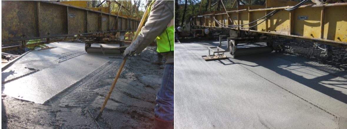
a.) Unfinished concrete after placement
