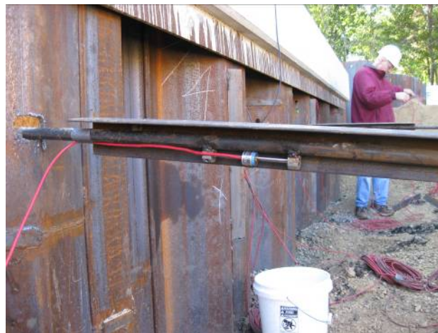
Figure 5-23. Tie rod strain gage installation.
