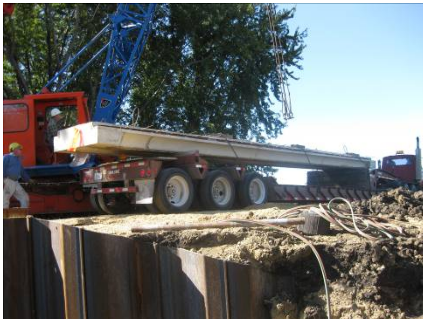
Figure 5-28. Precast beam-in-slab bridge deck element.
