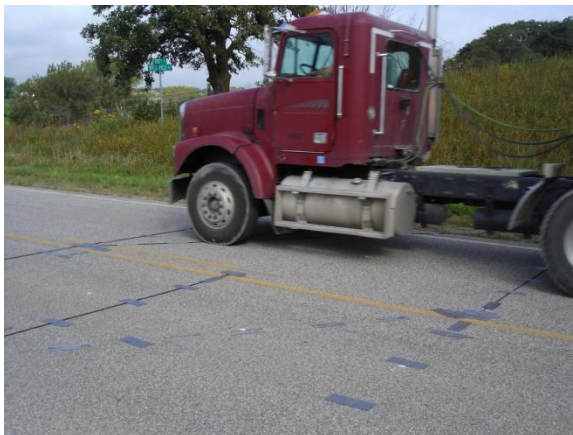
FIGURE G-4 Heavy vehicle in the inside lane
