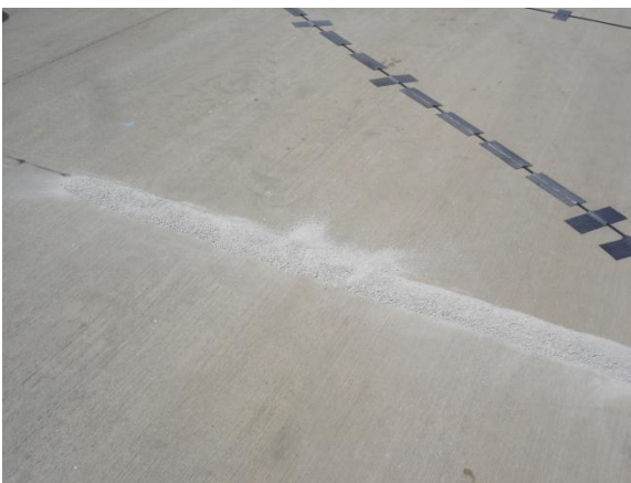
FIGURE F-9 Aggregate ridge after vehicle crossing
