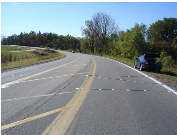
FIGURE G-19 Sta. B z-configured road tubes
