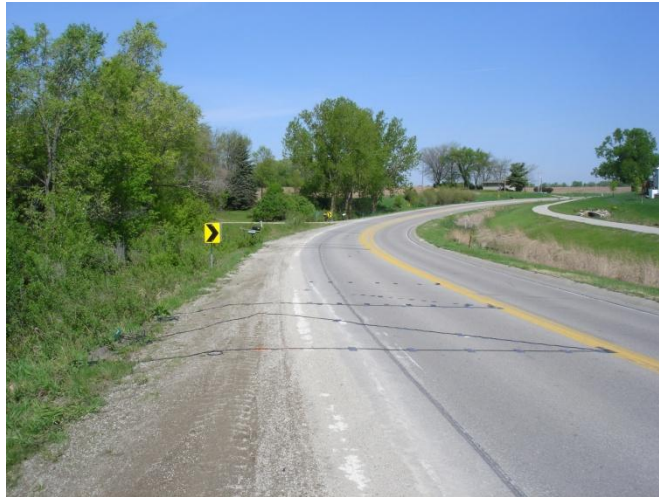
FIGURE F-10 Seven z-configured road tubes from the CC to the PC
