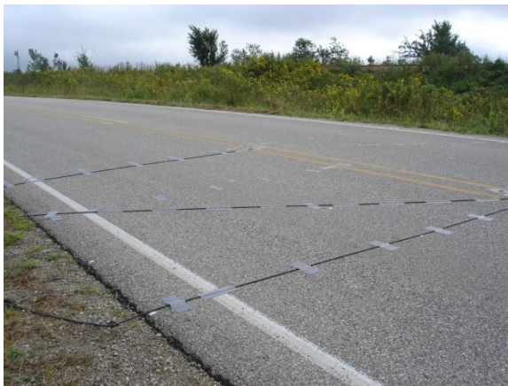
FIGURE G-2 Sta. B z-configured road tubes
