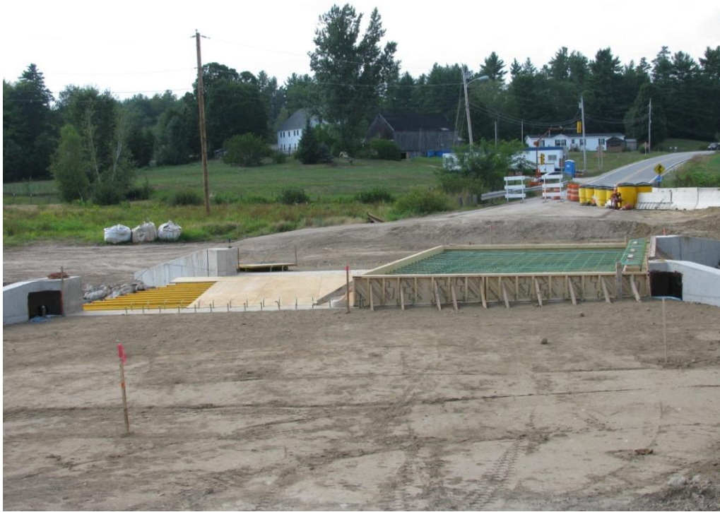
Figure 1 Route 107 bridge deck in Epsom, NH.
