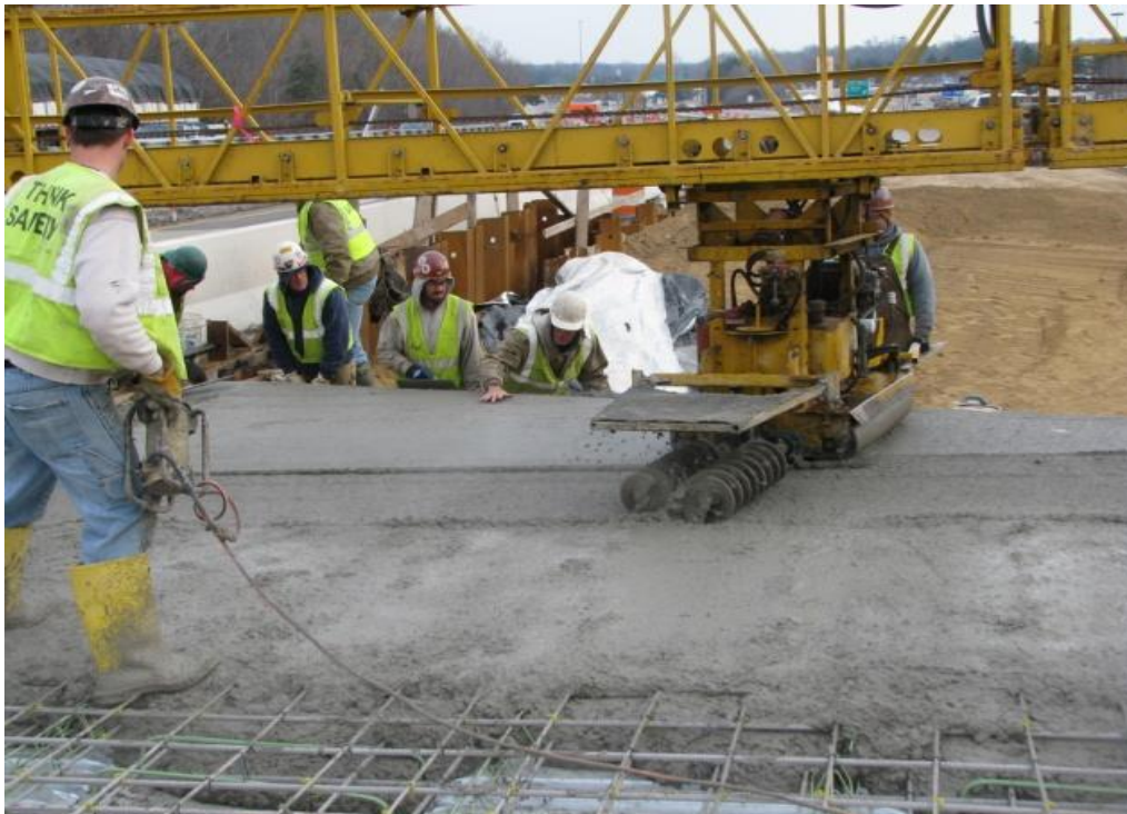
Figure 8 Concrete being placed.
