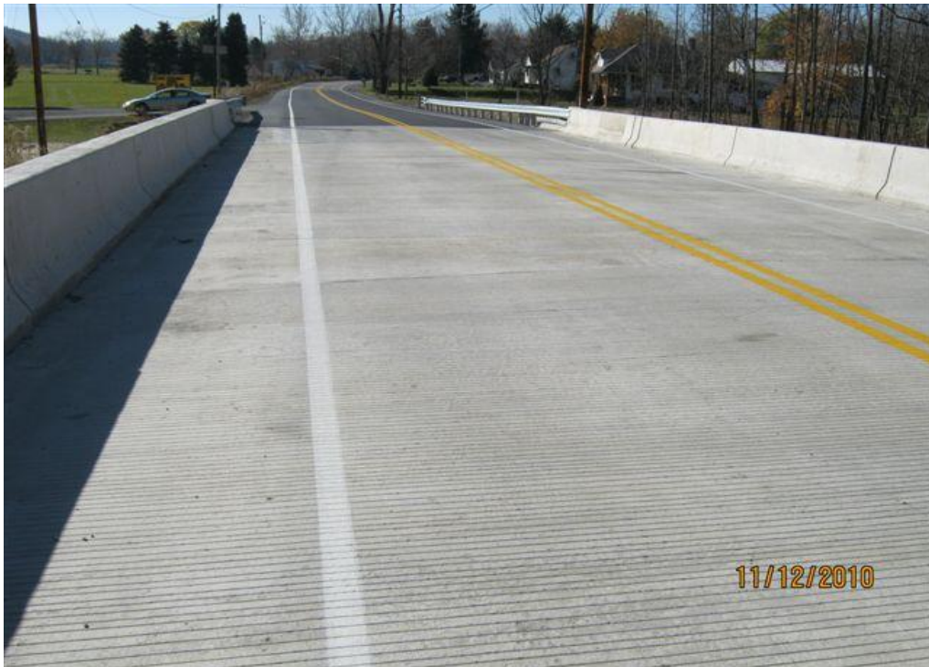
Figure 14 Bridge deck surface at four months after being constructed.
