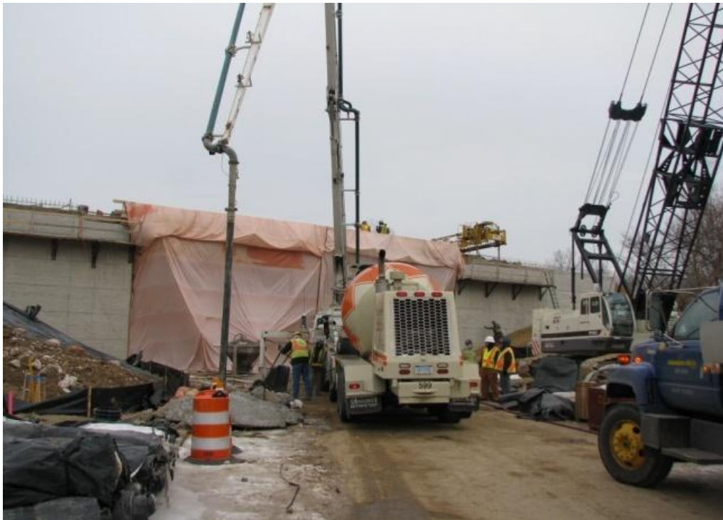
Figure 10 Concrete heated tent enclosure.
