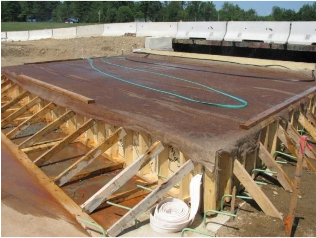
Figure 13 Concrete being cured with burlap.
