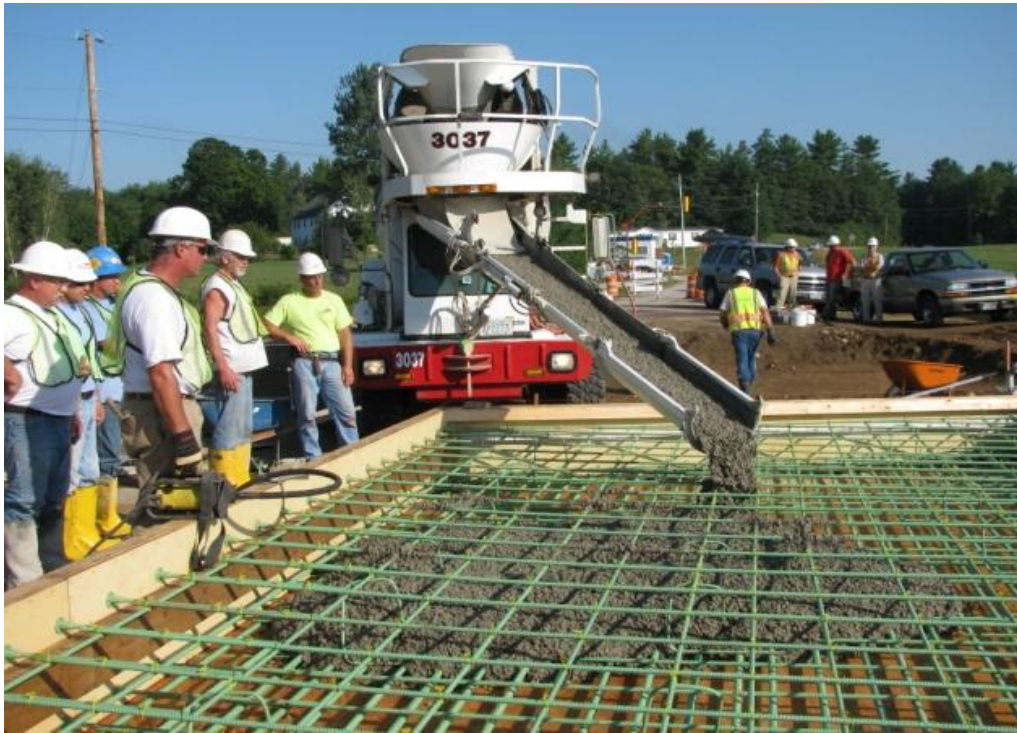
Figure 7 Concrete being placed.
