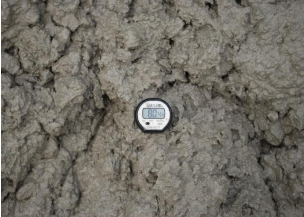
Figure 13 Concrete temperature being tested by sensor.
