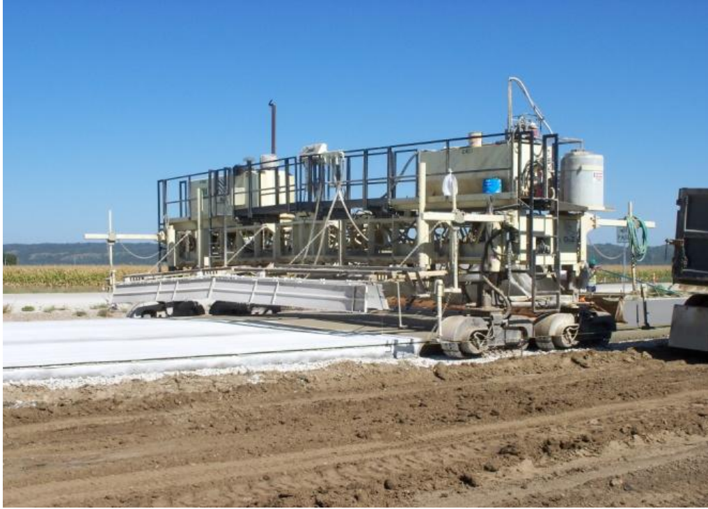
Figure 11 Concrete being finished and curing compound being applied.
