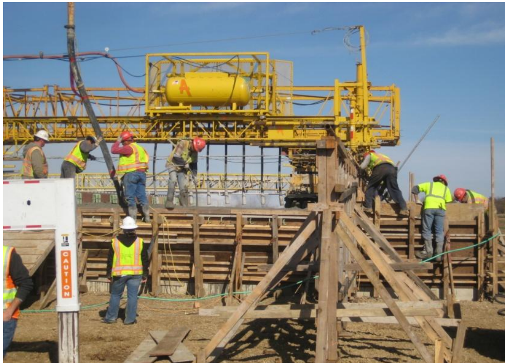
Figure 10 Concrete being placed and vibrated.
