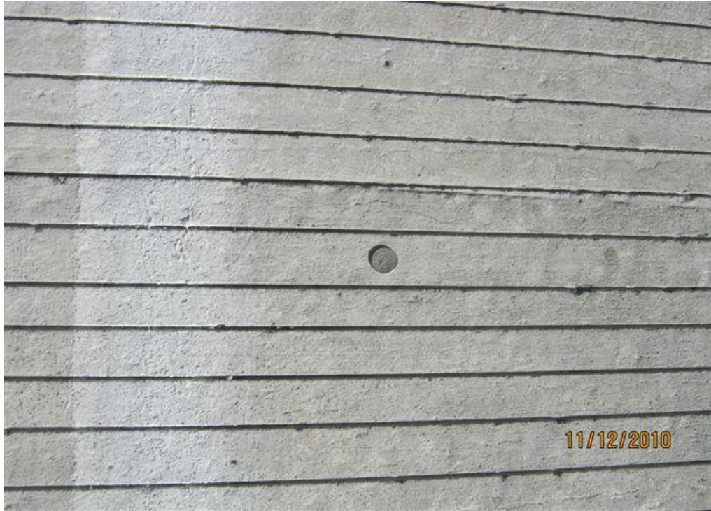
Figure 15 Bridge deck surface at four months after being constructed.
