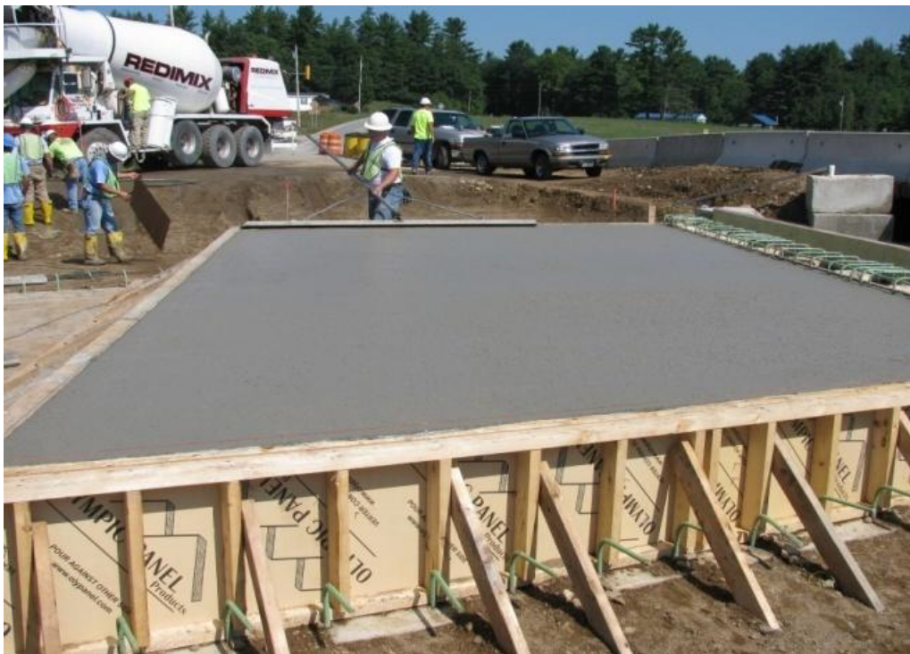
Figure 12 Concrete being finished.
