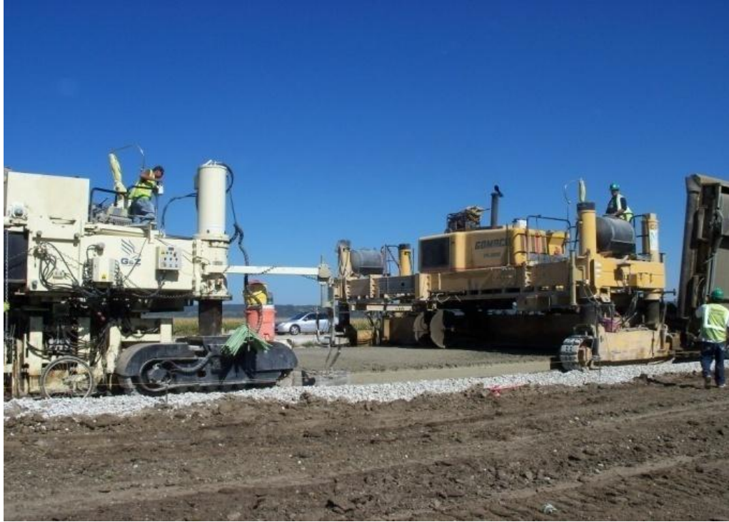
Figure 9 Concrete passing through the paver.
