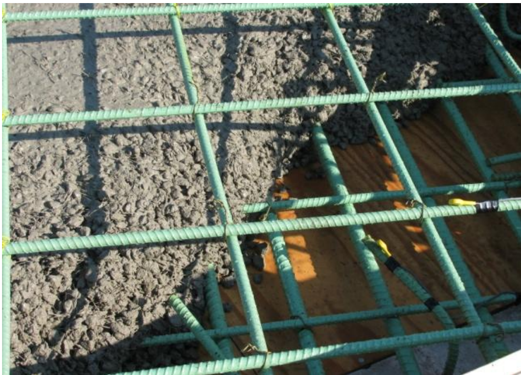
Figure 10 Two i-buttons being placed.
