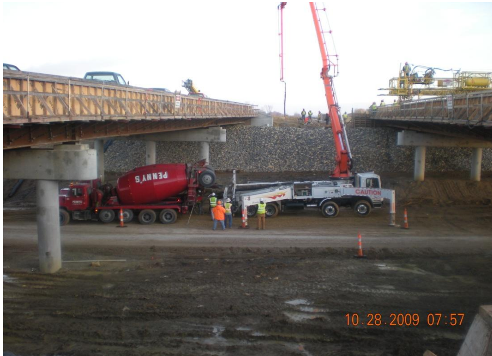
Figure 1 US-59 Bridges (Southbound-left and Northbound-right).
