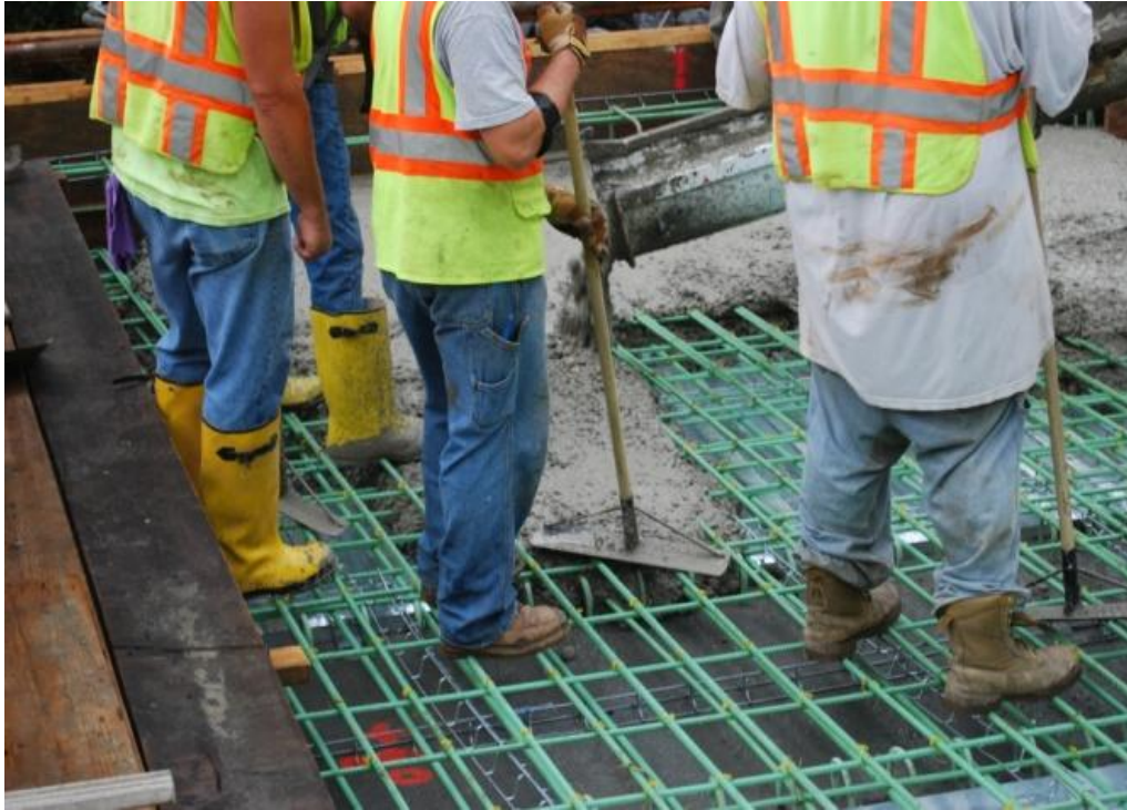
Figure 7 Concrete being spread by construction crews.
