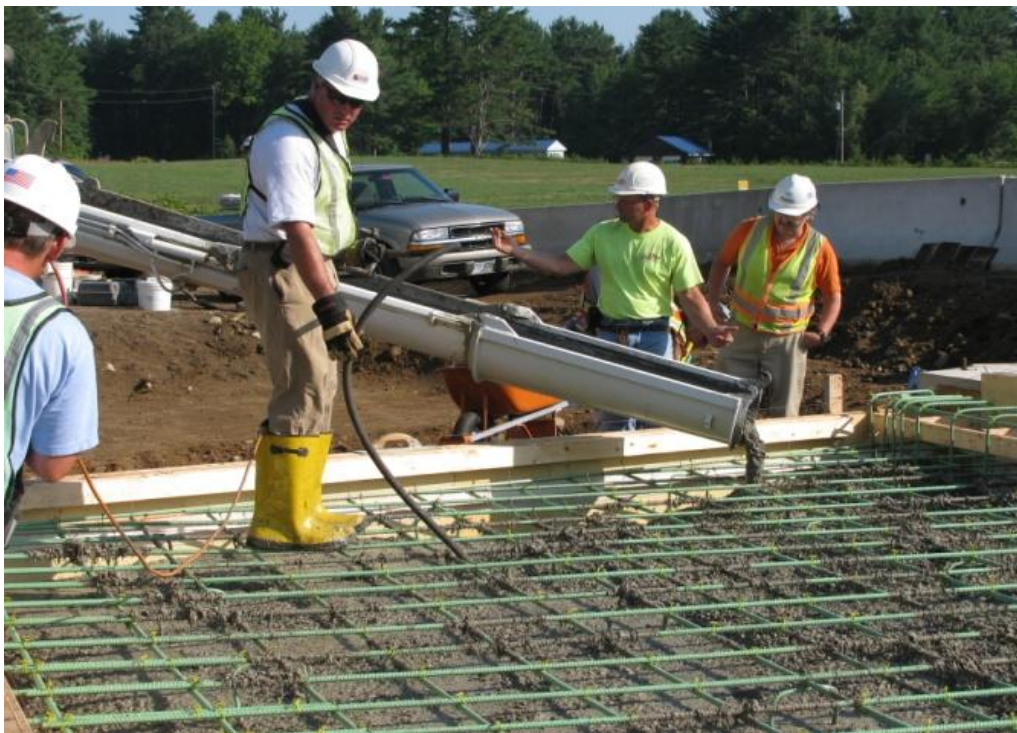
Figure 8 Concrete being vibrated.
