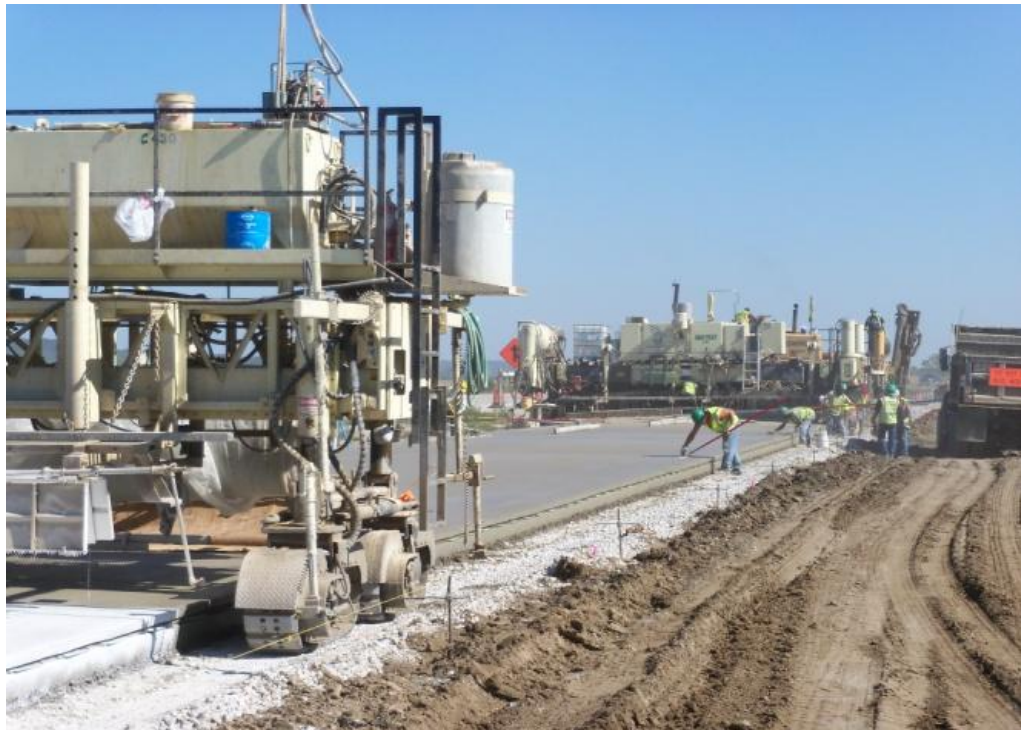
Figure 10 Concrete being finished and curing compound being applied.
