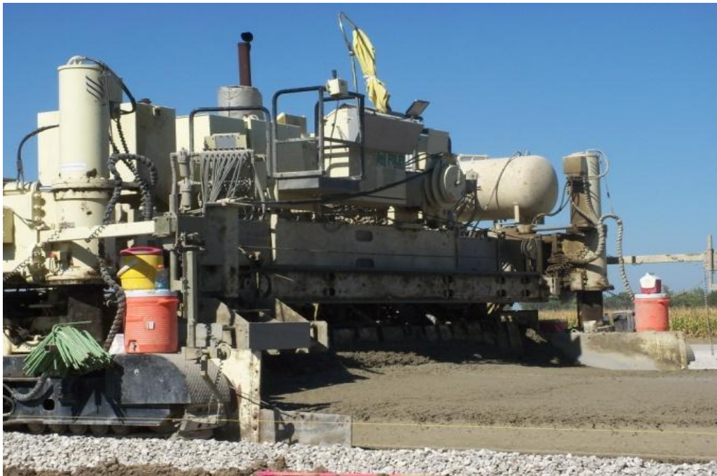
Figure 8 Concrete passing through the paver.
