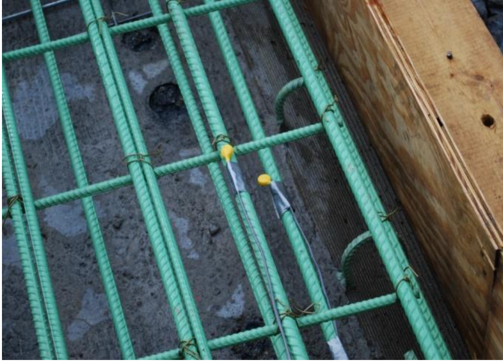
Figure 11 Two i-buttons being embedded on site.
