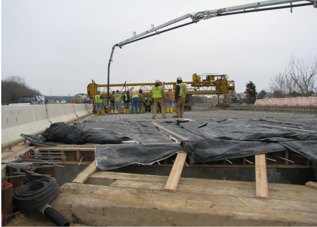
Figure 1 I-94 Riverside drive bridge deck placement.
