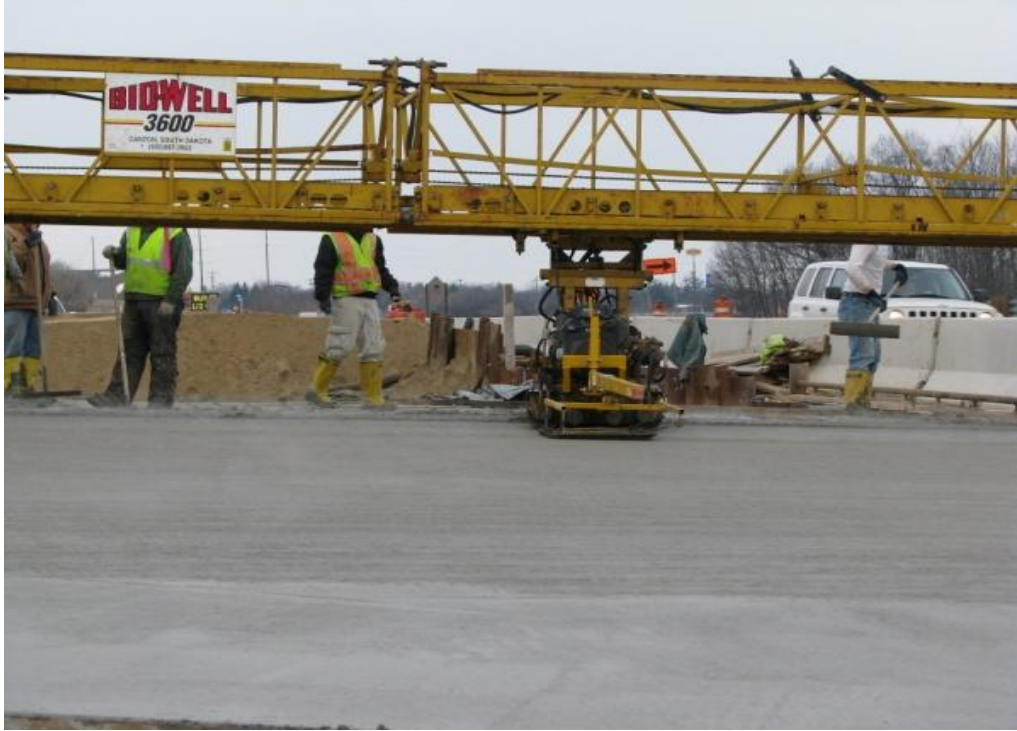
Figure 9 Concrete being finished.
