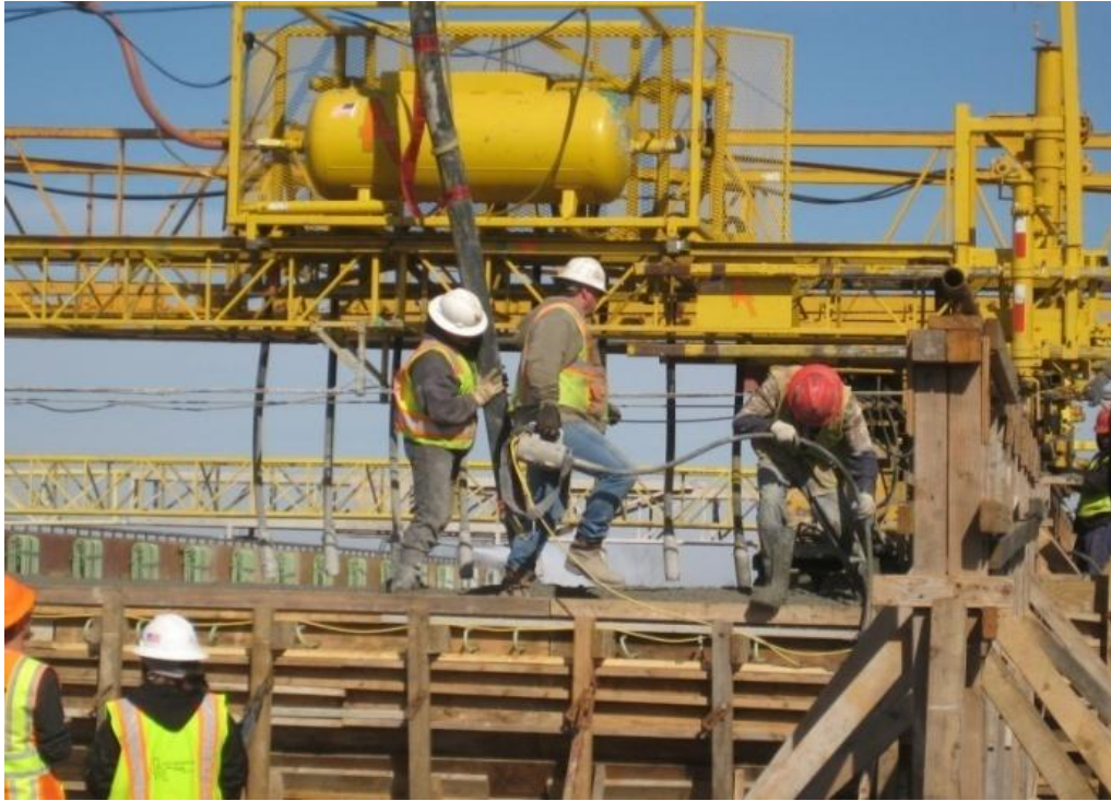
Figure 7 Construction crew placing concrete pouring and vibrating.
