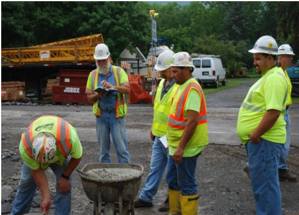
Figure 6 Concrete being tested by Penn DOT technicians .
