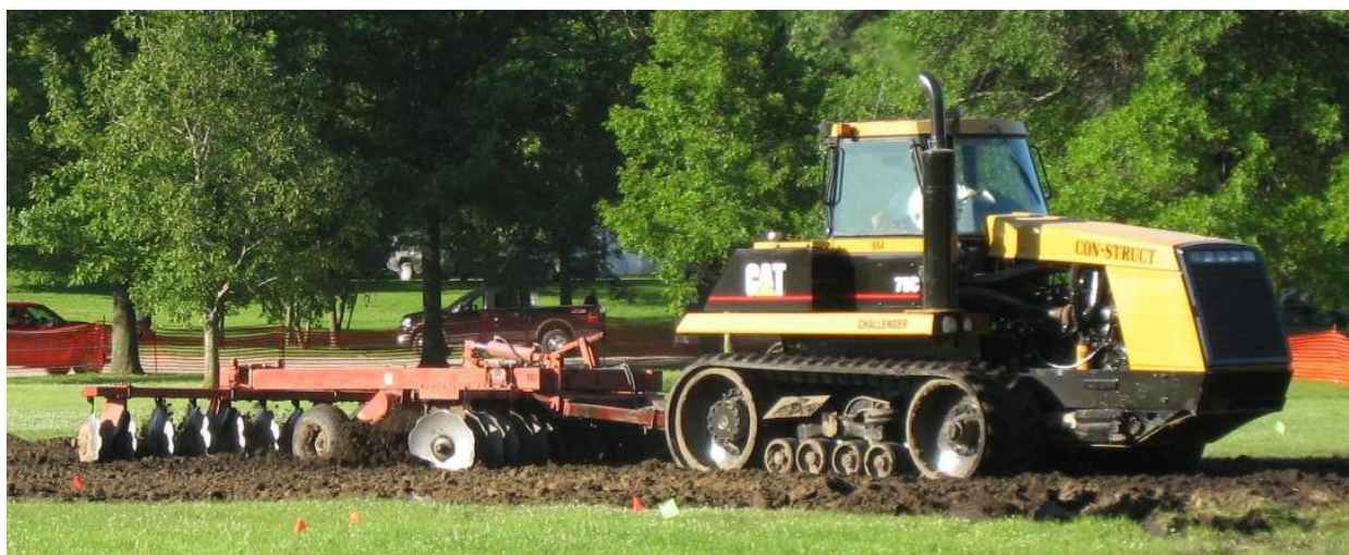
Figure 19. Disking method for soil drying. Propane forced air heaters could be added onto the trailer to reduce drying times (Blahut 2010).
