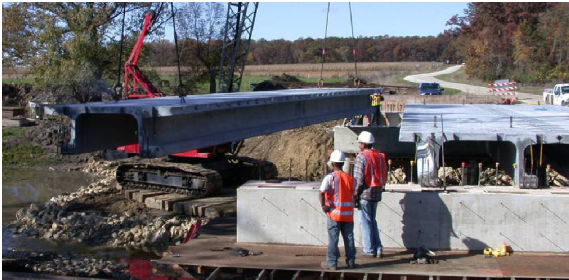
Figure 2.11: Installation of the Second Generation UHPC Pi-Girder on the Jakway Bridge in Buchanan County, Iowa (Bierwagen, 2009)
