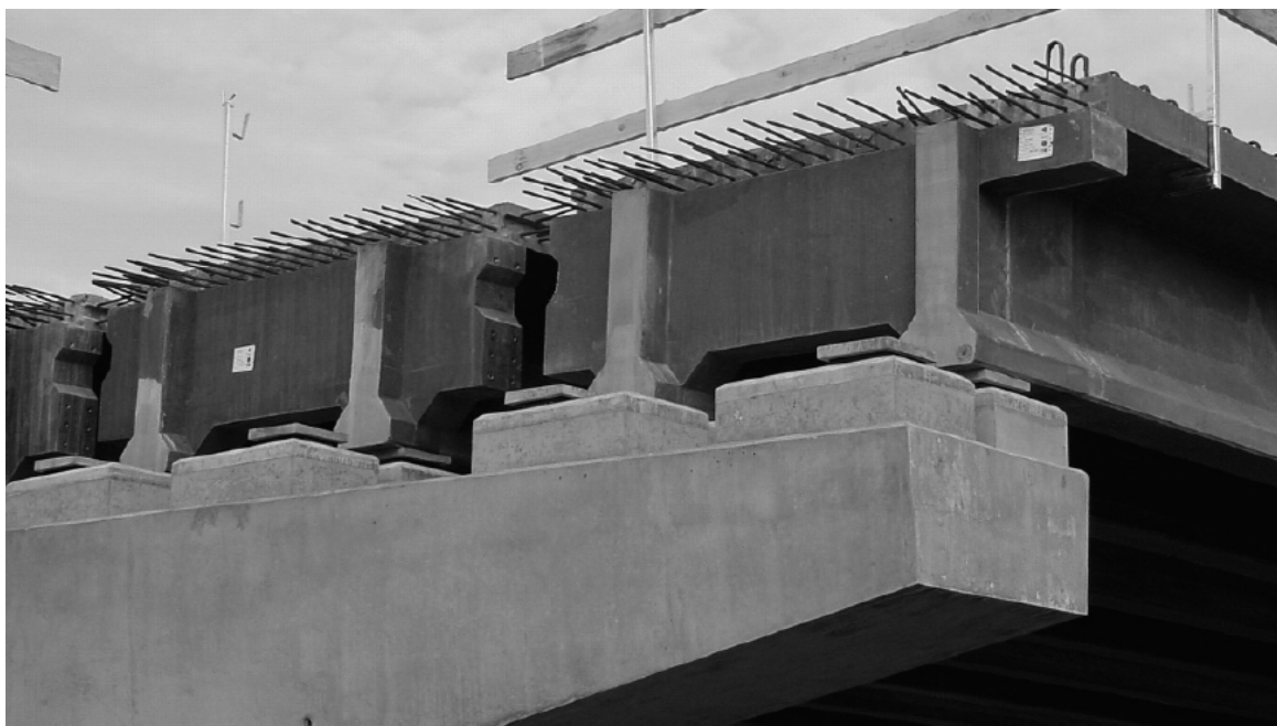
Figure 2.9: UHPC Pi-Girders in the Bourg-les-Valences Road Bridge in France (Vergoossen, 2008)
