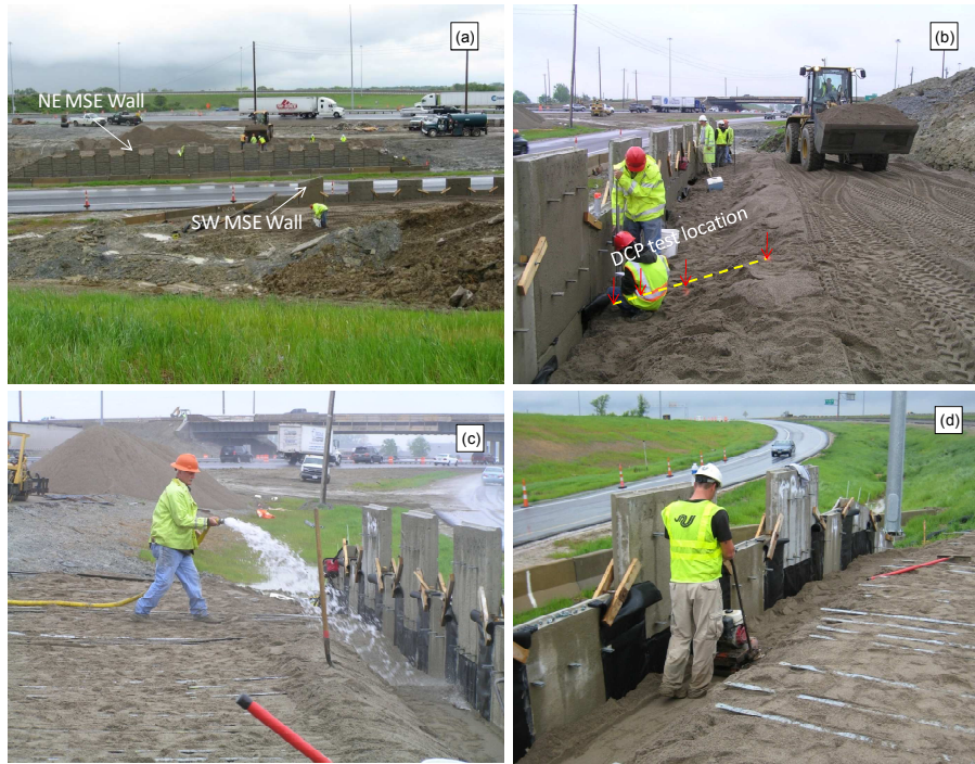
Figure 57. Bridge #1(BUT-75-0660) at I-75 &SR 129 interchange: (a) location of south and north MSE walls; (b) DCP test locations; (c) watering of backfill prior to compaction; (d) compaction of backfill next to the wall
