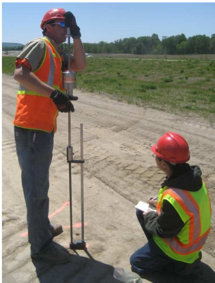
Figure 14. Dynamic cone penetration test
