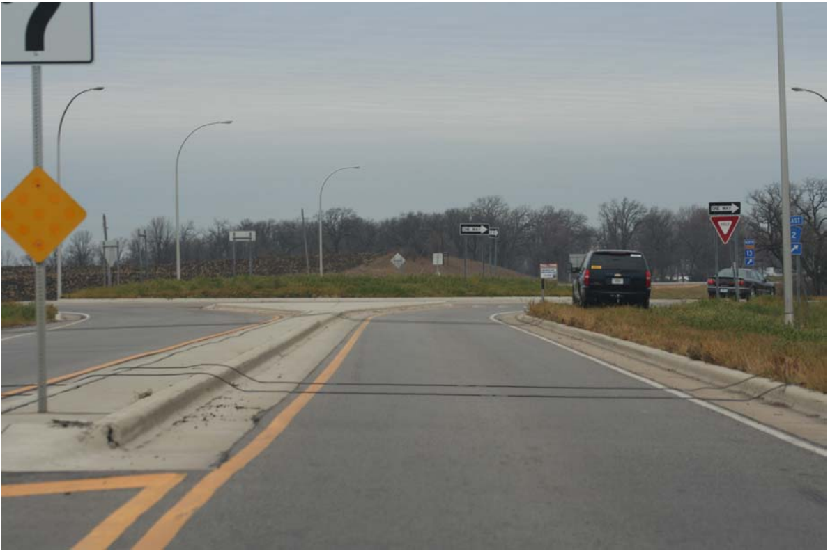
FIGURE 3. Road tube layouts at 250 ft and 100 ft from yield line in Minnesota
