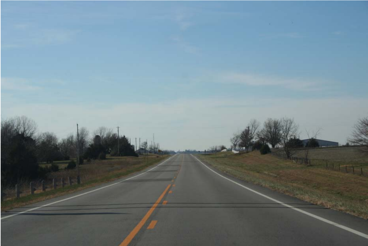
FIGURE 1. Photo showing road tubes at 1,500 ft and series of three rumble strips Layouts and Data Collection
