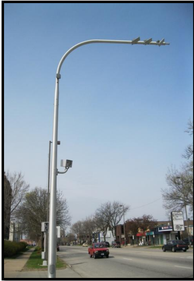
Figure 7: Mast arm and RF Antenna Set up
