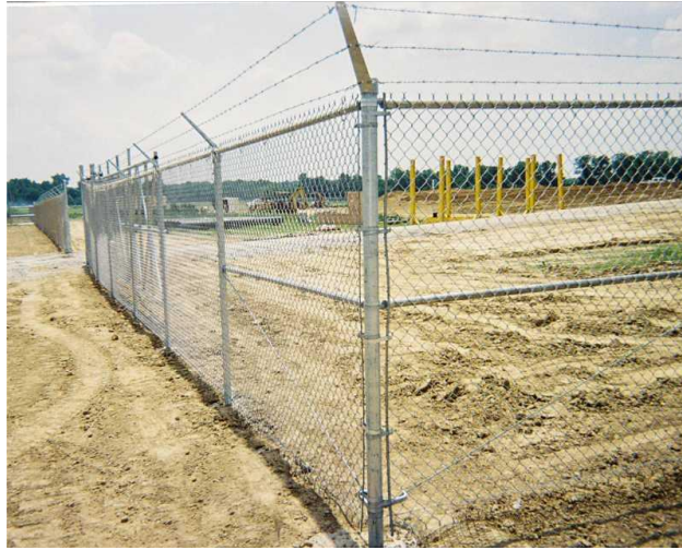
Figure 6: Chain Link Fence with Barbed Wire at 45-Degree Angle
