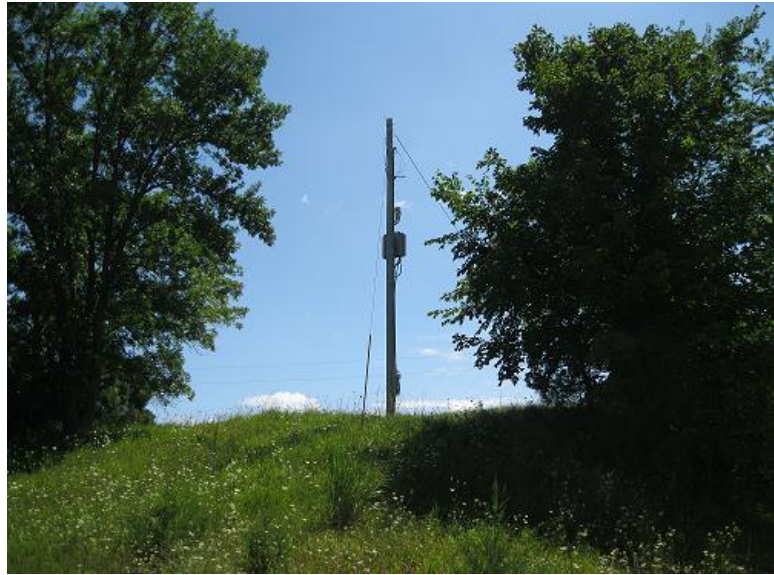
Figure 44: Holliwell Pole from Bridge
