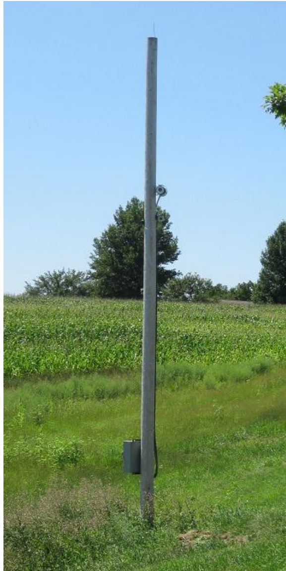
Figure 65: Complete Pole after Installation
