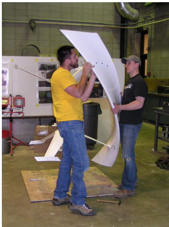
Figure 36: Assembly of 600 watt VAWT
