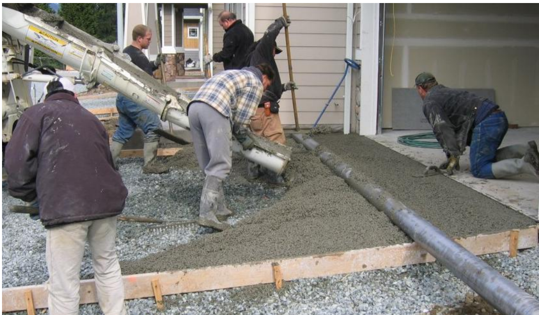
Figure 2-15. A Temporary Wood Spacing is Pre-placed (Adopted from [54])
