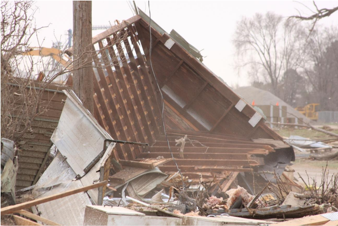
FIGURE 2-3 DAMAGE FROM THE MAPLETON, IOWA TORNADO OF APRIL 10, 2011 SHOWING AN ENTIRE ROOF LIFTED OFF OF ITS SUPPORTING WALLS
