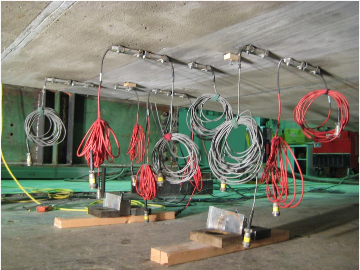
Figure 3.18. Surface Mounted Strain Gages on Top of Deck
