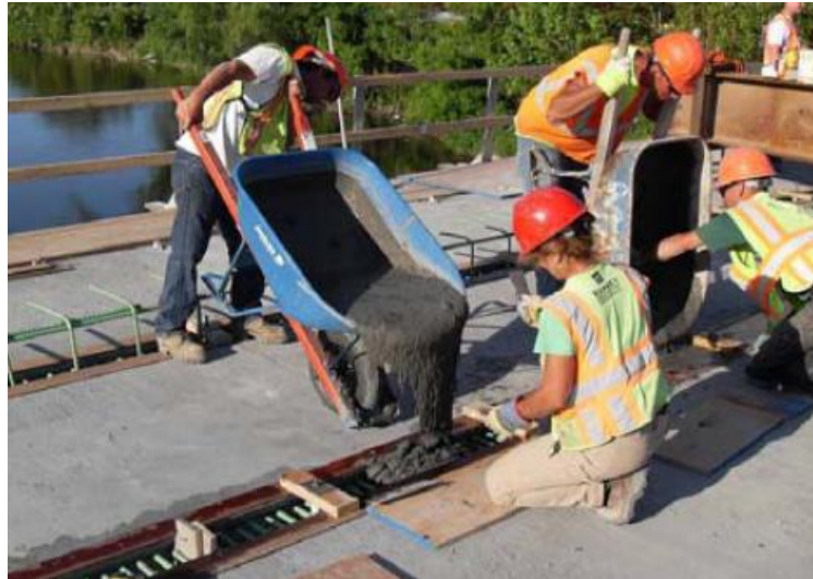
Figure 2.8. UHPC Deck Closure Joints
