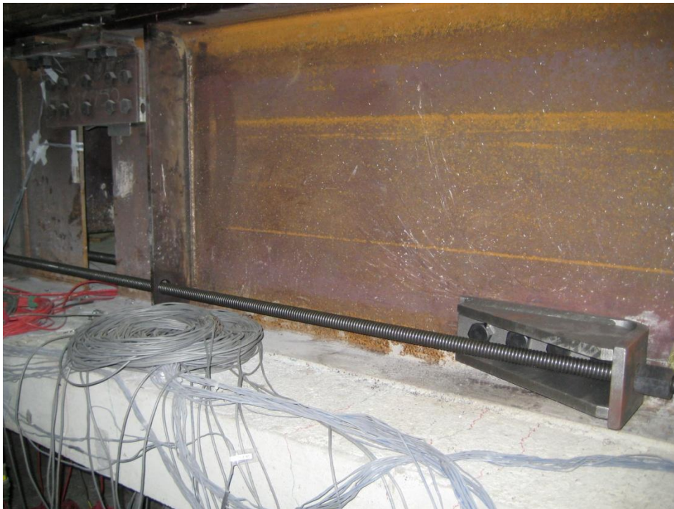
Figure 3.24. Connection Retrofit Installed
