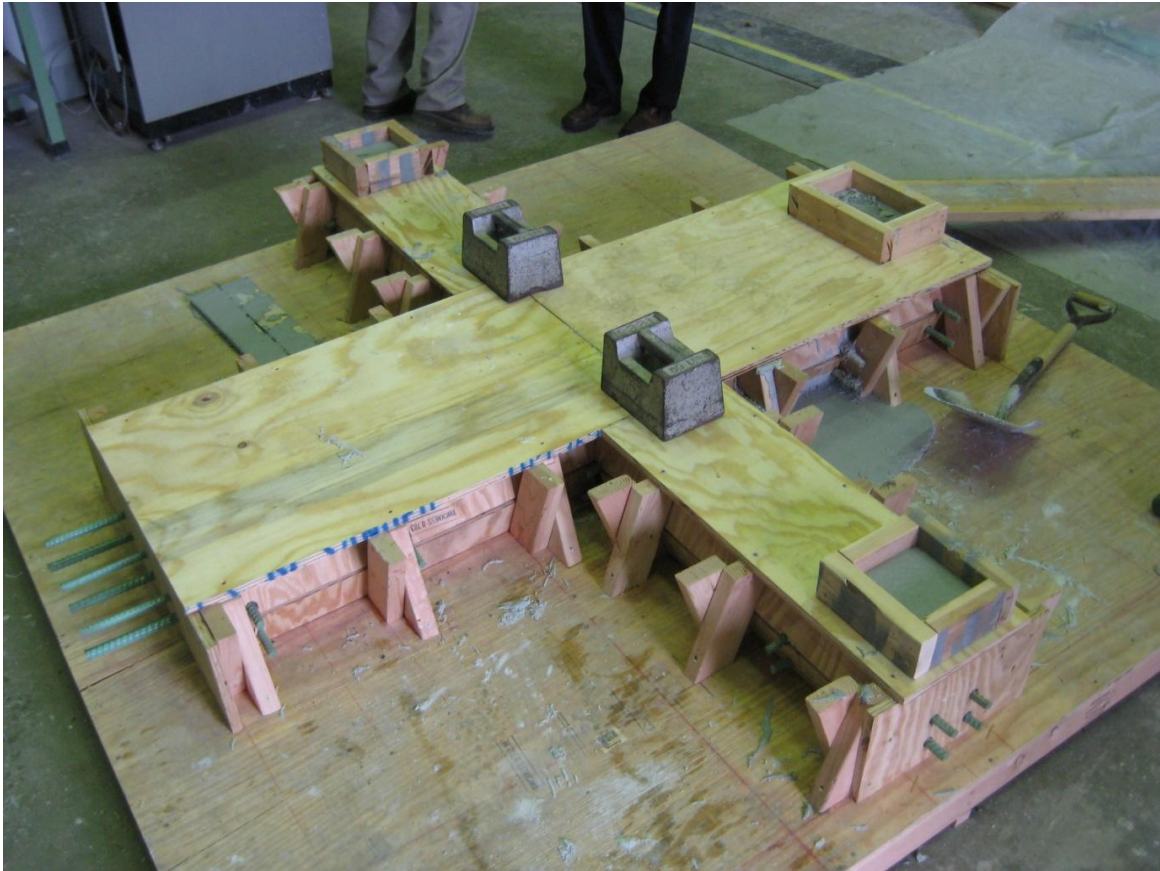
Figure 3.9. Plywood Top Forms
