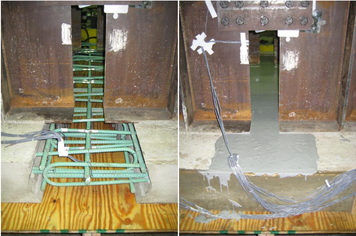
Figure 3.14. UHPC Joint Preparation and Placement
