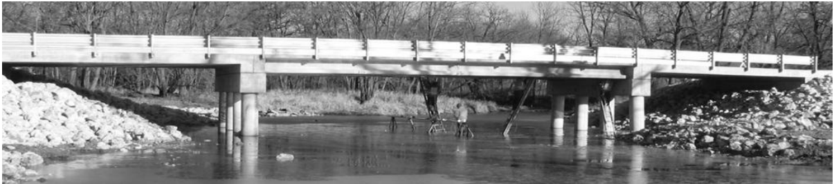
Figure 2.7. PI Girder Bridge - Buchanan County, Iowa
