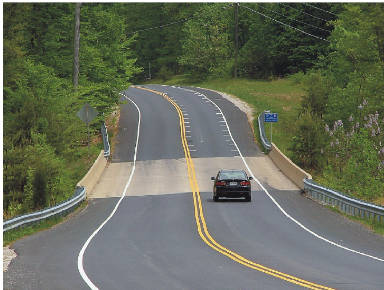
Figure 2.1 Optical speed bars (Virginia DOT)
