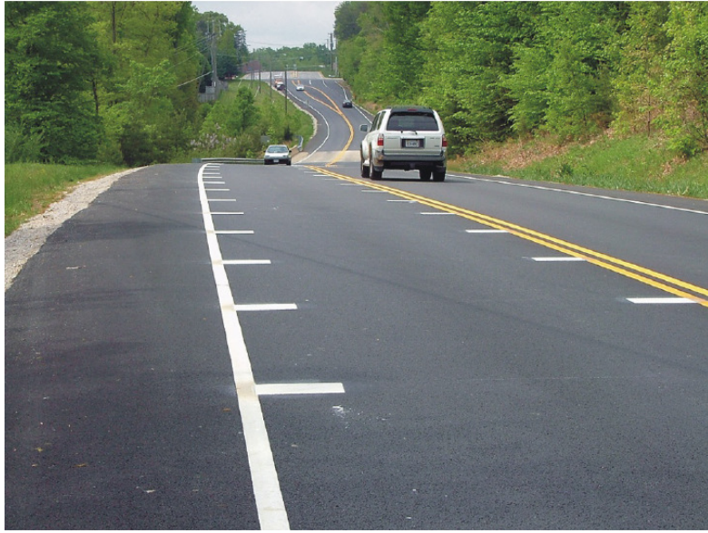
Figure 2.2 Optical speed bars close range (Virginia DOT)
