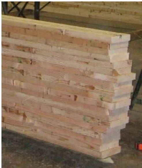
(a) Selected laminates for girder assembling
