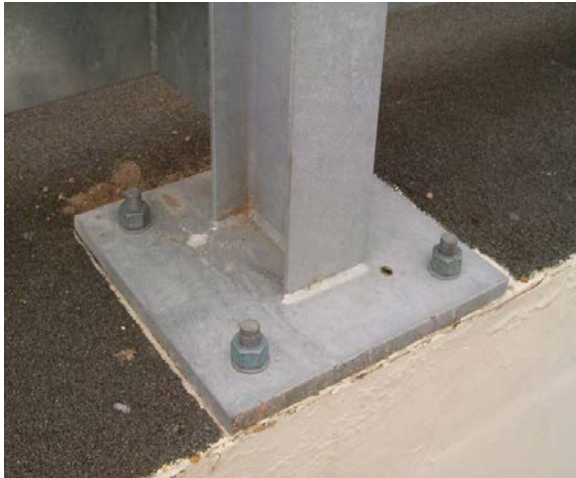
(c) Barrier rail connection
