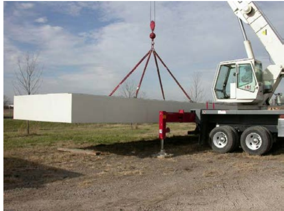
(b) FRP deck panel lifting
