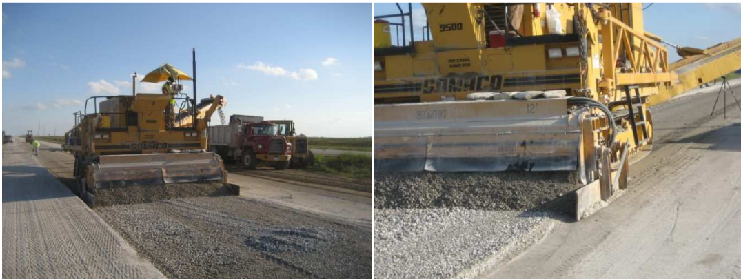
Figure 25. Trimming process for I-35 Iowa
