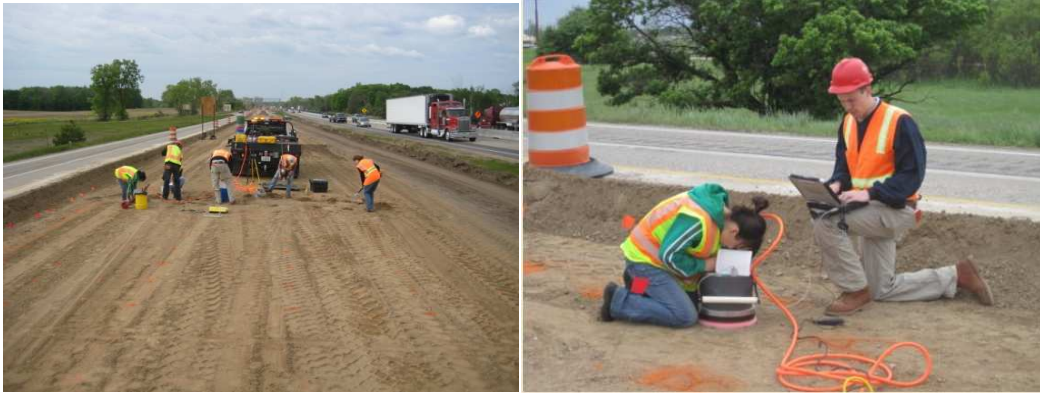
Figure 34. Overview for sandy subbase test bed (left) and GPT in situ testing on I-96, Michigan.
