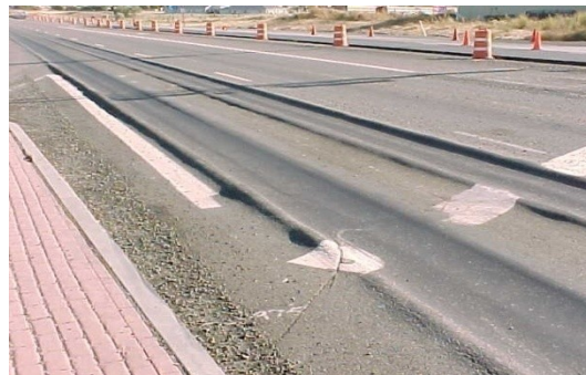
Figure 2.14A Pictorial View of Rutting
