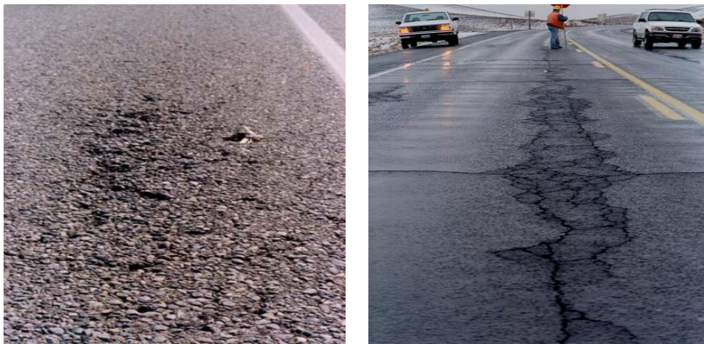
Figure 2.11 A Pictorial View of Raveling
