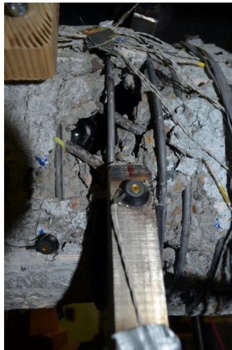
Figure 5-19: Specimen H1C3-C Close-Up of Local Failure on LED Side after Clearing Damaged Concrete
