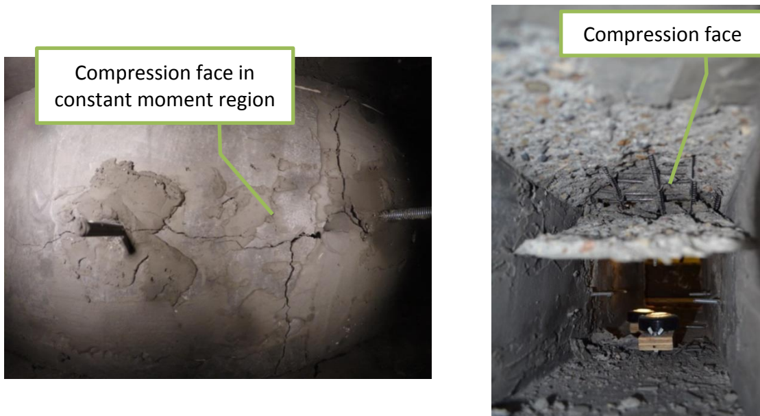
a) Prior to failure on the inner surface
