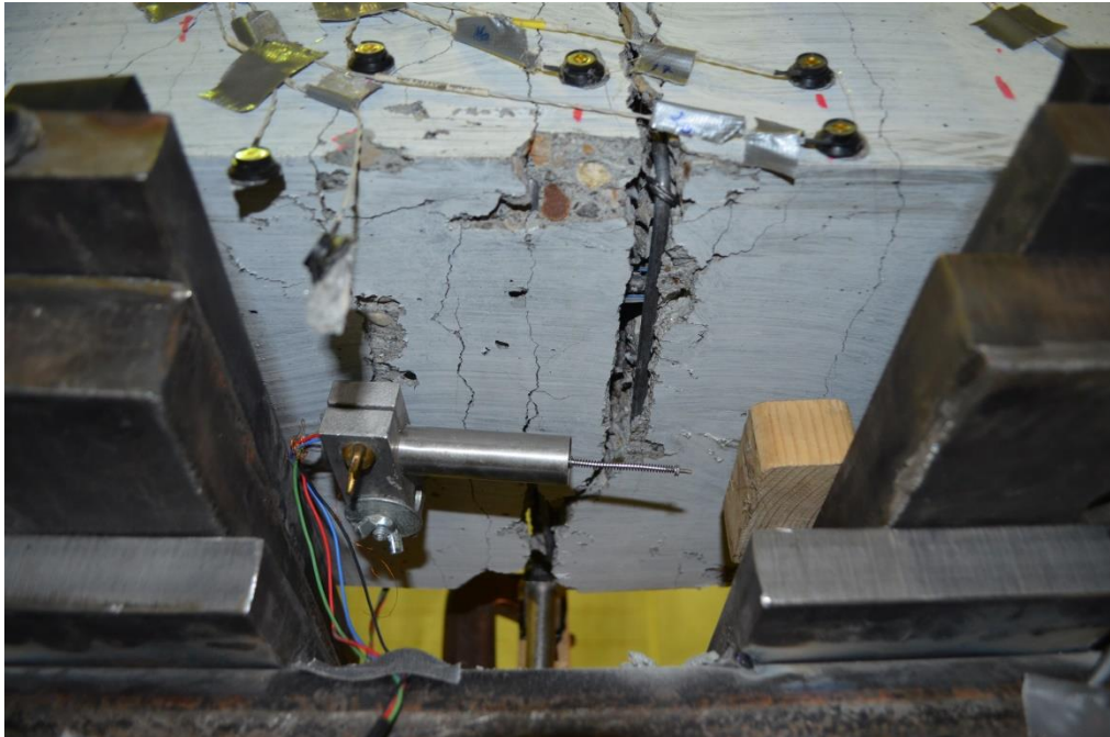
Figure 5-63: Specimen SS2-C Large Flexural Crack in Constant Moment Region after Failure
