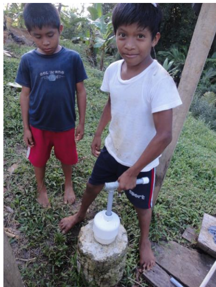
Figure D.4: Broken Handle of EMAS Pump at Attachment between Galvanized Iron “T” and PVC Half Inch Pipe La Ensenada
