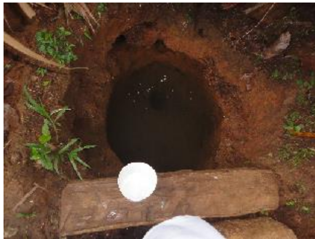
Figure D.2: Unimproved Drinking Water Source and Water Scoop Top View (which demonstrates soil and depth characteristics)
