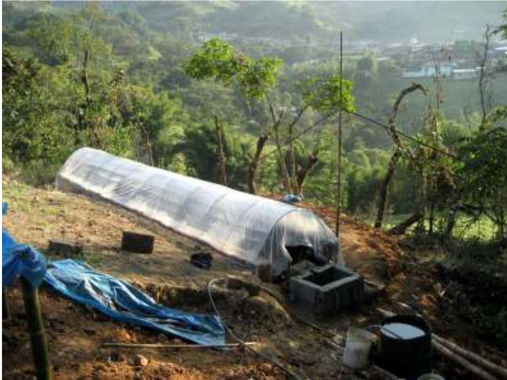
Figure 7: Photo of Taiwanese biodigester installed in Santo Domingo, Piura, Peru (photo from Christopher Galvin).
