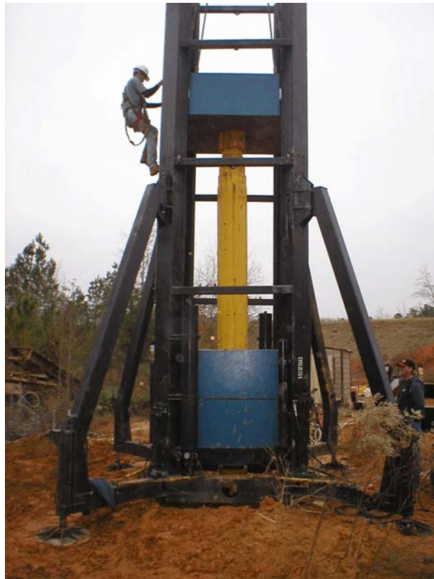
Figure 5.27 - 4MN static load test setup Auburn test site
