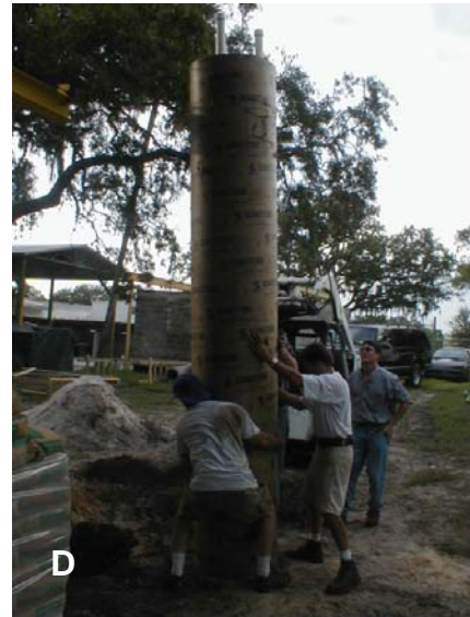
Figure 4.12 - Excavation and erection of test shafts for field trial #1, A - auger attached to skid steer, B - completed hole, C - setting Sonotube into hole, D - final erection of Sonotube
