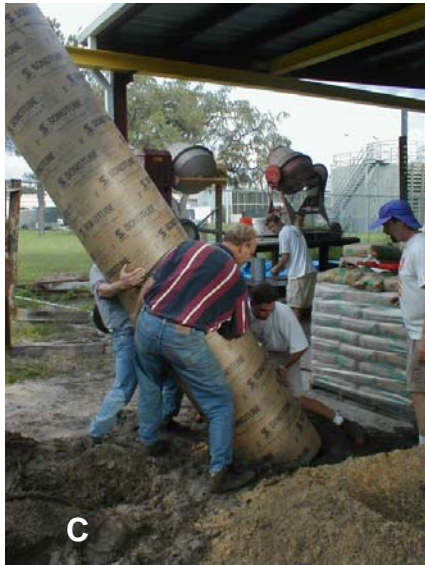
Figure 4.12 - Excavation and erection of test shafts for field trial #1, A - auger attached to skid steer, B - completed hole, C - setting Sonotube into hole, D - final erection of Sonotube
