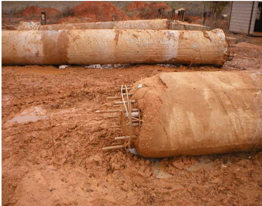
Figure 5.14 - Control shaft TS-4 and the CSL test results for TS-4 Auburn test site
