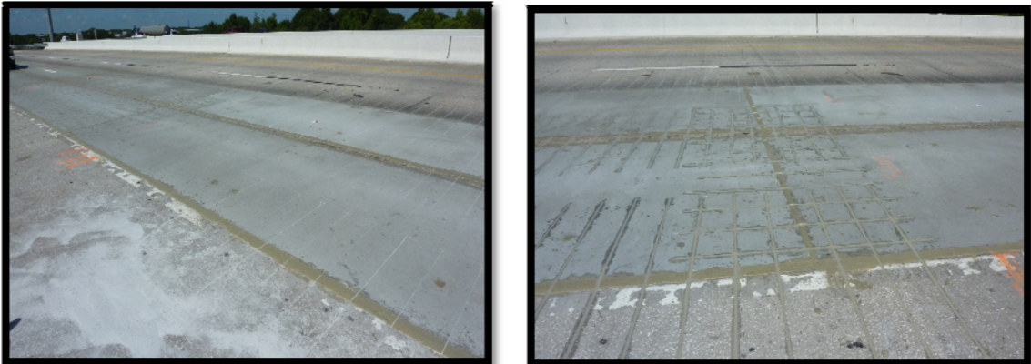
Figure 6.7 Completed Deck (Transverse and Longitudinal NSM CFRP Installation)
