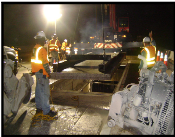
Figure 6.2 Existing Deck Cut and Removal Using Strong Back
