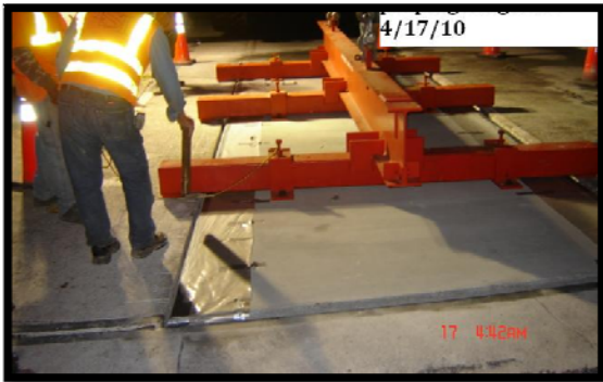
Figure 6.3 New Deck Suspension Using Strong Back
