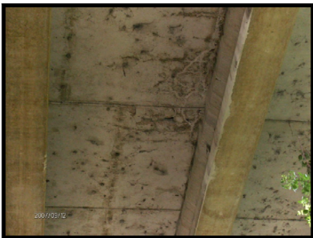
Figure 3.5 Bridge No. 100436, Span 4 Failure (Deck Underside)
