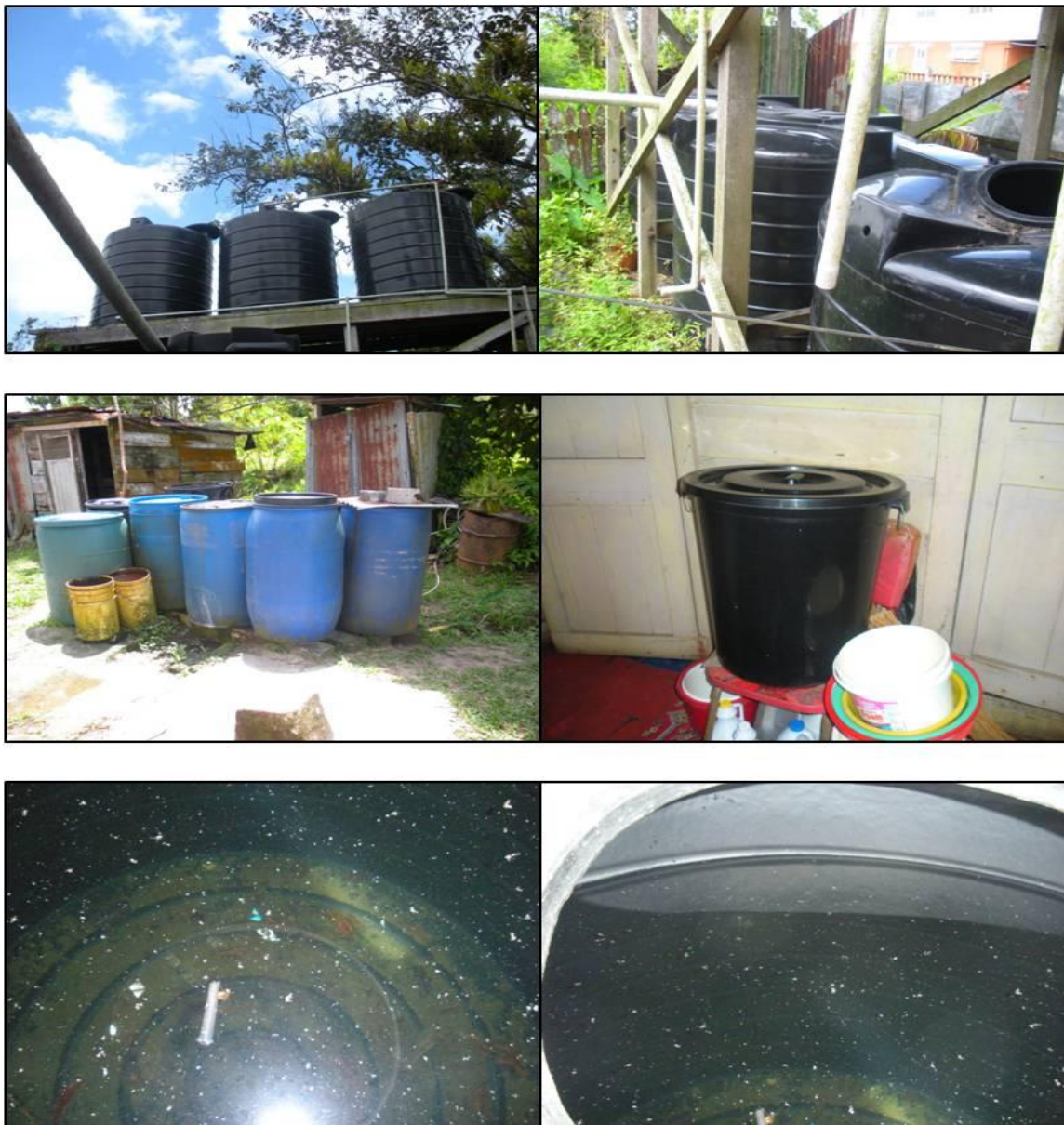
Figure D.7 Water storage devices and interior of water storage tank in Mocha-Arcadia Neighborhood Democratic Community, Guyana.
