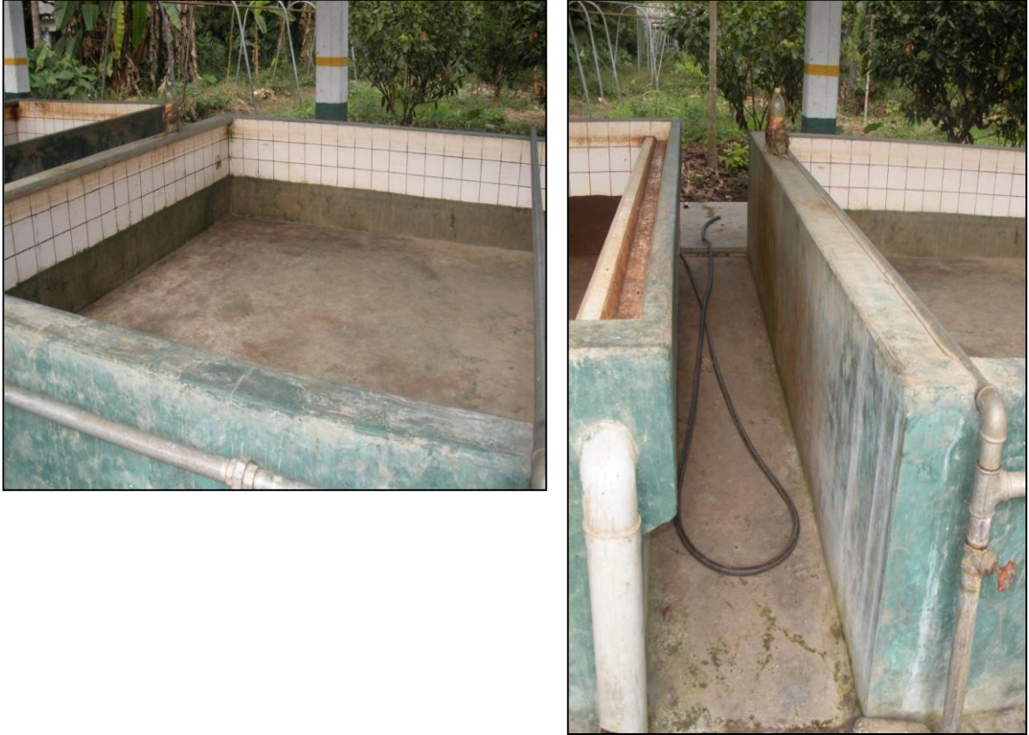
Figure D.14 Community pump and water source in Villa Litoral, Bolivia.
