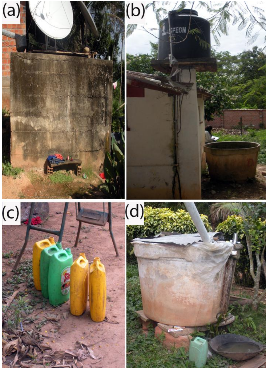
Figure 5.5 Representative water storage in Villa Litoral, Bolivia. (a) cement storage tank being filled with rainwater (roof runoff) and/or piped water from which water is collected at the base; (b) 400 gallon HDPE storage tank on the roof of a house that gets water from the main via a pump before it is piped to the house; (c) 5 gallon jerry cans used to collect water from standpipes; and (d) rain water collecting in a cement tank from which water is obtained from the base.
