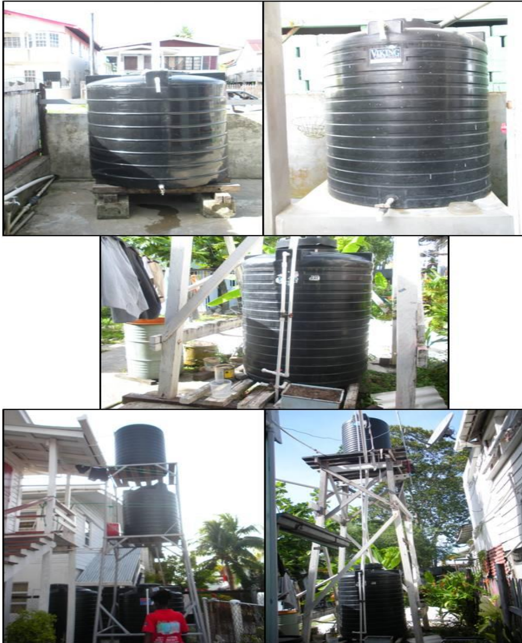
Figure D.10 Various water storage tank elevations seen in Georgetown, Guyana.
