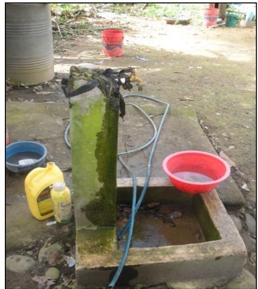
Figure D.13 Water sources in Villa Litoral, Bolivia. Left, dug well and right, stand pipe.
