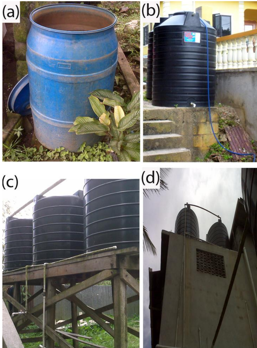
Figure 5.3 Representative water storage in Siparia, Trinidad and Tobago. (a) a 55 gallon HDPE storage drum (located next to a larger tank); (b) 400 gallon HDPE storage tanks being filled by a hose connected to a standpipe from which water is collected directly from the base; (c) 400 gallon HDPE storage tanks collecting rain water and water from the main from which water is obtained directly from the base and piped to the house; and (d) 400 gallon HDPE storage tank from which water is pumped from the ground to the rooftop tank prior to being piped to the house.
