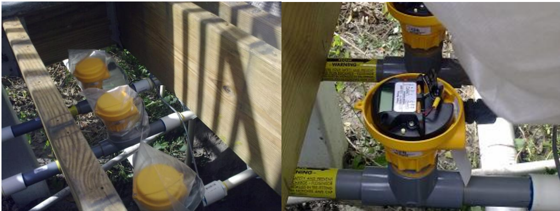
FIGURE 26: Installed water sensors under decking.
