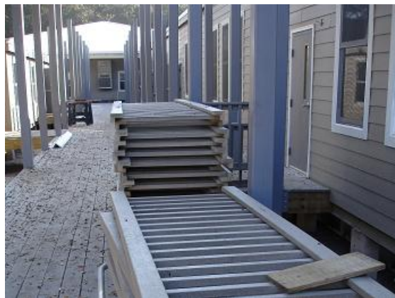
Decking made of recycled plastic
