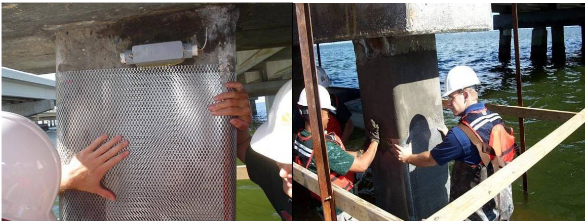
Figure 4.1 Sacrificial CP system using a mesh anode [4.7].
