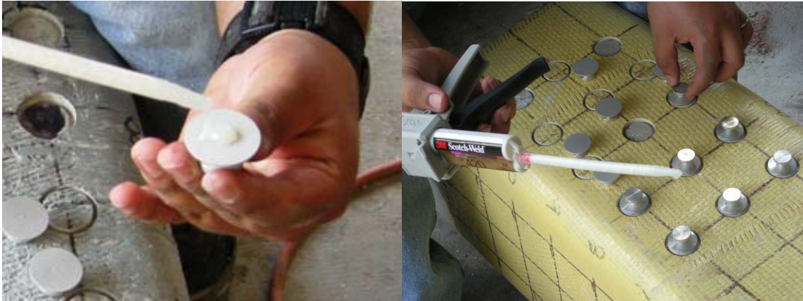
Figure 3.5 Installation of dollies for pullout test.
