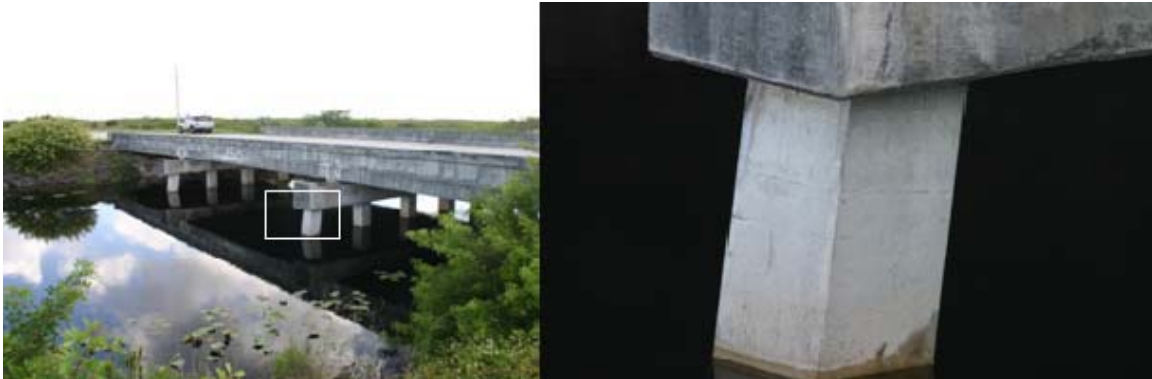
Figure 5.1 Bridge 1 used for evaluation of systems.
