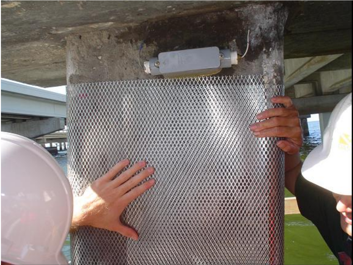
Figure 2.8 Expanded zinc anode in FRP pile repair.
