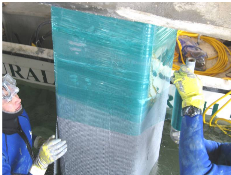
Figure 2.1 FRP repair kept in place by plastic shrink wrap.
