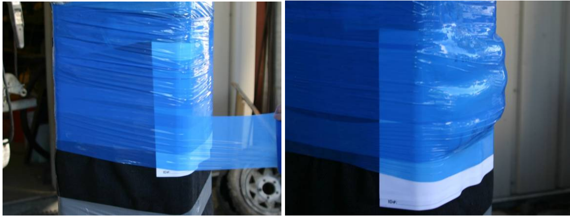
(a) (b) Figure 8.2 (a) Shrinkwrap on pile; (b) Shrinkwrap with bubble wrap.
