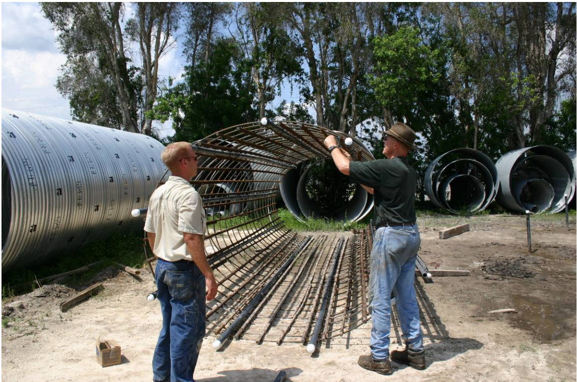
Figure 3-2: Voided Shaft Reinforcement Cage Instrumentation.
