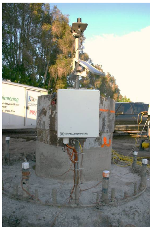
Figure 3-23: Remote Thermal Monitoring System for Voided Shaft.
