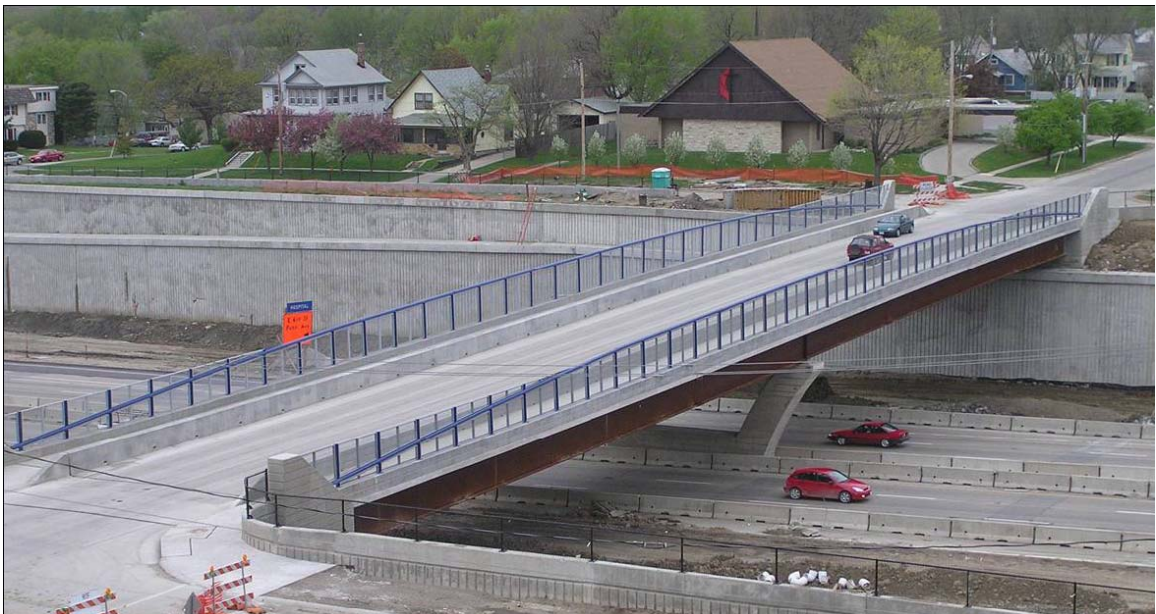
Figure 2-17: East 12 th Street Bridge, Des Moines, Iowa. (Hemphill, 2004)
