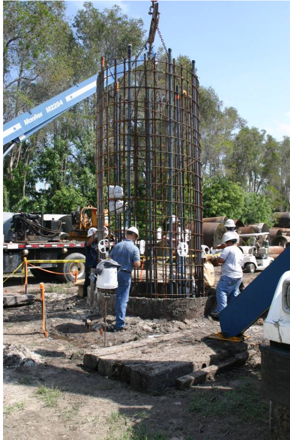
Figure 3-9: Placement of Reinforcement Cage for Voided Shaft.
