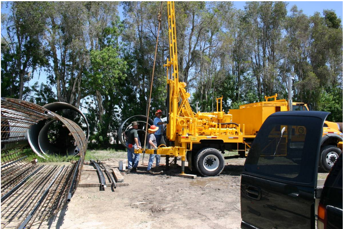
Figure 3-6: Voided Shaft Ground Monitoring Tube Installation.
