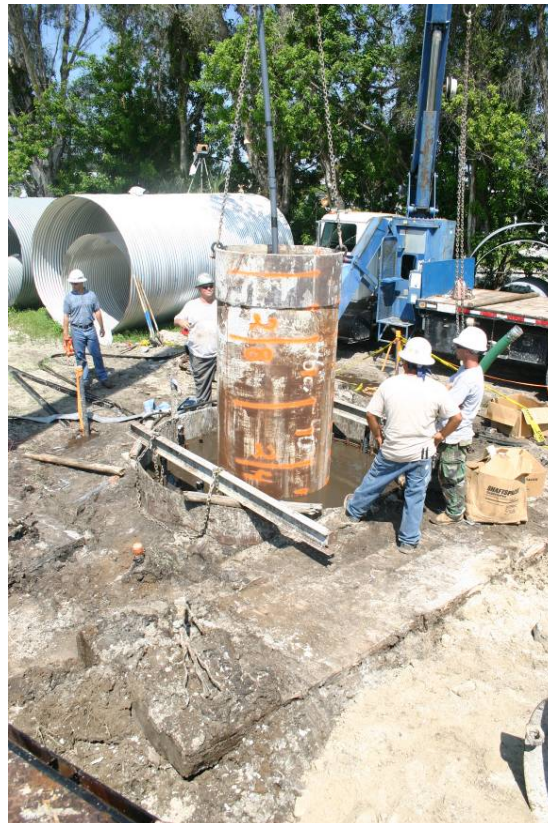
Figure 3-12: Placement of Central Casing for Voided Shaft.
