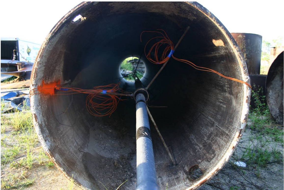
Figure 3-4: Voided Shaft Thermocouples Installed in Central Casing.
