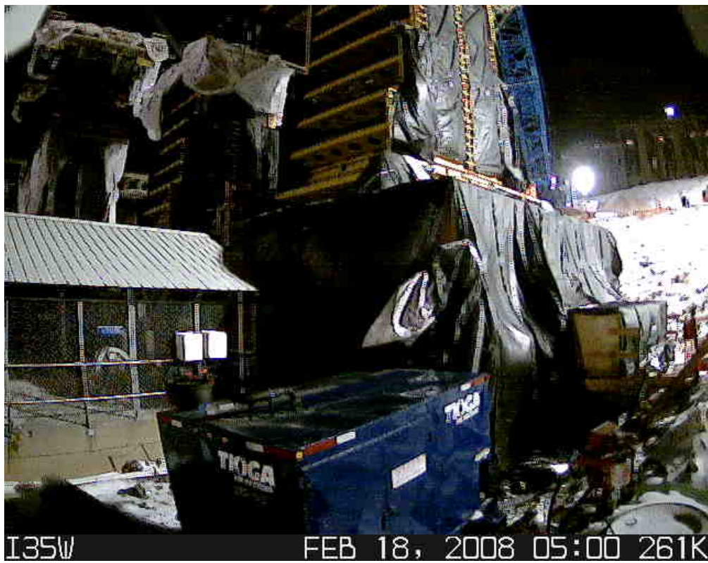
Figure 4-37: I-35W Bridge Exterior Column Lift 2 Formwork Placement.
