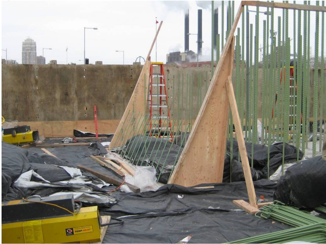
Figure 4-25: Reinforcement for 1 st Column Pour for I-35W Bridge Columns.
