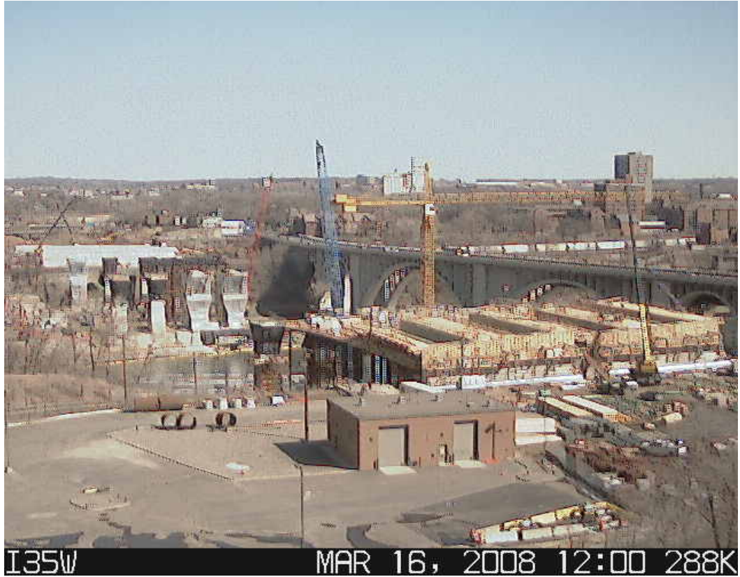
Figure 4-38: I-35W Bridge South Perspective CC640 Field Camera.
