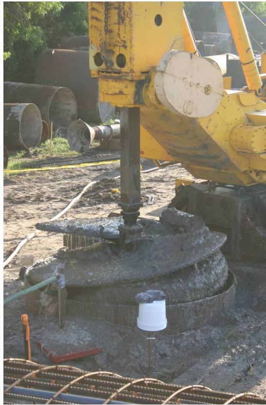
Figure 3-7: Excavation for Voided Shaft.
