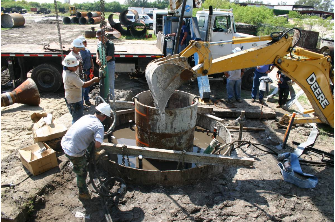
Figure 3-13: Voided Shaft Central Casing Stabilization.
