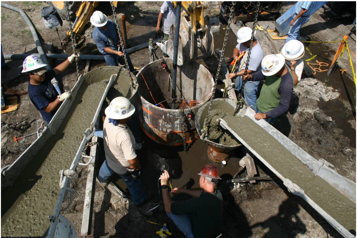
Figure 3-14: Double Tremie Concrete Placement.
