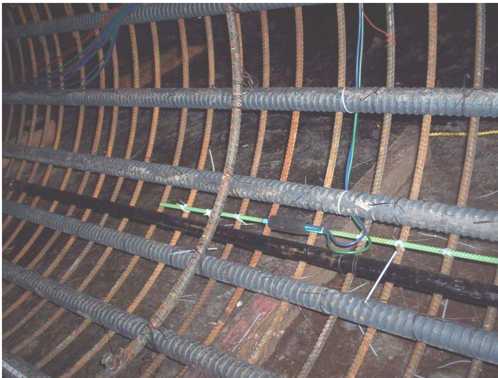
Figure 4-24: Coupled VW and RT Gages. (VW – Blue Cable, RT – Green Cable)
