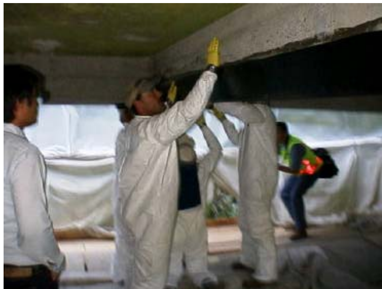
Figure 2-13: FRP Wrap Installation on Bridge Superstructure. (Udd et al., 1999)
