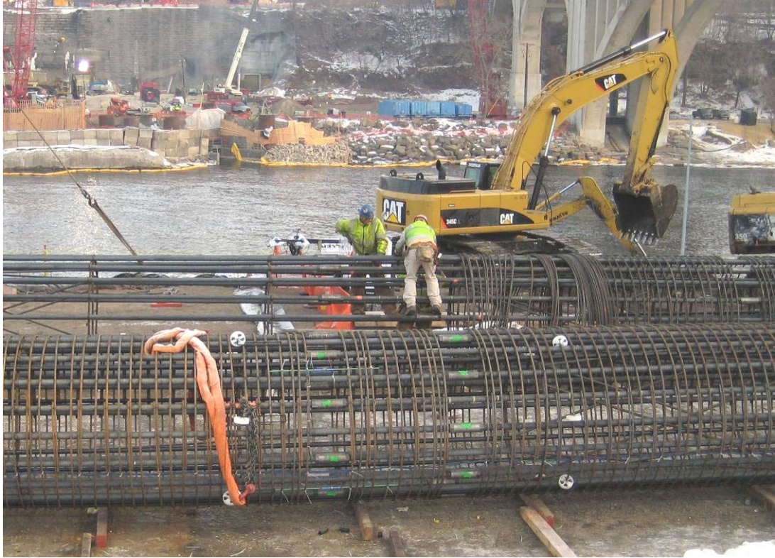
Figure 4-3: I-35W Bridge Shaft Reinforcement Cage Construction.
