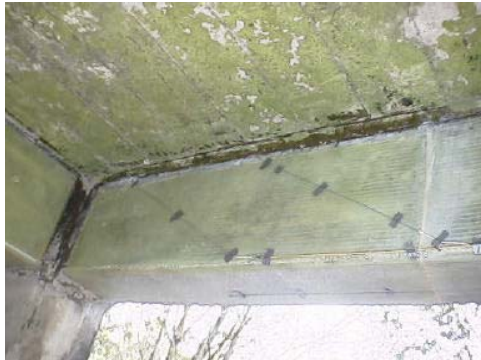
Figure 2-15: FOS Installation Above FRP Layers. (Udd et al., 1999)
