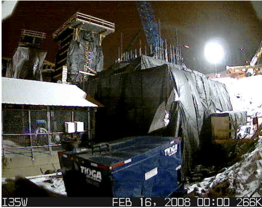
Figure 4-36: I-35W Bridge Interior Column Lift 2 Formwork Placement.
