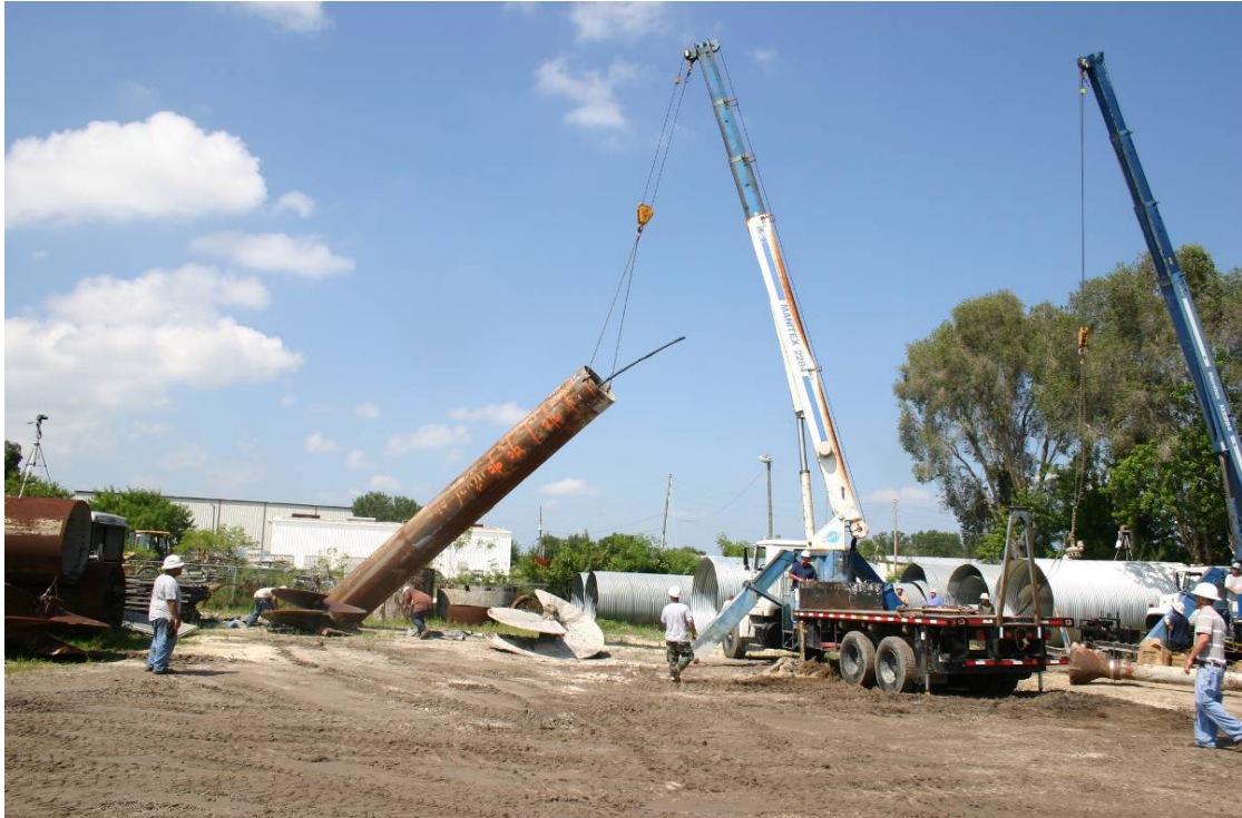
Figure 3-11: Picking of Central Casing for Voided Shaft.
