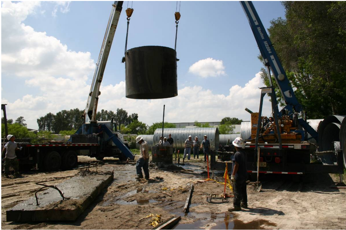
Figure 3-15: Outer Steel Casing Removal.
