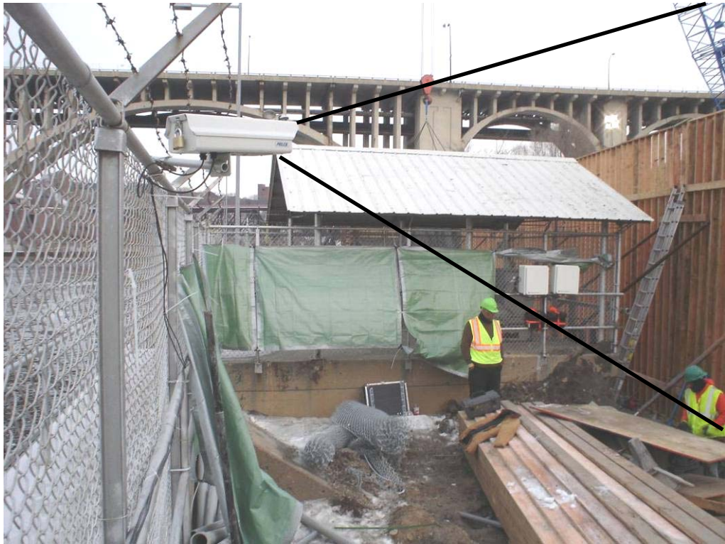
Figure 4-13: CC640 Jobsite Camera with Perspective Outlines.
