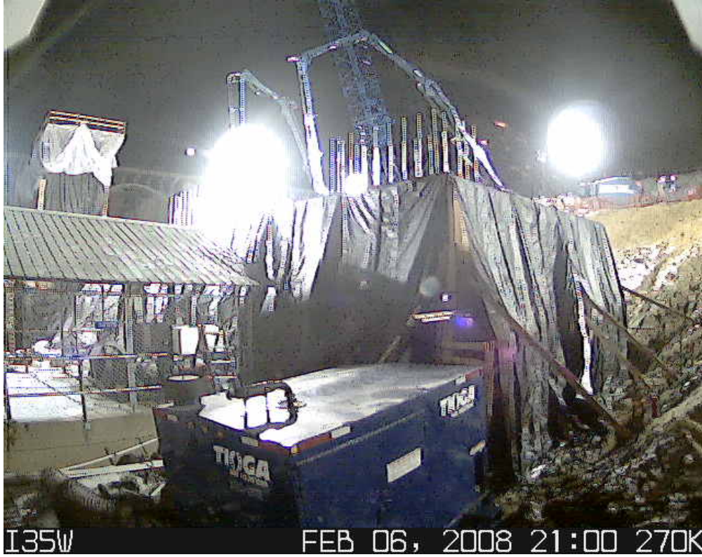
I35W FEB 06, 2008 21:00 270K Figure 4-34: I-35W Bridge Southbound Pier Footing Concrete Placement.
