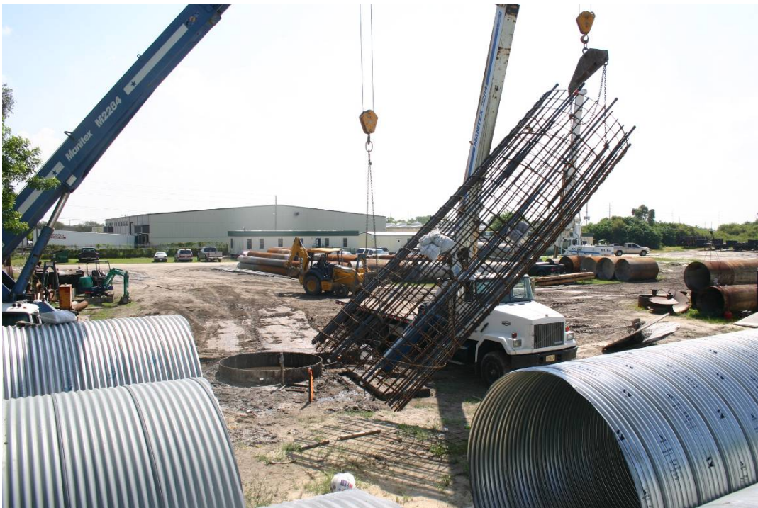
Figure 3-8: Picking of Reinforcement Cage for Voided Shaft.
