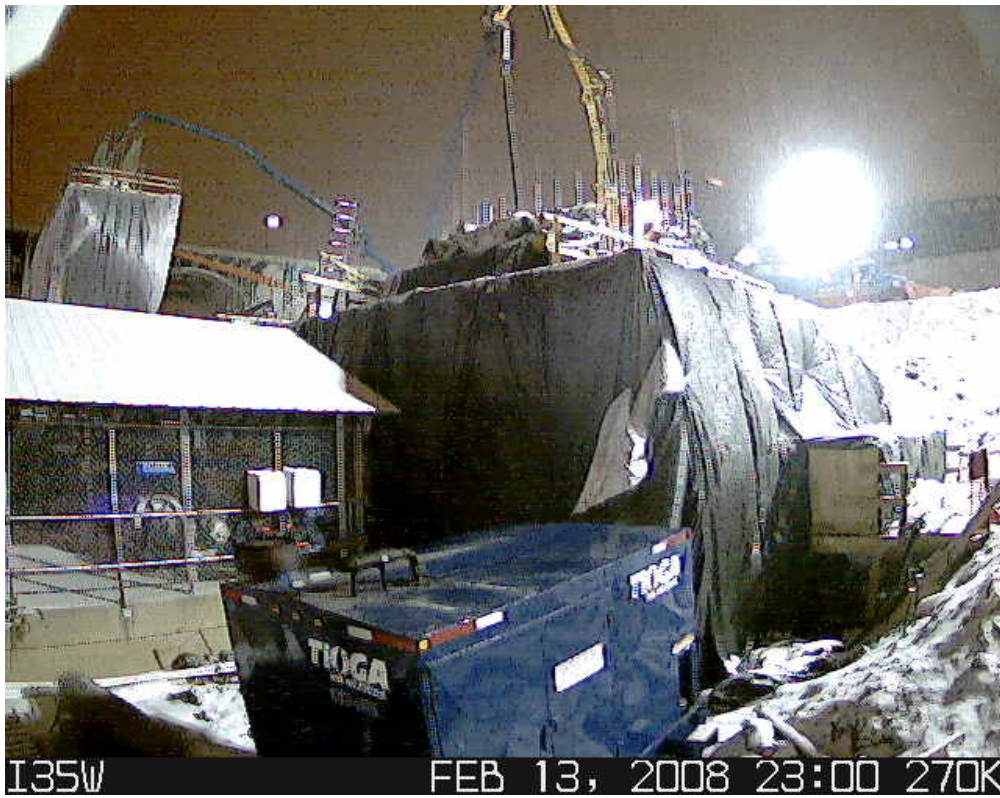
I35W FEB 13, 2008 23:00 270K Figure 4-35: I-35W Bridge Lift 1 Column Concrete Placement.
