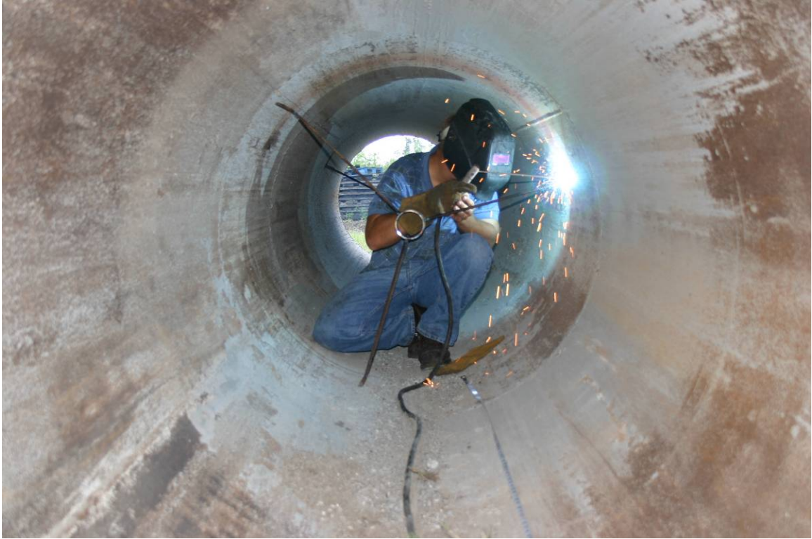
Figure 3-3: Voided Shaft Central Casing Center Tube Supports.
