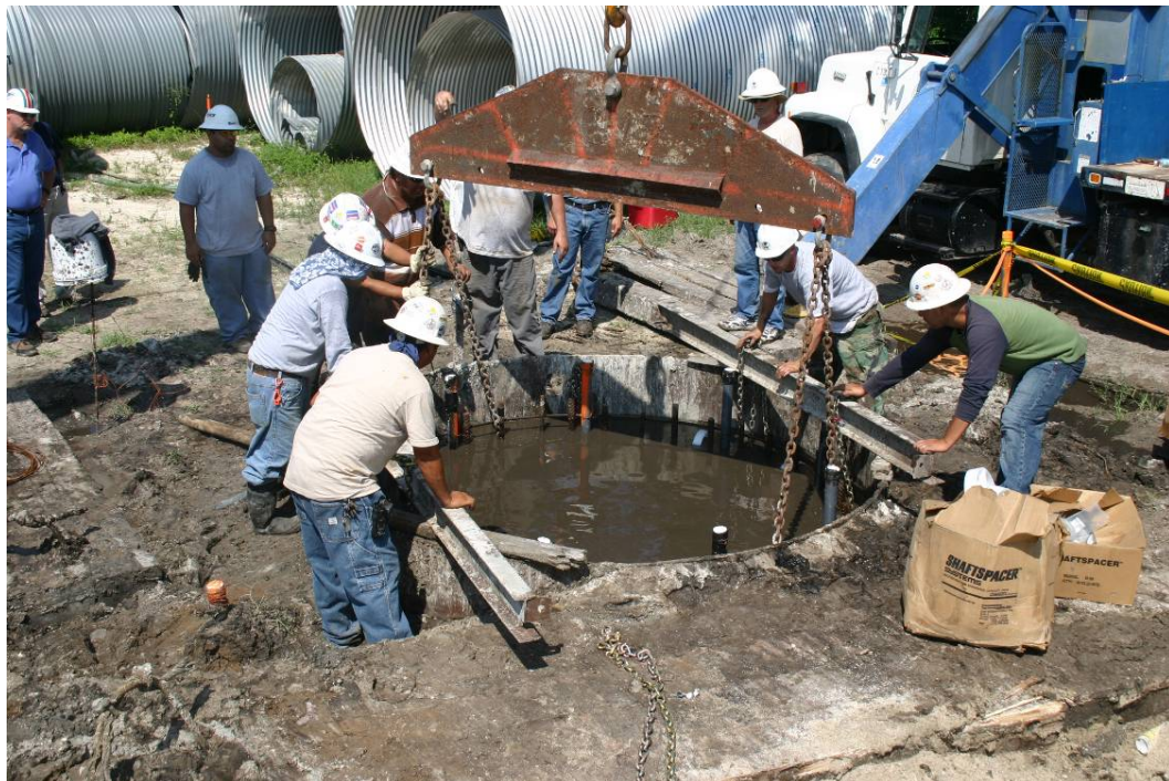
Figure 3-10: Hanging of Reinforcement Cage for Voided Shaft.
