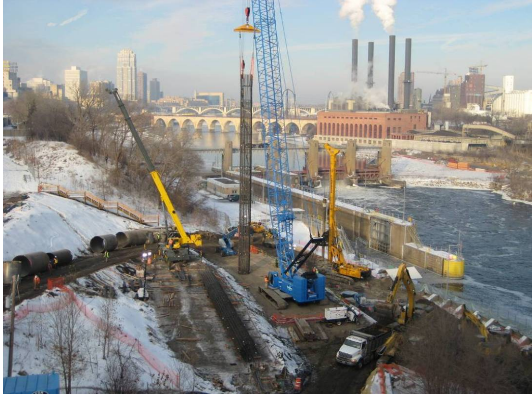
Figure 4-7: Placement of Reinforcement Cage for I-35W Bridge Shaft.
