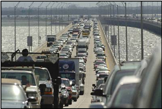
Figure 1 Florida Evacuation from Hurricane Charley in 2004
