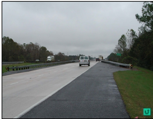
This photo displays how a shoulder lane may not provide continuous capacity, and lead to merging congestion for hurricane evacuation.
