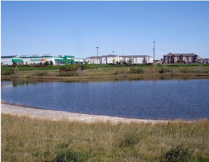
Figure 54: Typical Retention Pond
