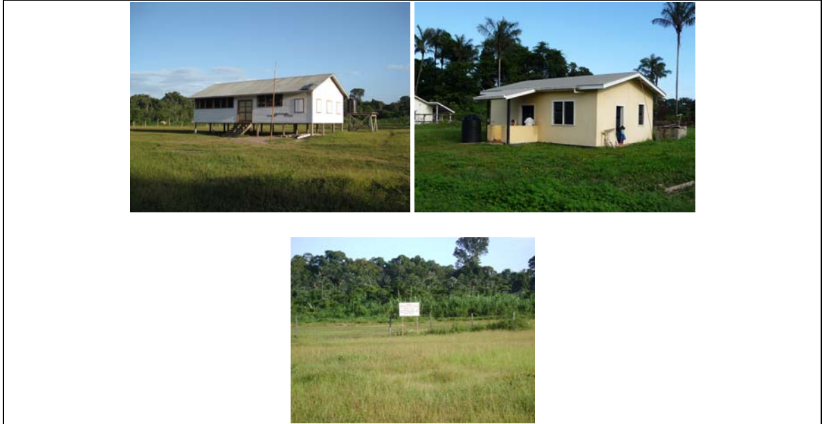
Figure C11 Fairview Village Primary School (top left), Health Center (top right) and air field (bottom).
