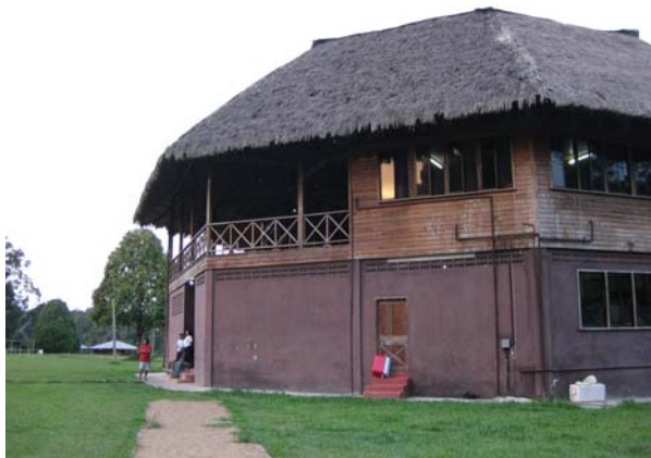
Figure C3 The main building with offices, kitchen and training facilities.
