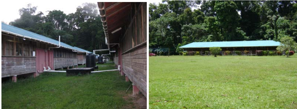
Figure C5 Views of the staff and researcher accommodations. Image on left shows rainwater harvesting technique from the roofs of the accommodations.
