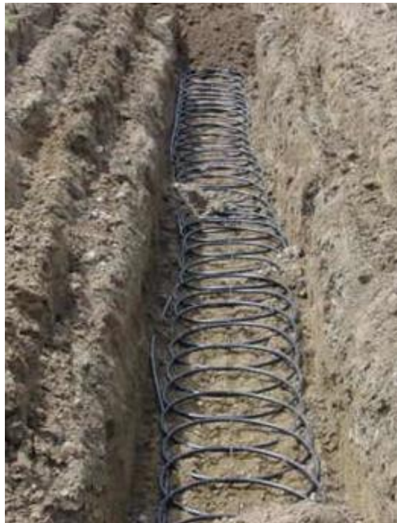
Figure 1.2: Geothermal Ground Loop
