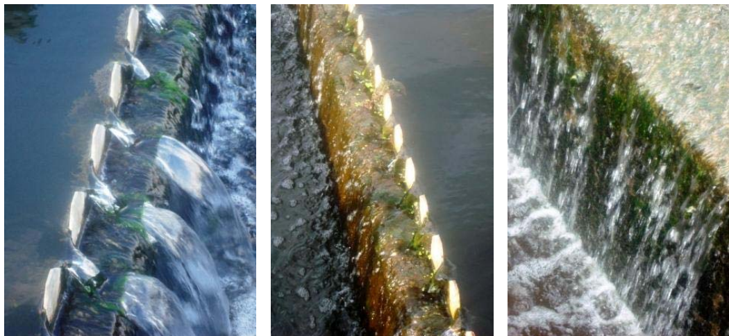
Figure 2.1: Native algae growing at different stages of treatment train at the Howard F. Curren AWTP. Post carbonaceous BOD removal clarifier (left), post nitrification clarifier (center) and denitrification filter (right).
