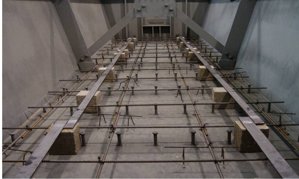
Figure 3.6 Placement of Bottom Concrete Slab
