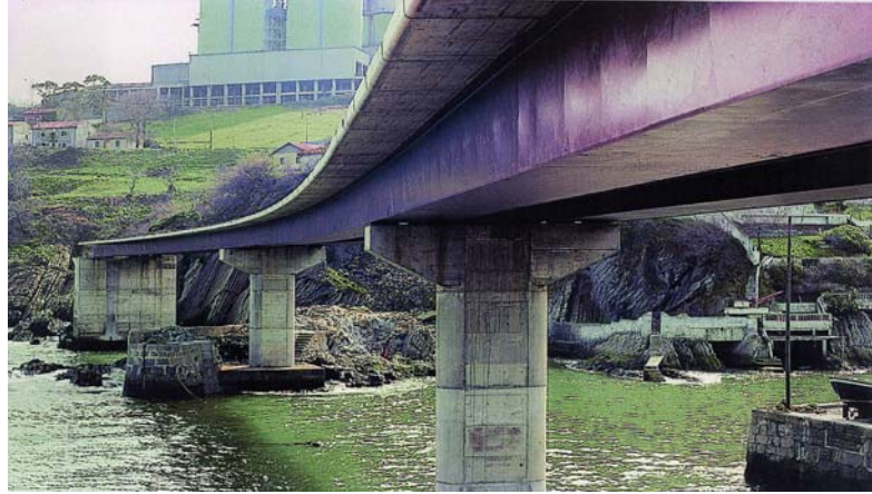
Figure 2.2 First Double Composite Bridge, Ciervana Bridge. (Courtesy J.M. Calzon)
