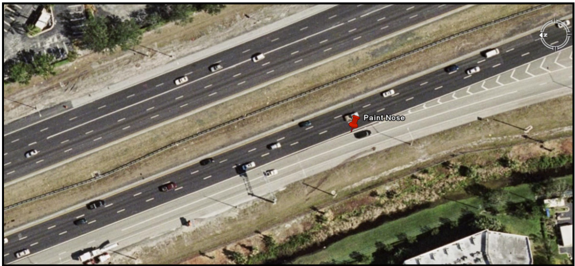
FIGURE 17. Site Picture for I-95 Southbound Exit 74
