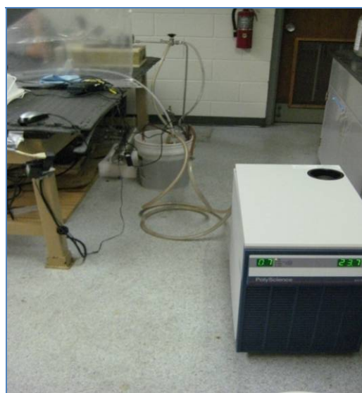
Polyscience Chiller and tubing
