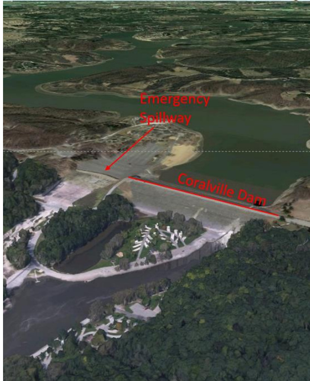
Figure 6.2 Close-up view of the Coralville Dam, including the main dam and the emergency spillway.
