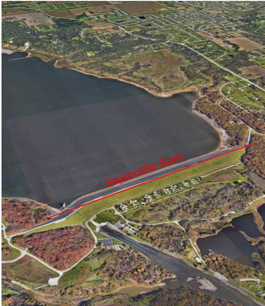
Figure 6.15 Close-up view of the Saylorville Dam.
