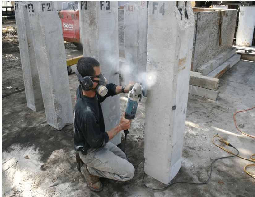
Figure 3.3 Grinding Corners of the Pile
