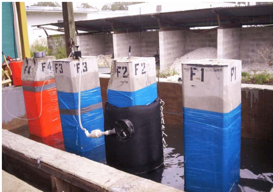
Figure 3.18 Pressure Bagged Fyfe and Air Logistics Piles
