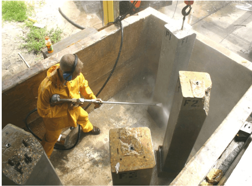
Figure 3.5 Pressure Washing Piles in Tank
