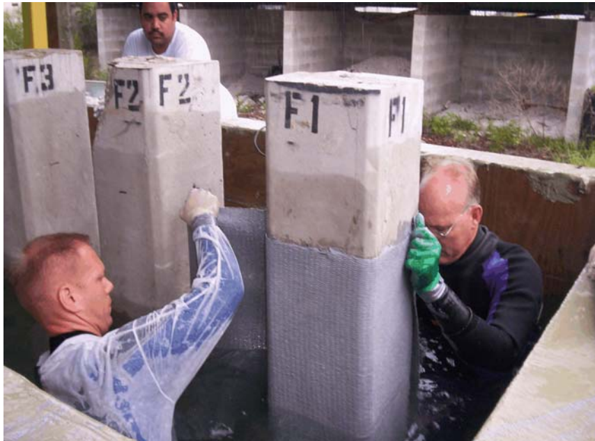
Figure 3.7 Applying Transverse FRP Layer to Fyfe Pile
