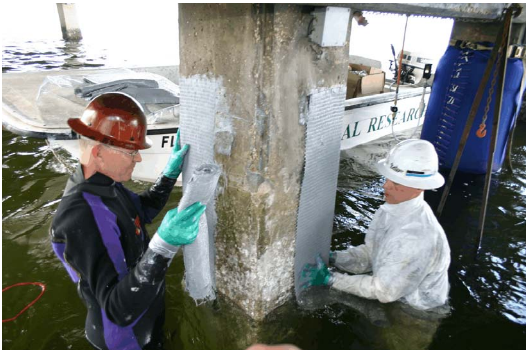
Figure 1.2 FRP Wrapping of Corrosion Damaged Bridge Pile
