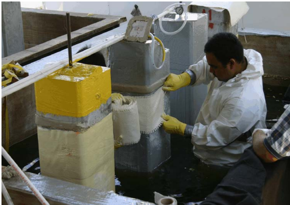
Figure 3.10 Applying Transverse FRP Layer to Fyfe Pile
