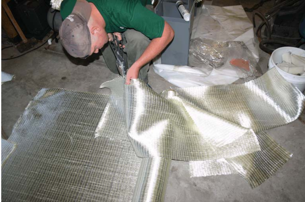
Figure 1.1 Cutting Dry Sheets of FRP Prior to Placement
