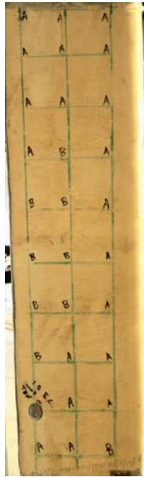
Figure C.109 Pile A4 Face D Color Photo
