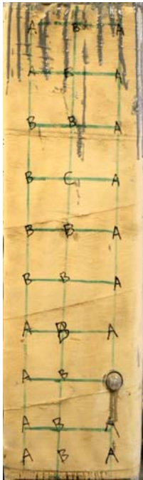
Figure C.77 Pile A1 Face D Color Photo
