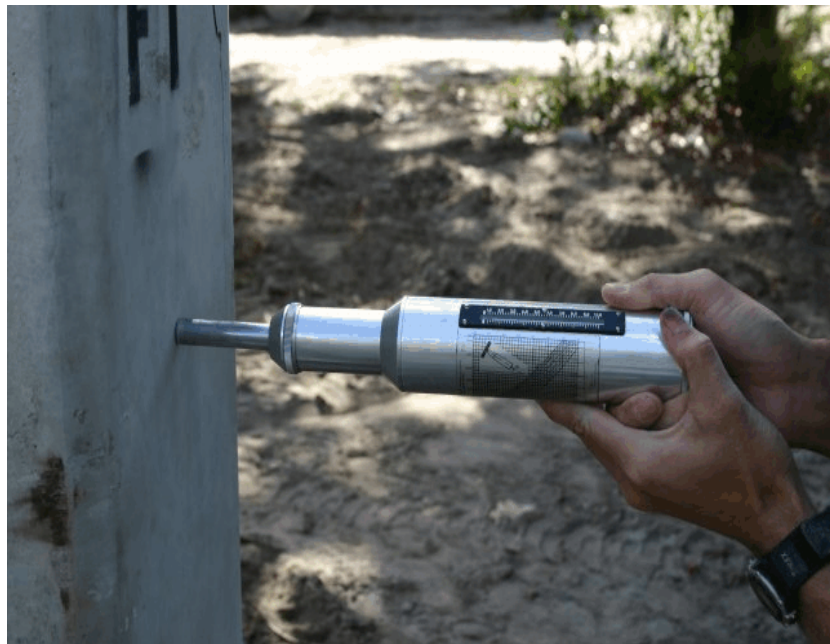
Figure 3.4 Testing Compressive Strength with Schmidt Hammer
