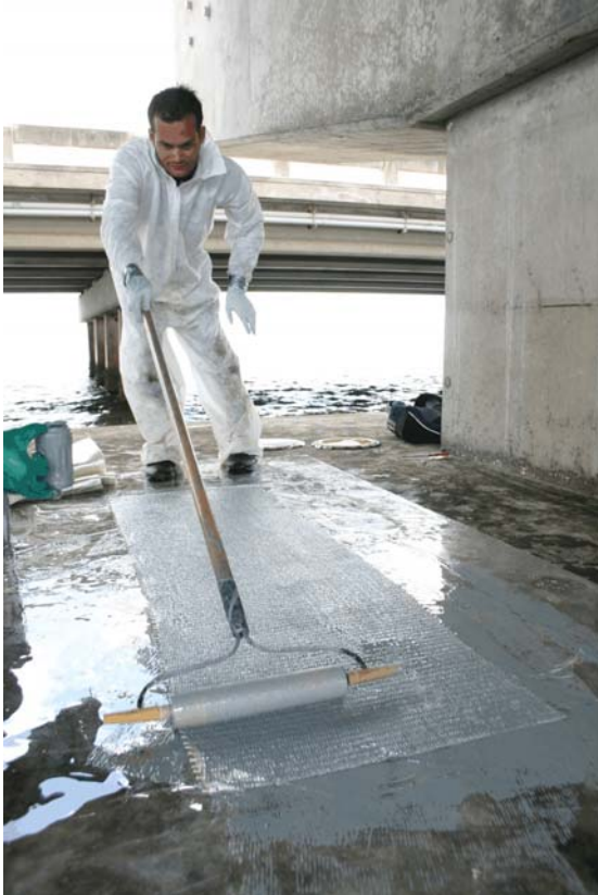
Figure 2.1 Field Saturation of FRP Fibers with Curing Compound
