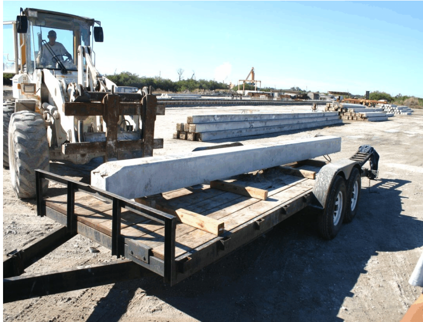
Figure 3.1 Loading Piles Onto Trailer at Henderson Prestress Yard
