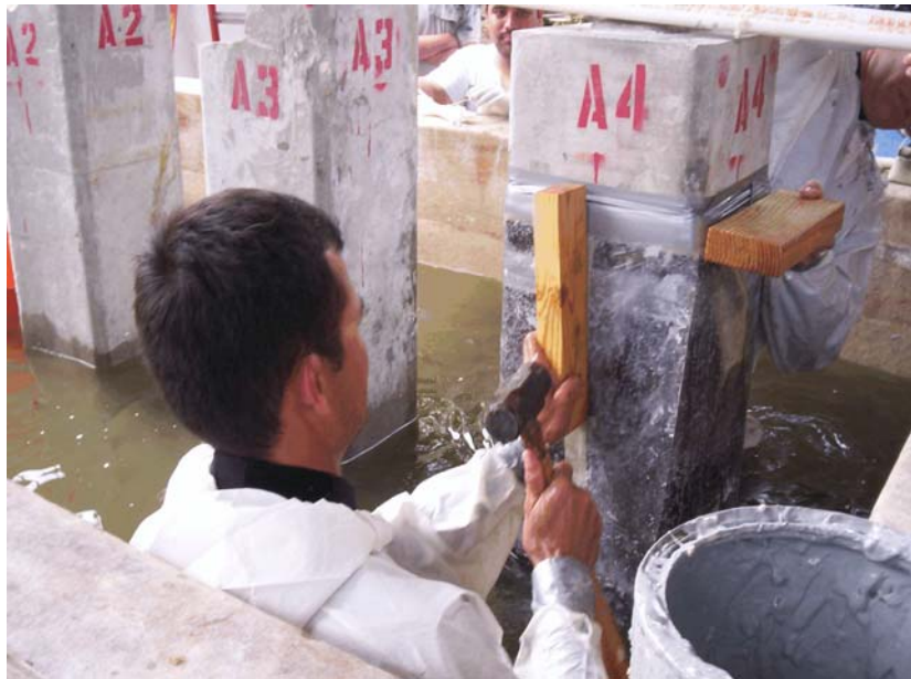
Figure 3.11 Hammering Down Layers for Vacuum System
