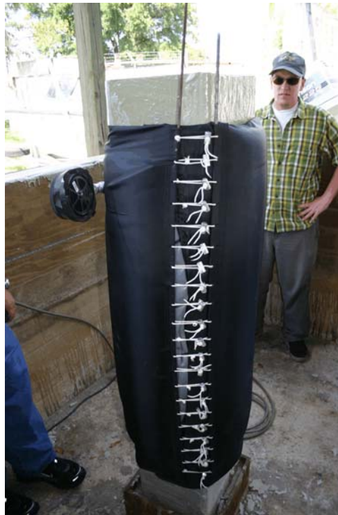
Figure 3.17 Pressure Bag Shown on Pile, Inflated, with Vertical Toggle System
