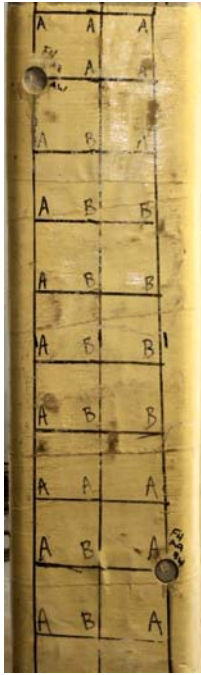
Figure C.60 Pile F4 Face C Color Photo
