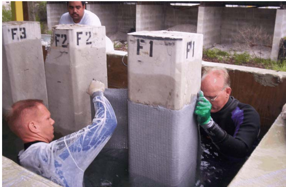
Figure 2.3 FRP Wrapping of Pile During Laboratory Study
