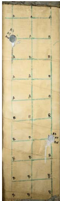
Figure C.92 Pile A3 Face C Color Photo
