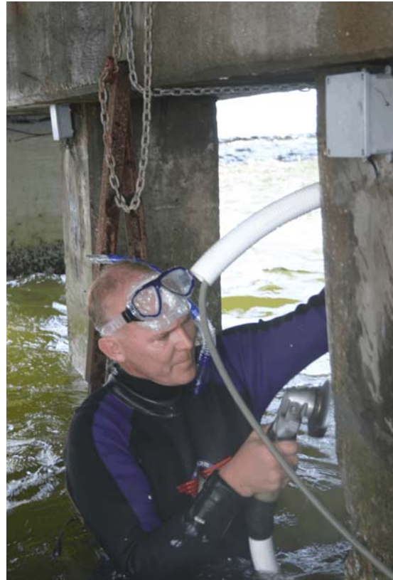
Figure 2.2 Grinding Edges of Pile to Ease FRP Application
