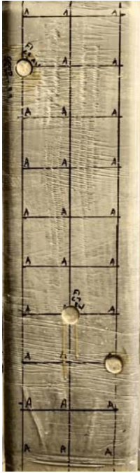
Figure C.10 Pile F1 Face C Color Photo
