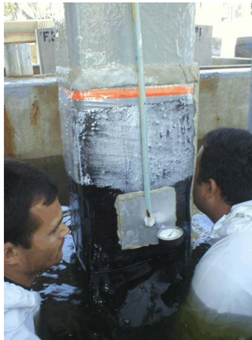
Figure 3.14 Vacuum Seal Installed, Awaiting Final Shrink Wrap Layer
