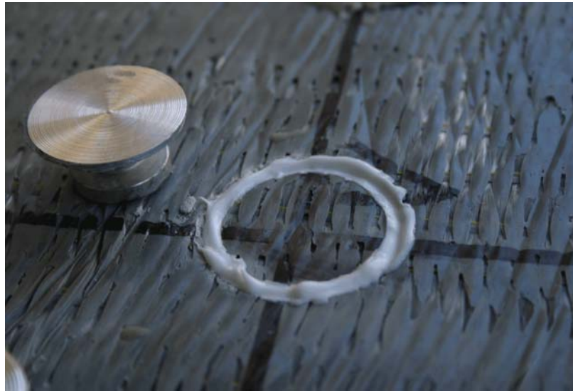
Figure 4.3 Pull-off Test Area
