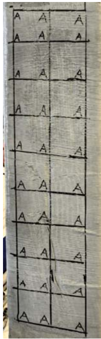
Figure C.41 Pile F3 Face B Color Photo
