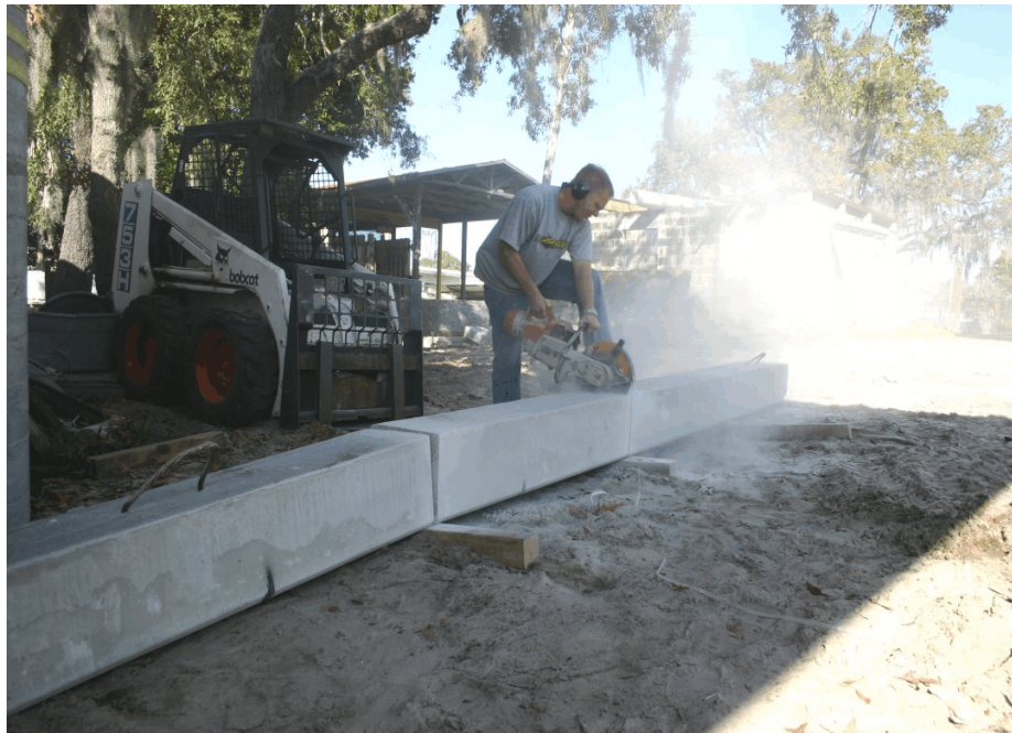
Figure 3.2 Cutting Piles Into 5 ft Sections
