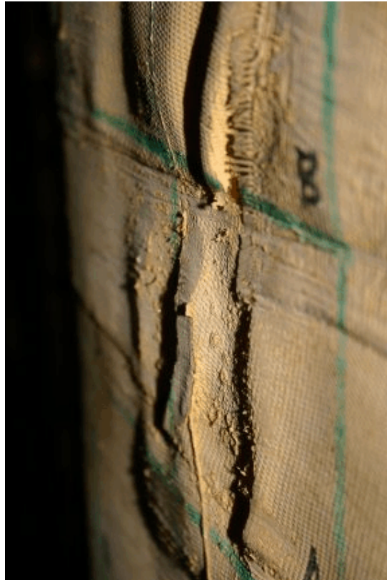
Figure 5.1 Wrinkles on Air Logistics Piles
