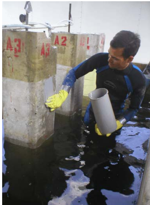
Figure 3.8 Applying Resin Pre-coat to Air Logistics Piles
