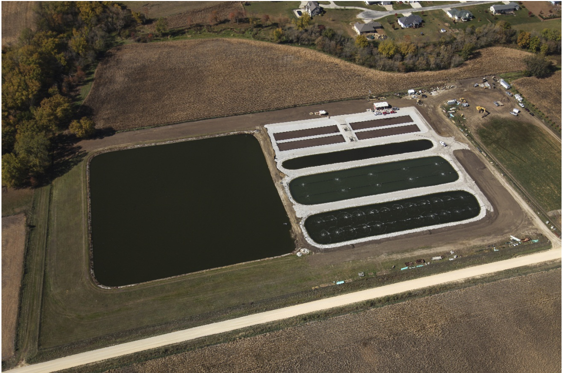
Figure B.1 Aerial view of the Walker, IA lagoon-SAGR WRRF.
