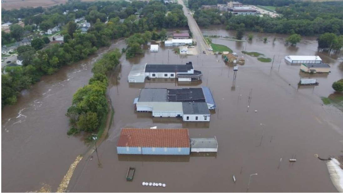
Figure 3. Drone photo of flooding in downtown Manchester during September 2016
