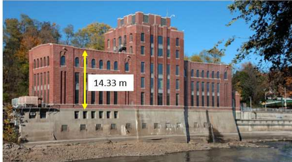
Figure 4.2 IIHR - Hydrosience & Engineering building where the snowfall experiment was conducted
