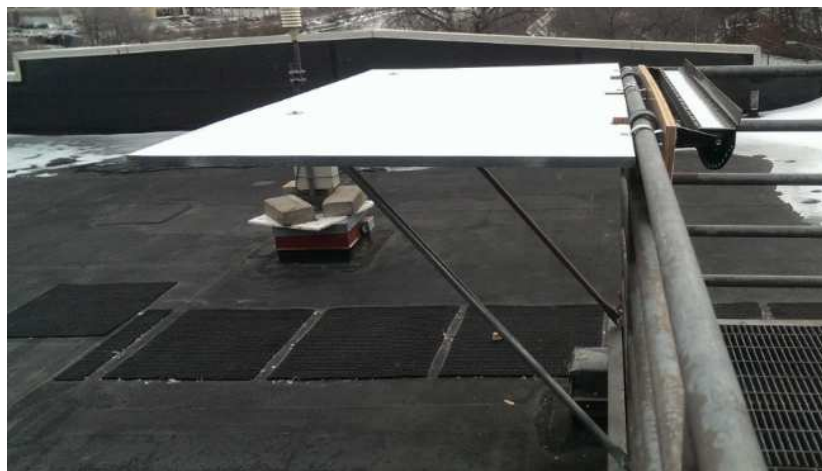
Figure 4.4 Snow measurement board used to measure snow accumulation as part of the rooftop experiment
