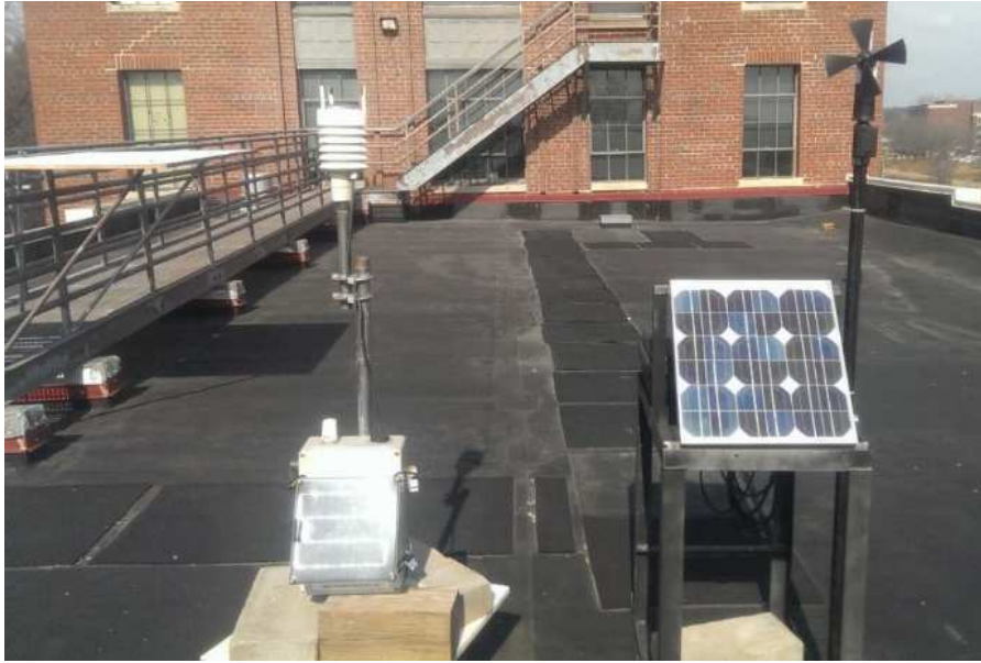
Figure 4.11 Setting of the Vaisala & Youngs anemometers on the roof of IIHR building
