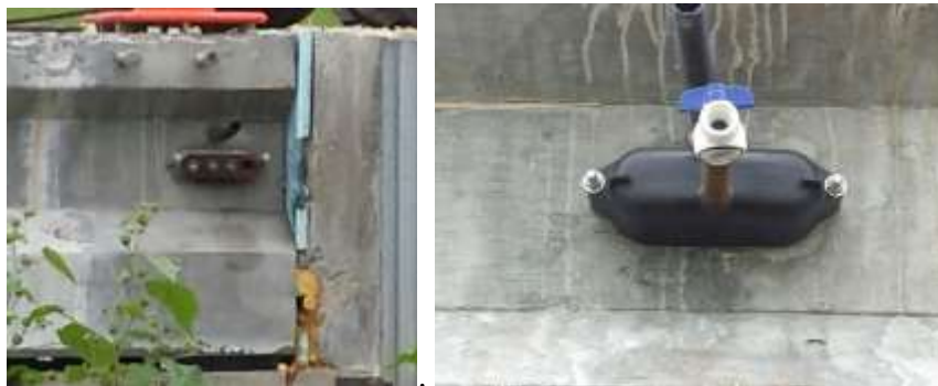
Figure 5-40 Post Tensioned Transverse Strands with/without Cap
