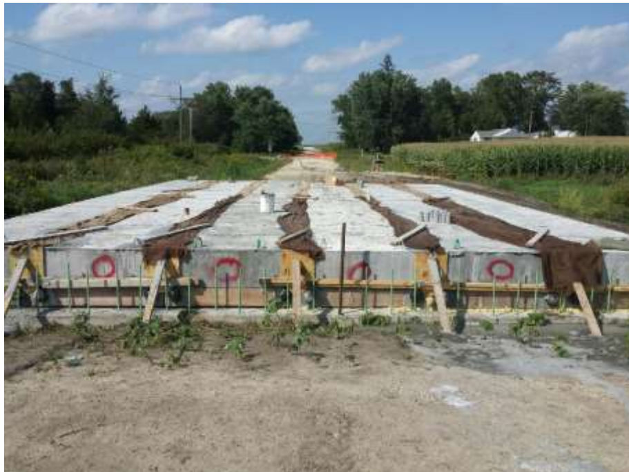
Figure 5-36 Burlaps Put on Each Joint
