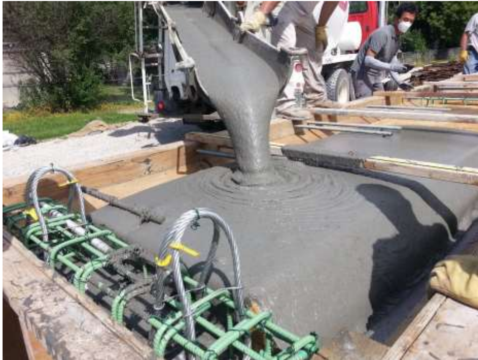
Figure 5-18 K-UHPC Pouring for Sixth Girder
