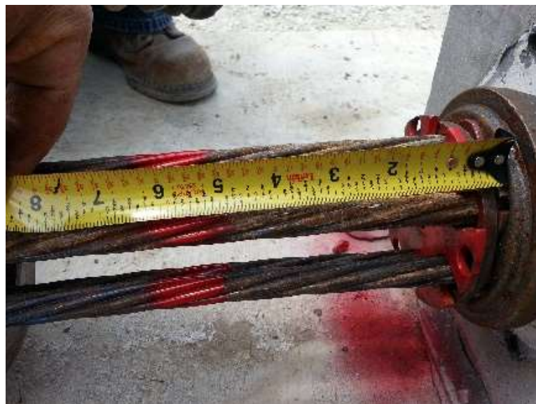
Figure 5-14 Elongation of Post-tensioned Strands
