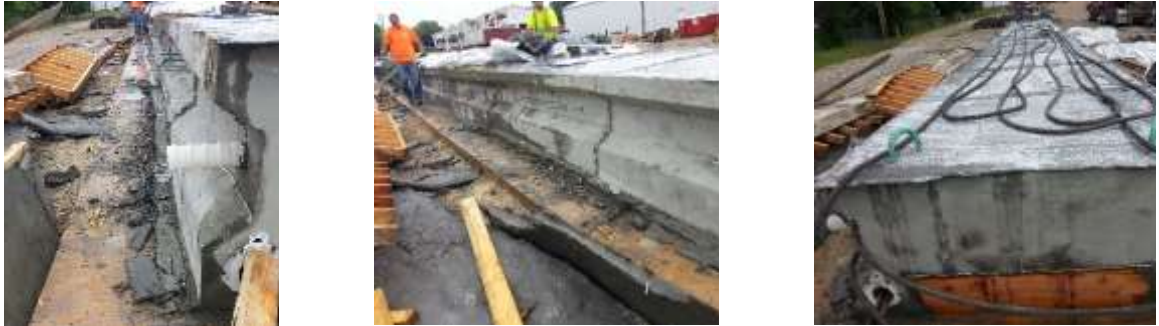
Figure 5-12 Completed Second Girder
