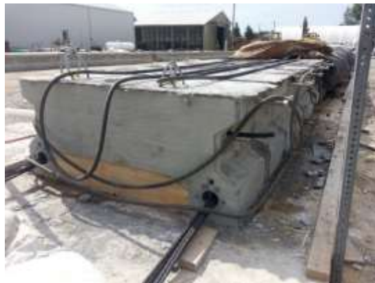
Figure 5-19 Steam Curing on Sixth Girder
