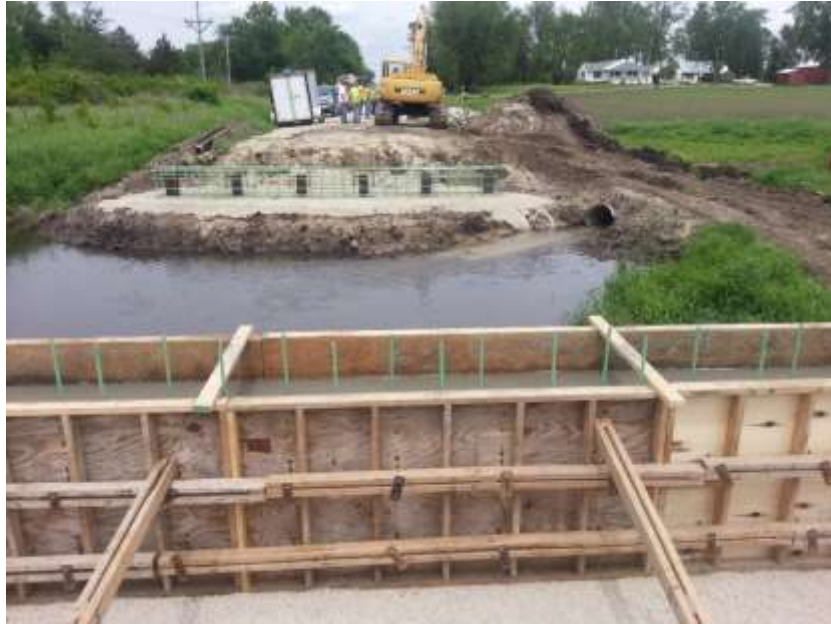
Figure 4-2 Construction of Substructure of Hawkeye UHPC Bridge
