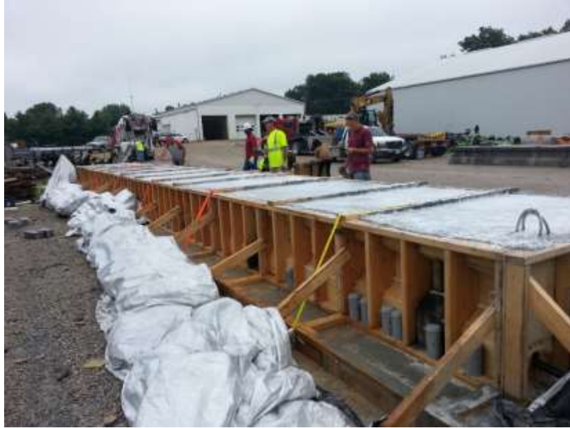
Figure 5-16 Casted Third Girder with Improved Support on Form
