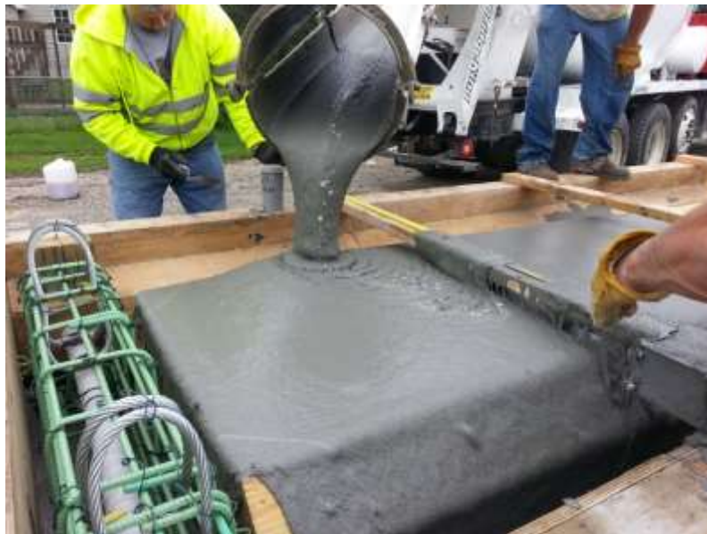
Figure 5-15 K-UHPC Pouring for Third Girder
