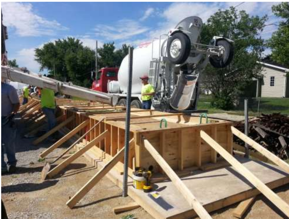
Figure 5-2 Orientation of Two Trucks during Pouring
