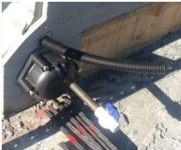
Figure 5-22 Cap with Attached Grout Opening
