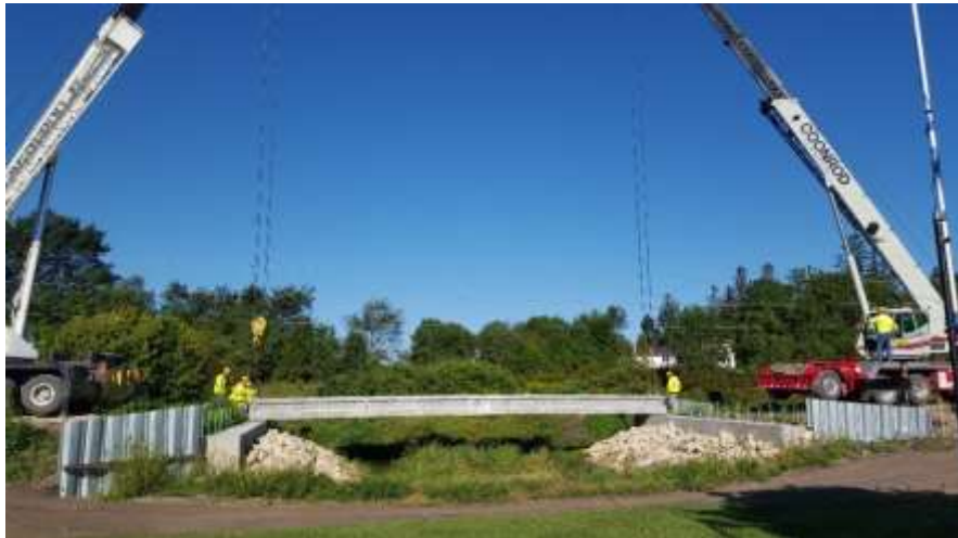
Figure 5-27 Bridge Installation
