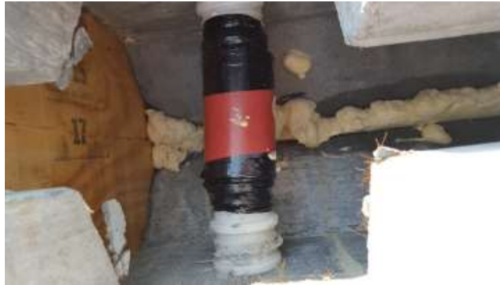
Figure 5-31 Filled Gap and Connected Post-tensioning Duct
