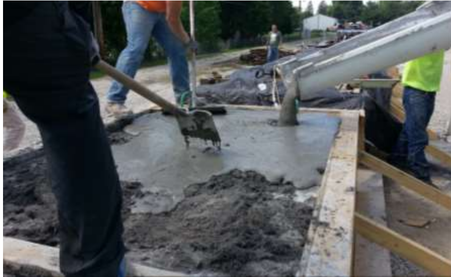
Figure 5-6 Additional 2CY of K-UHPC Pouring
