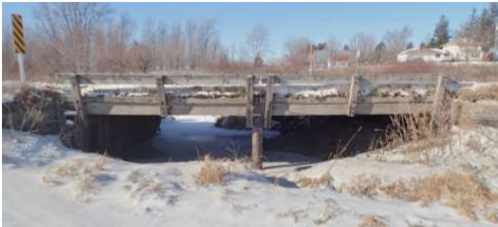
Figure 2-4 Old Multi-Beam Timber Bridge
