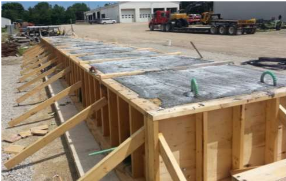
Figure 5-4 Casted First Girder
