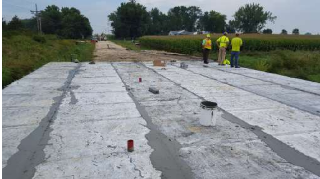
Figure 5-35 Filled Joints with K-UHPC
