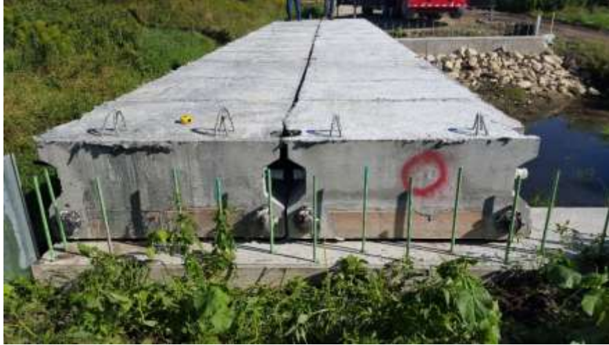
Figure 5-28 Two Installed Girders
