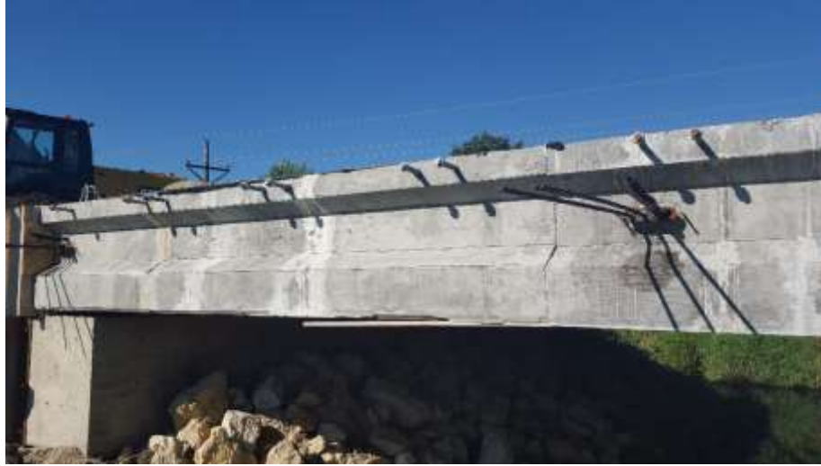
Figure 5-39 Post-tensioned Transverse Strands
