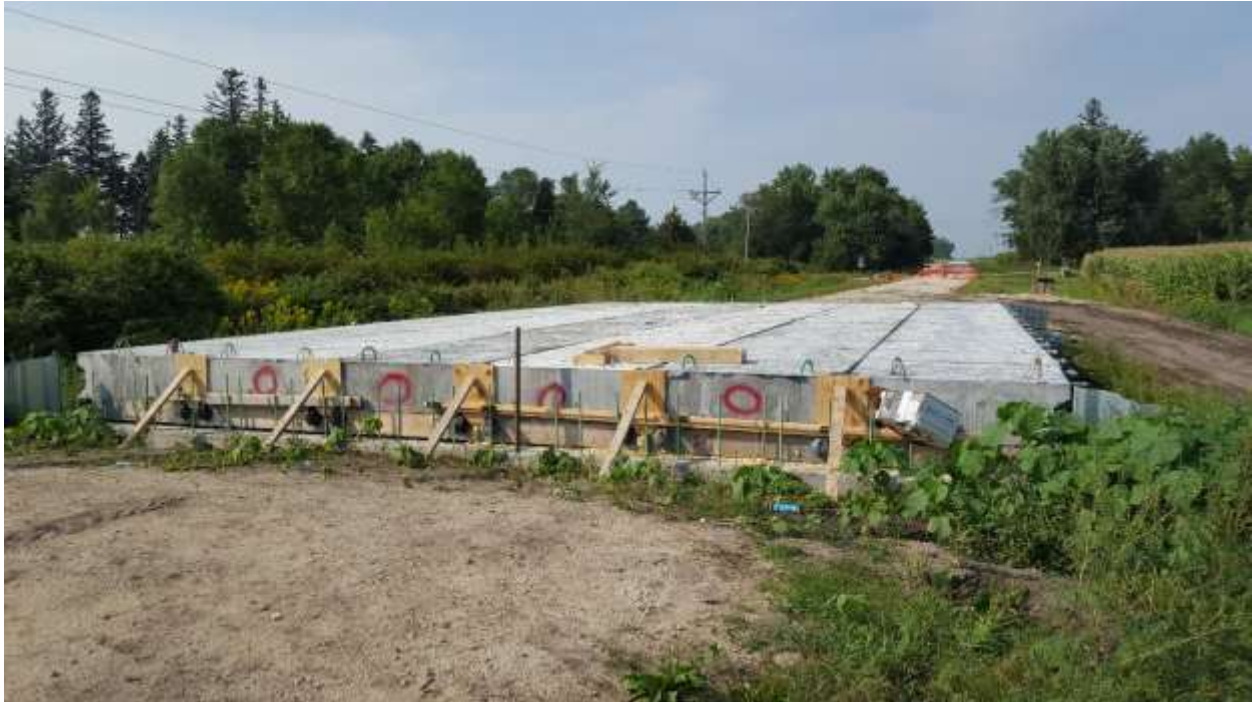
Figure 5-33 Formwork for Joint Filling
