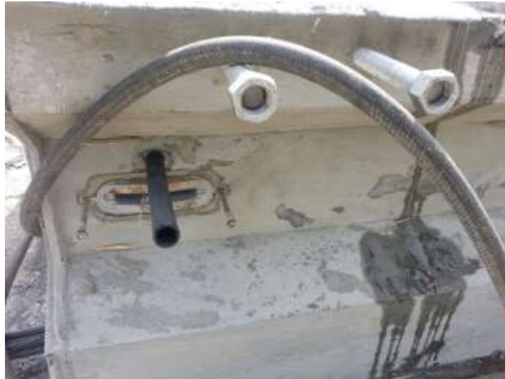
Figure 5-20 Opening for Transverse Post-tensioning Strands
