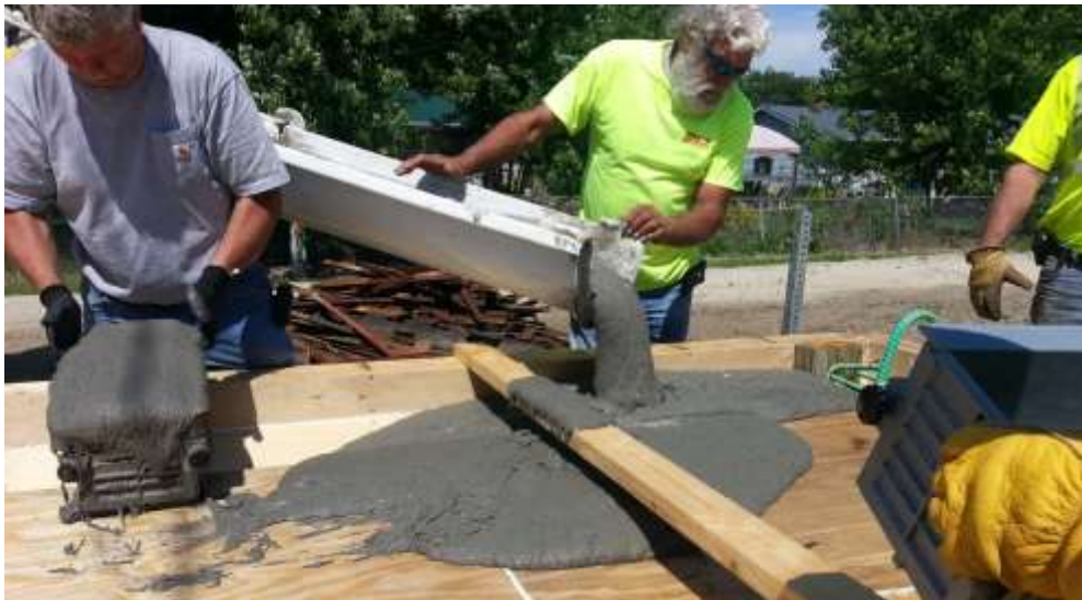
Figure 5-3 First Girder Pouring
