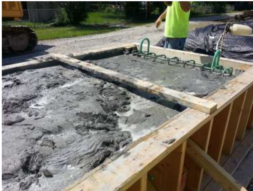
Figure 5-5 Incomplete Second Girder
