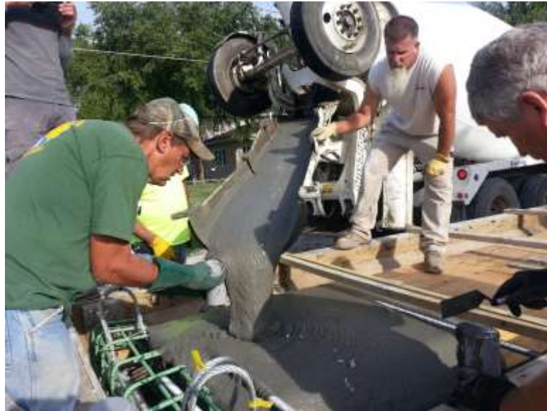
Figure 5-17 K-UHPC Pouring for Fifth Girder
