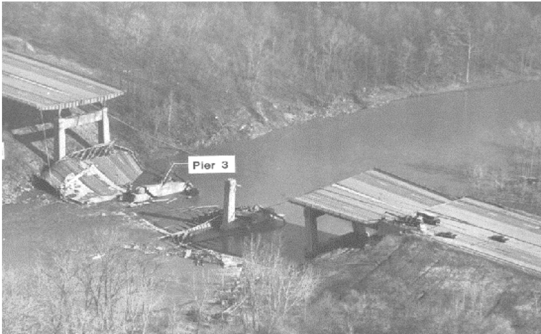
Figure 1.1: I-90 over Schoharie Creek (Courtesy of Northwestern University Infrastructure Technology Institute [6])
