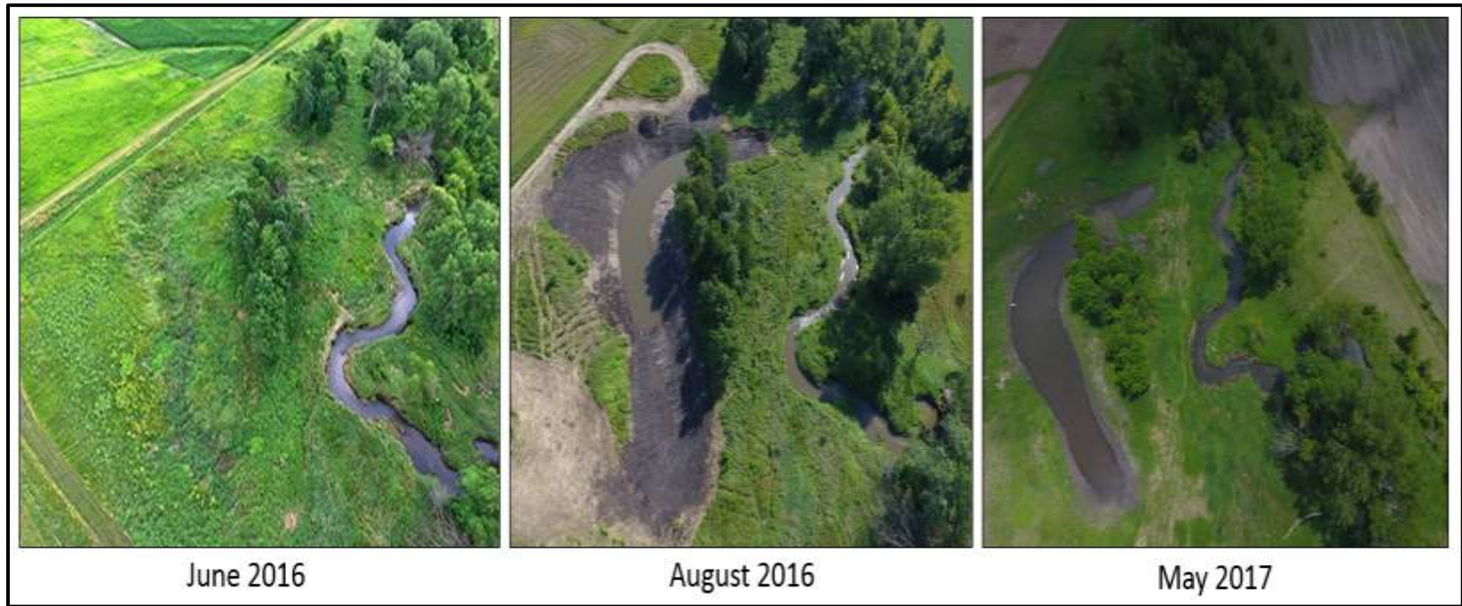
Figure 3.2. The transition of a restored oxbow from the initial "scar" in June, 2016 (a), post construction in August 2016 (b), to the completed project with established vegetation along the perimeter of the oxbow in May, 2017 (c).
