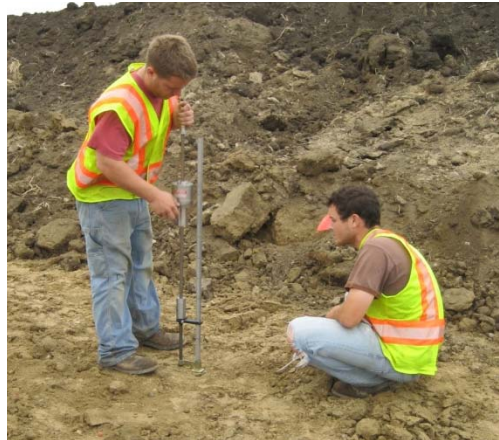
Figure 62: Strength determination using dynamic cone penetrometer
