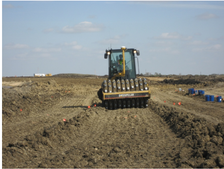
Figure 76: TH60 strip compaction
