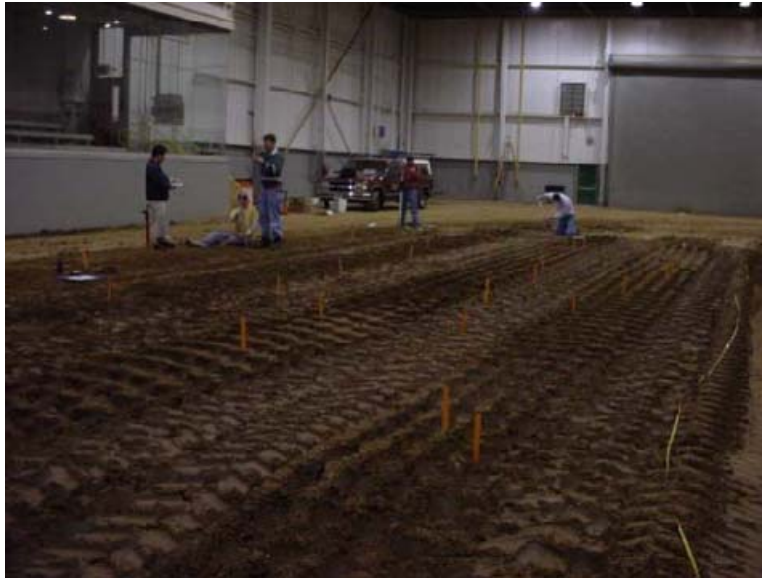
Figure 69: Test strips A through D after compaction
