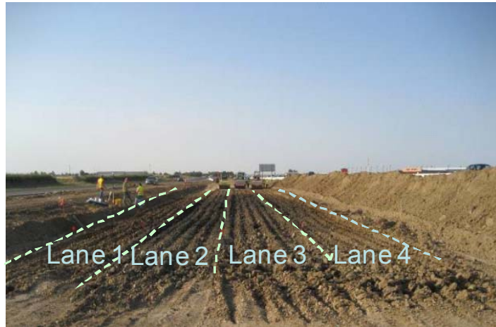
Figure 81: Picture of subgrade lanes prepared for compaction and testing - Colorado
