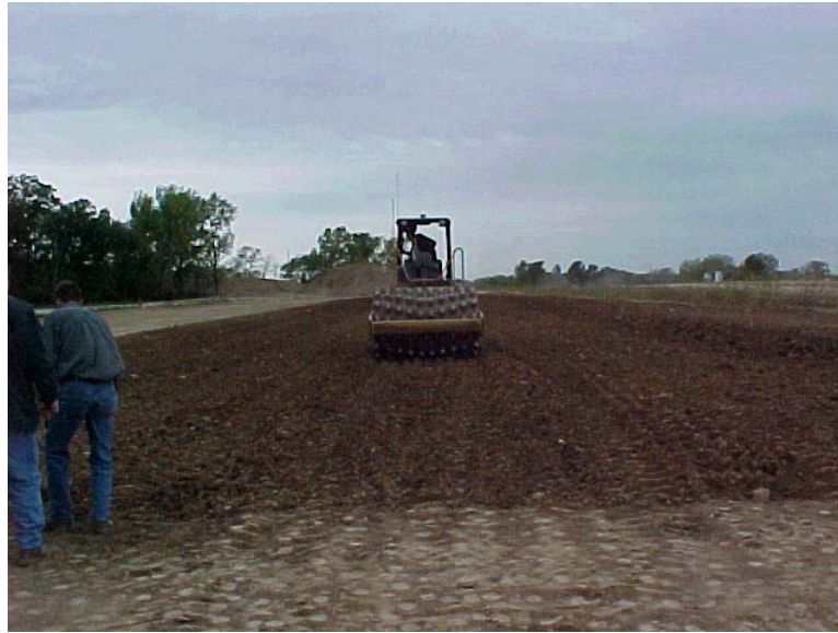
Figure 68: Compaction being performed by CAT CP533E roller in reverse for test strip 2A
