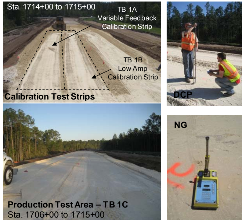
Figure 82: Field conditions and in-situ testing from Florida I-10 project
