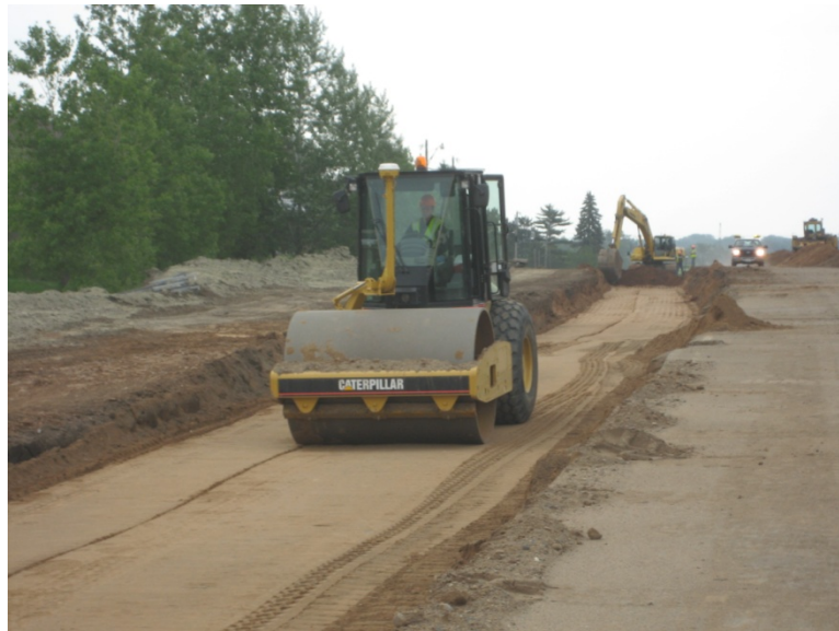
Figure 74: Field compaction using CS-563 roller
