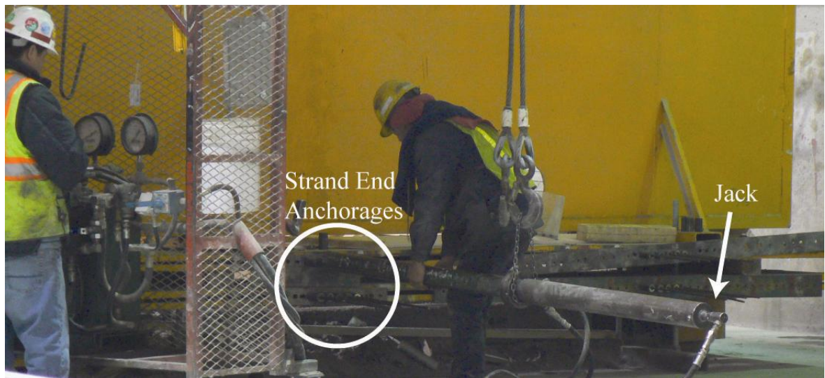
Figure 4.12. Stressing of prestressing strands for UHPC pile P1
