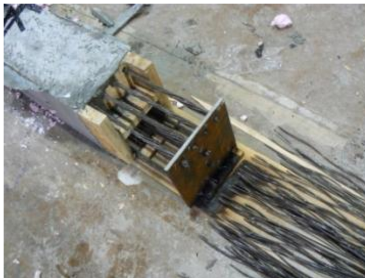
Figure 4.15. Strands released at end of UHPC pile P2
