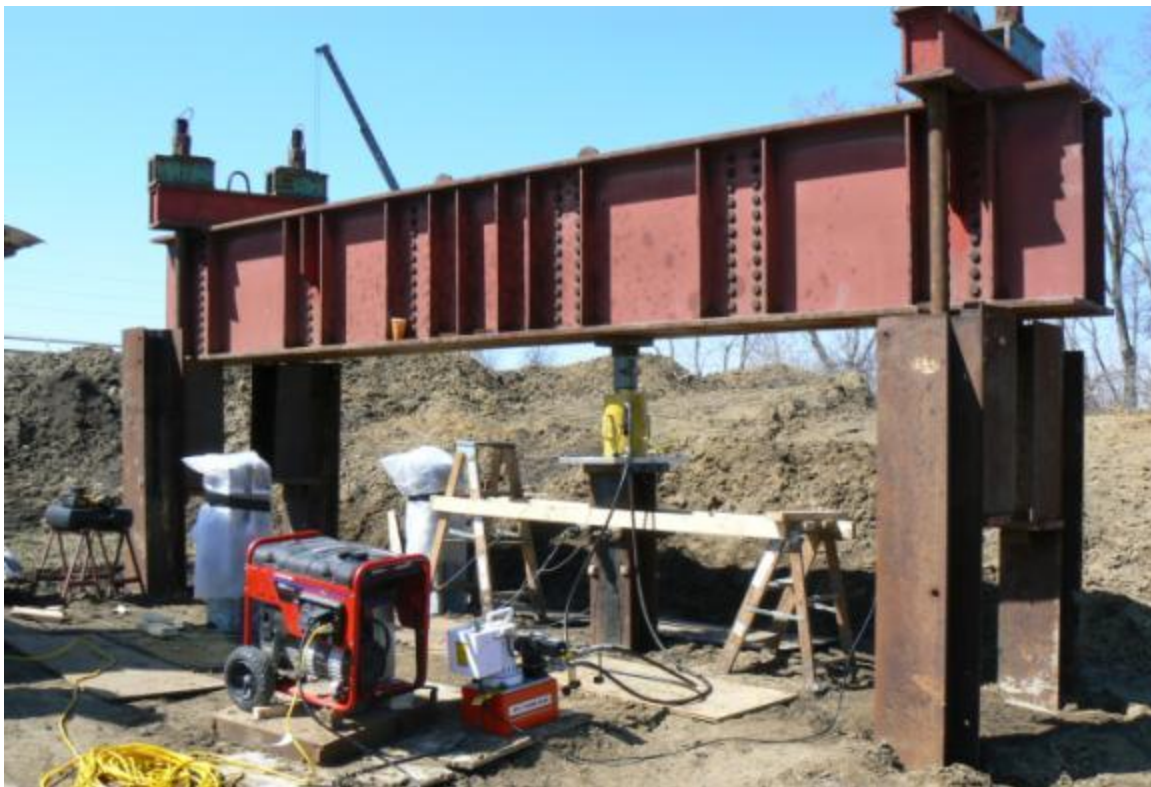
Figure 5.18. Completed vertical load test frame at the Oskaloosa test site
