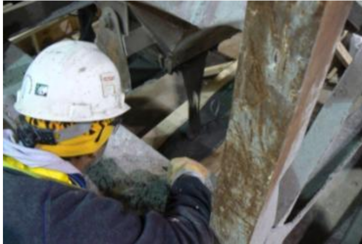
Figure 4.18. Beginning of first pour of UHPC units
