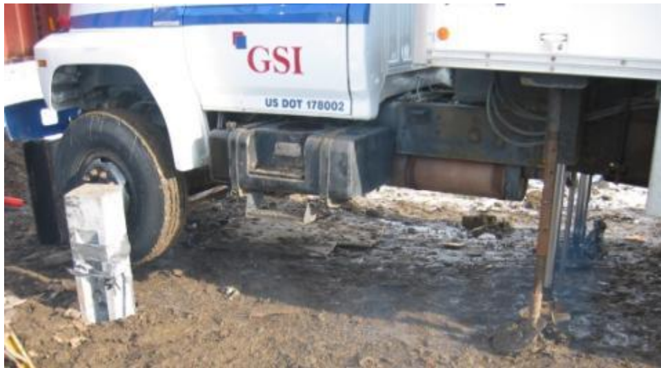
Figure 5.2. View of CPT2 test in progress, located 9 ft (2.7 m) south of UHPC pile P2
