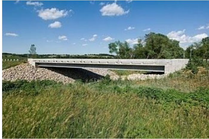
Figure 2.41. A view of completed Mars Hill Bridge (Bridge Engineering Center 2007)
